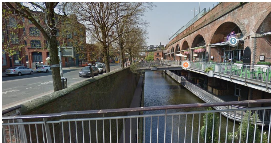
PHOTO 1 VIEW ON DEANSGATE LOCKS APPROXIMATELY 3M BELOW STREET LEVEL
