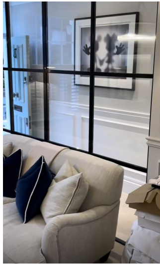
crittall glazing into front snug / lounge
