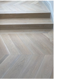
timber chevron flooring or reclaimed planks
