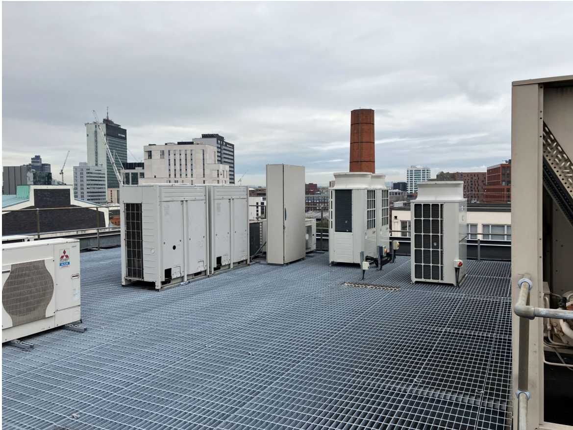
Reference 2: Existing roof plant to be matched
