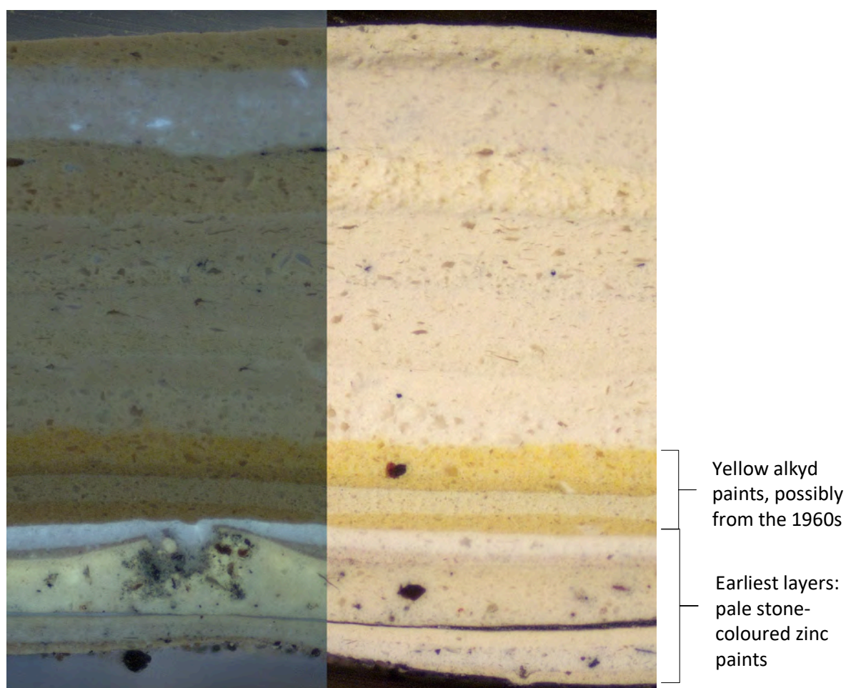
Figure 16: Sample 4 , façade stucco (left is under UV light)
