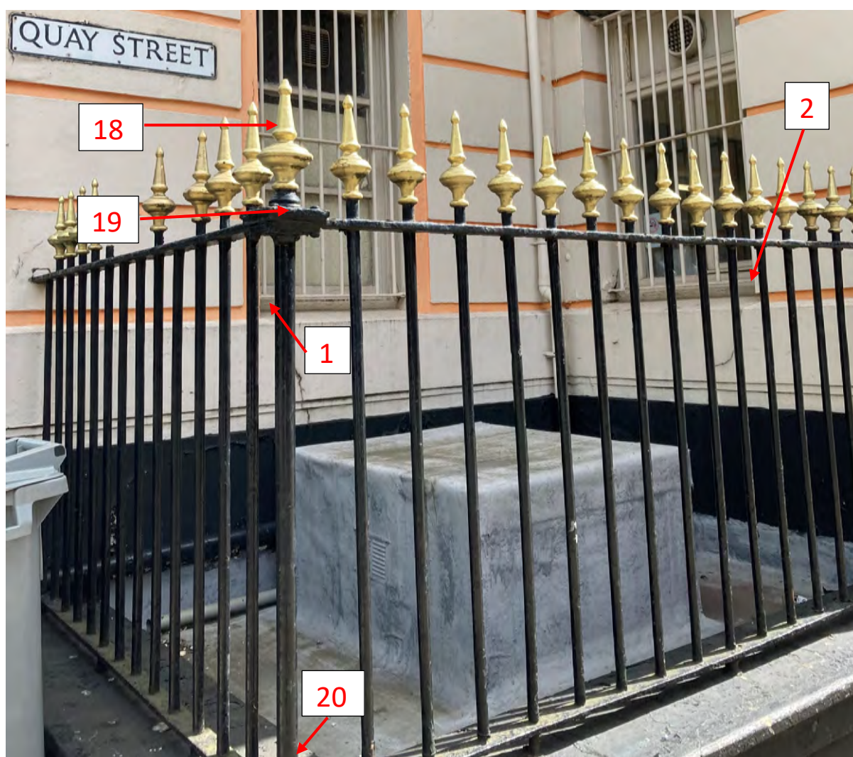
Figure 5: sample locations 1, 2 (windows W2-F and W3-F) & 18 – 20 (railings)
