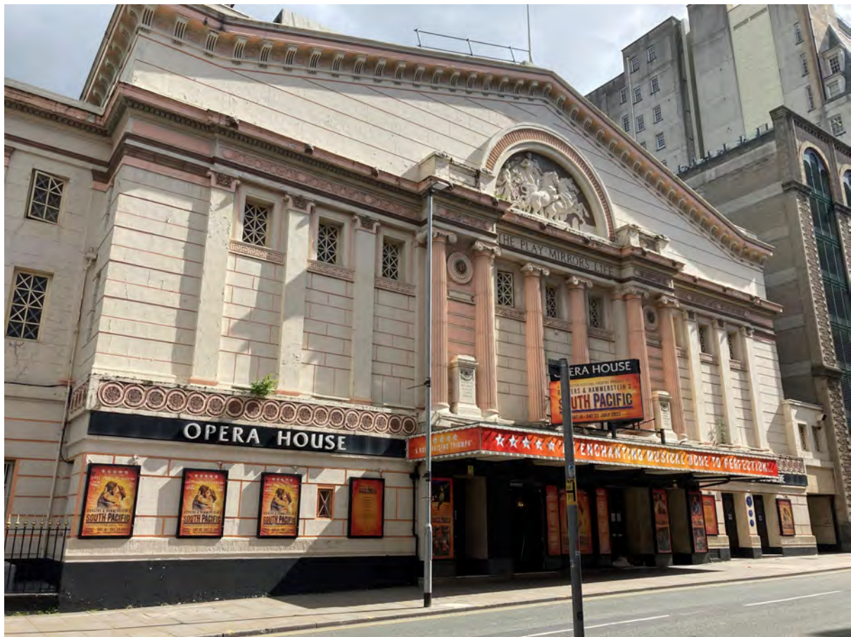
Figure 1: The Opera House façade facing the road
