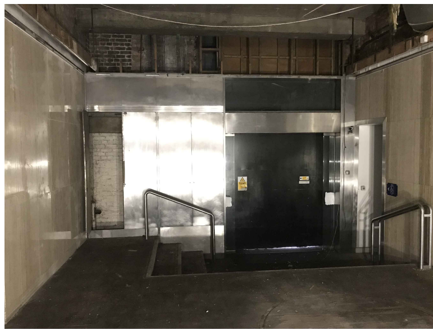
10 EXISTING ENTRANCE LOBBY 500 NTS INTERNAL PHOTO
