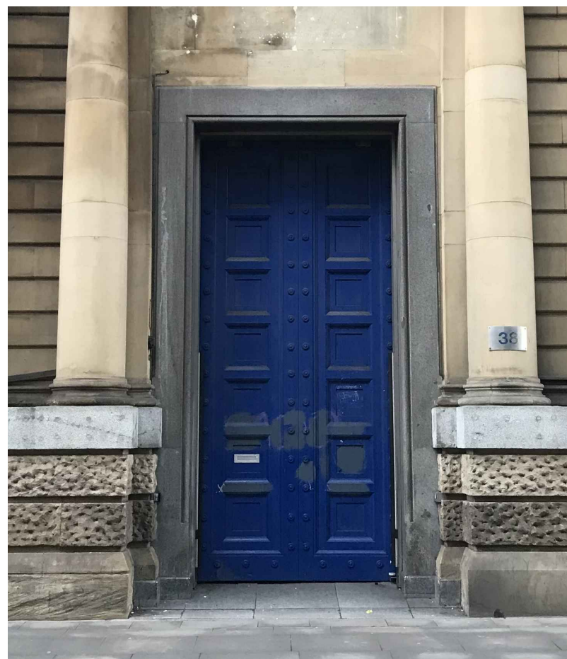
04 EXISTING MAIN DOOR 500 NTS EXTERNAL PHOTO
