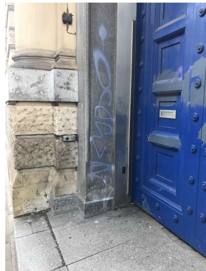
03 EXISTING MAIN DOOR 500 NTS EXTERNAL PHOTO
