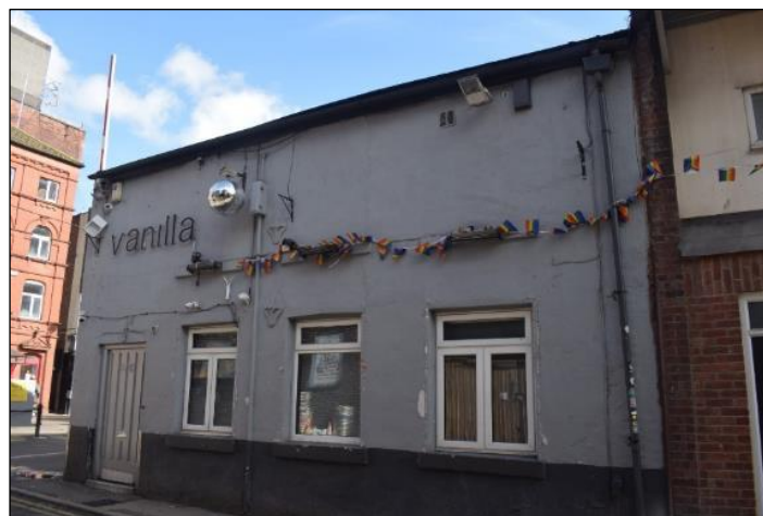
Photo 2: 39 - 41 Richmond Street, front elevation
