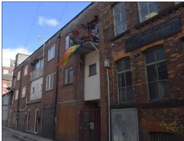
Photo 11: Modern infill, adjacent south of site
