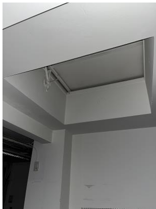
Concrete upstands/reveals to roof lights
