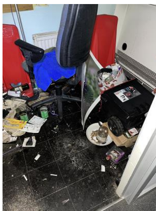
Vinyl tiles visible in small store
