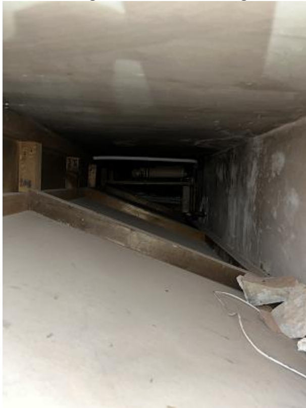
Interior of angled timber duct/boxing
