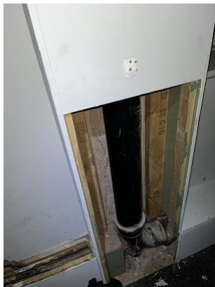
Boxing to soil pipe
