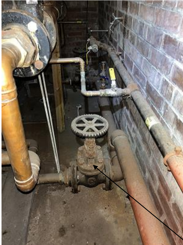
Sample LR05 Asbestos thermal
