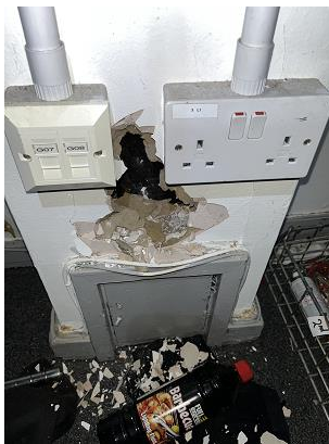
Plasterboard boxing to cast pipe
