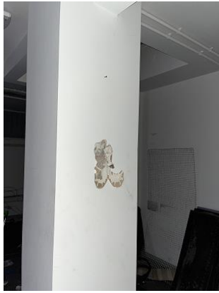
Plasterboard dry-lining to central pillar
