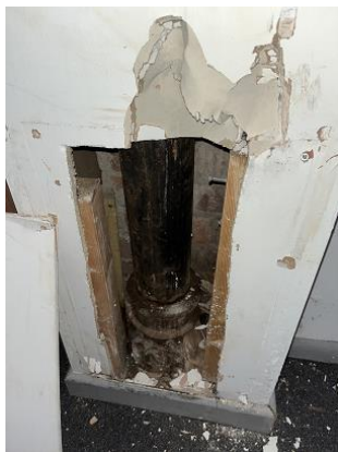
Plastered boxing to cast downpipe
