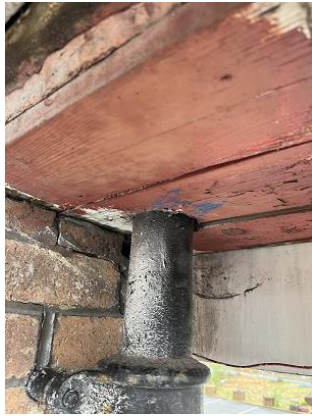
Timber boarded soffit to eaves
