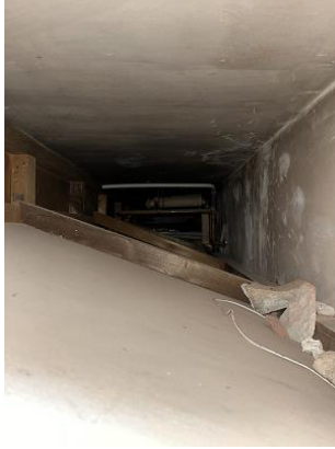
Timber boxing to high level
