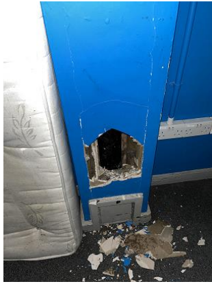
Plasterboard boxing to cast downpipe
