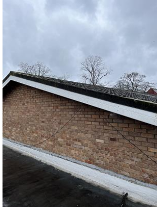
Plastic renovation fascia over timber bargeboards
