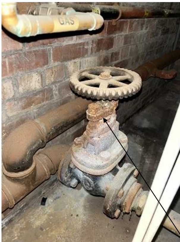
Sample LR05 Asbestos thermal
