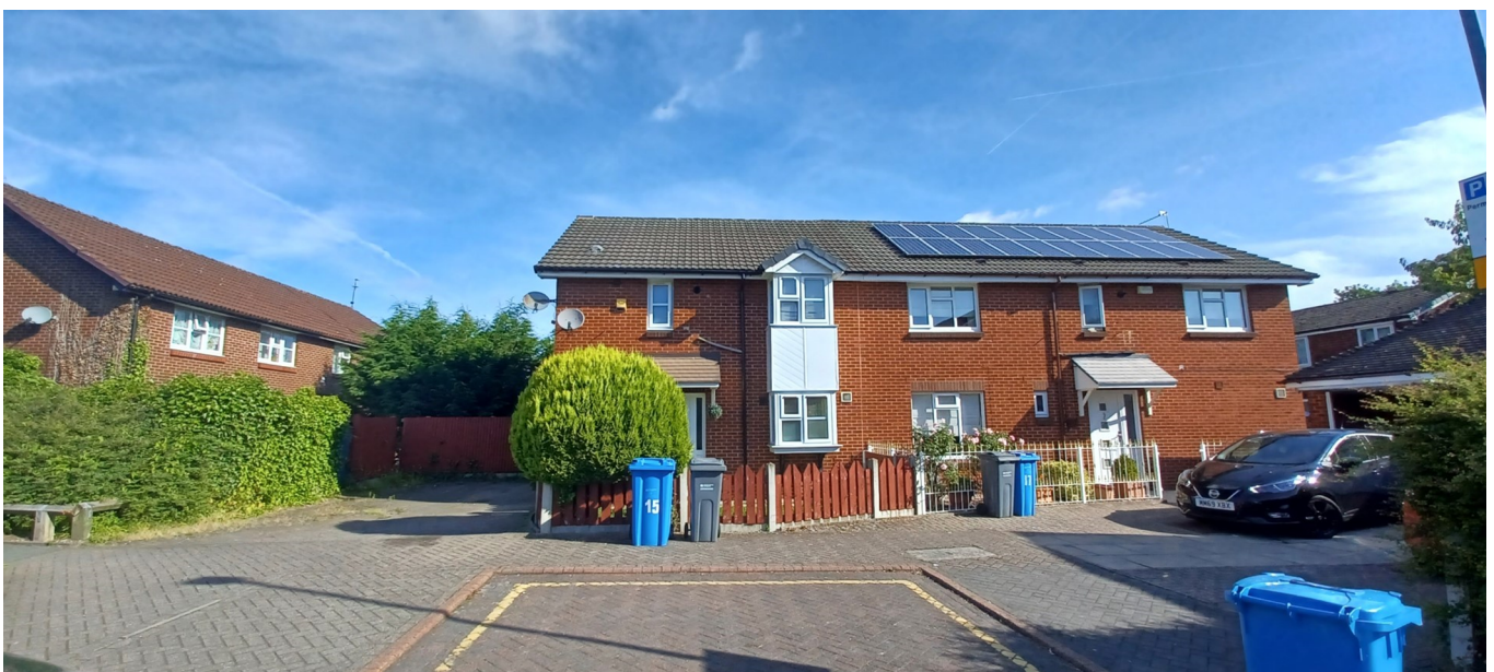
Figure 1. Principal elevation of property.
