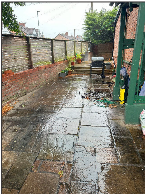
Picture 3. The root protection area of T2# is already hardstanding where the proposed build is to be located.
