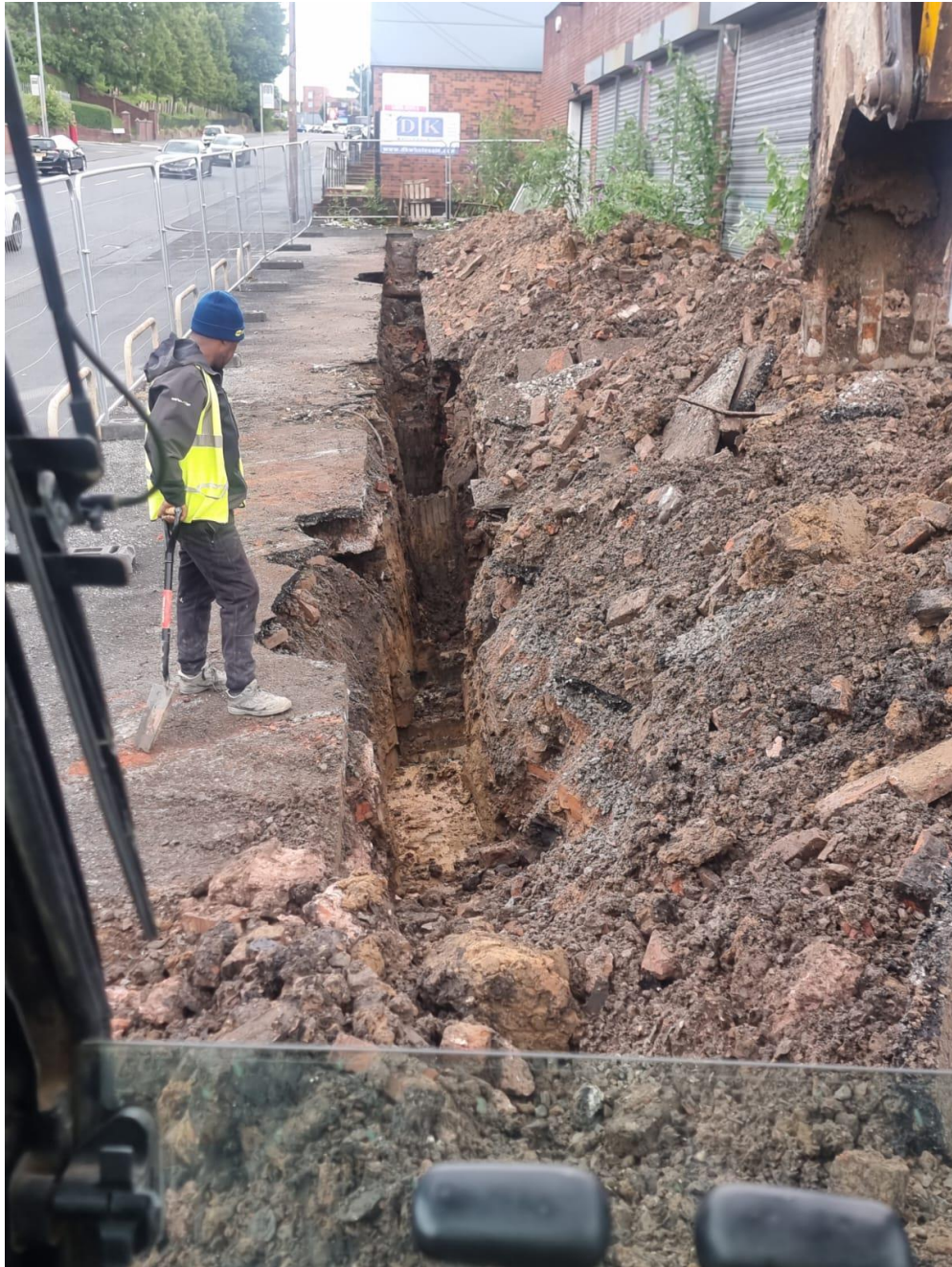
Pic 1. View from South Western end of trench
