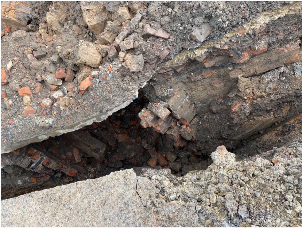
Pic 3. Evidence of former basement bay windows of Victorian terrace that used to occupy the site.
