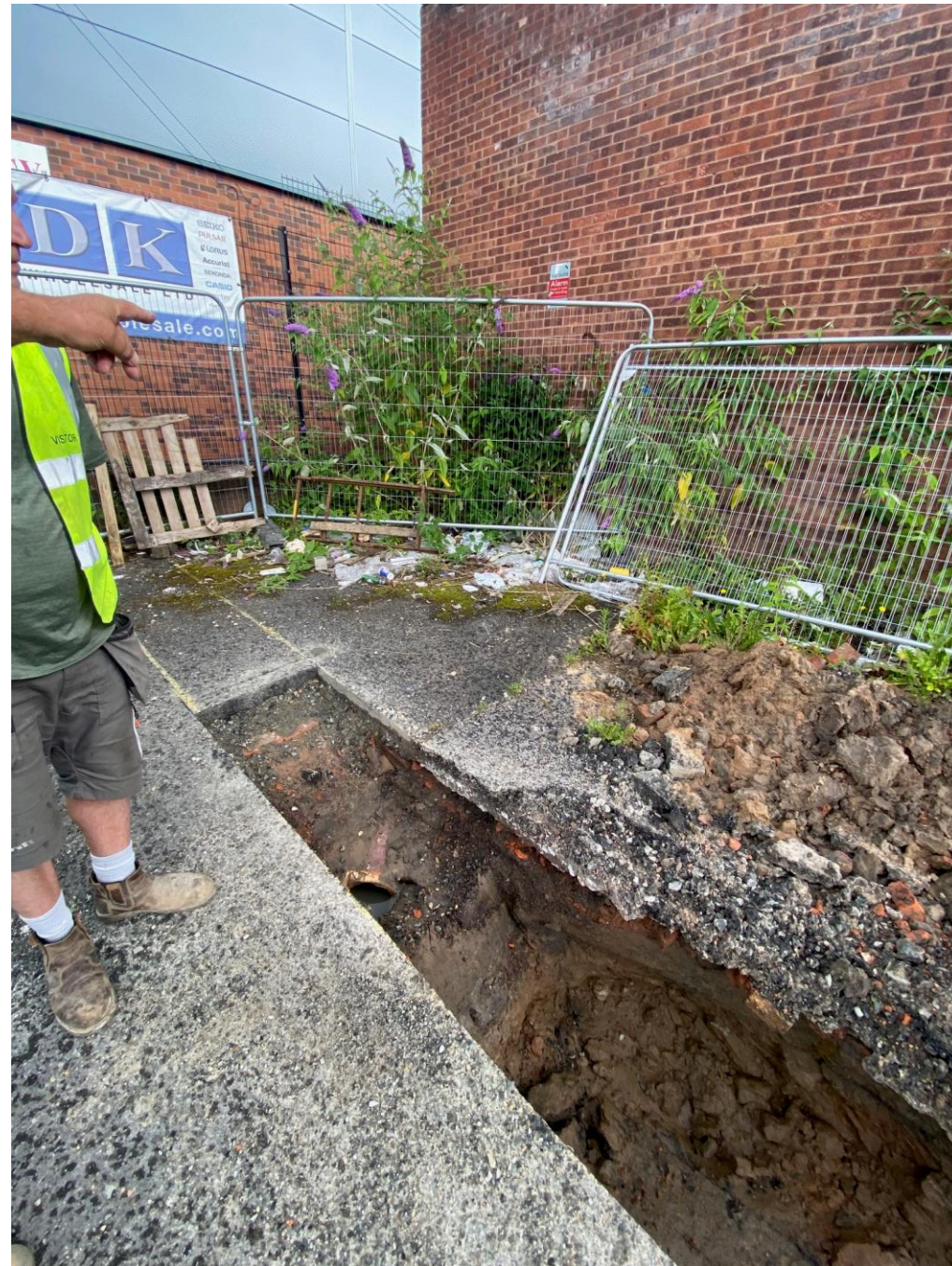
Pic 4. Similar angle to pic 2. Possible culvert just visible appears to clip corner of existing building.
