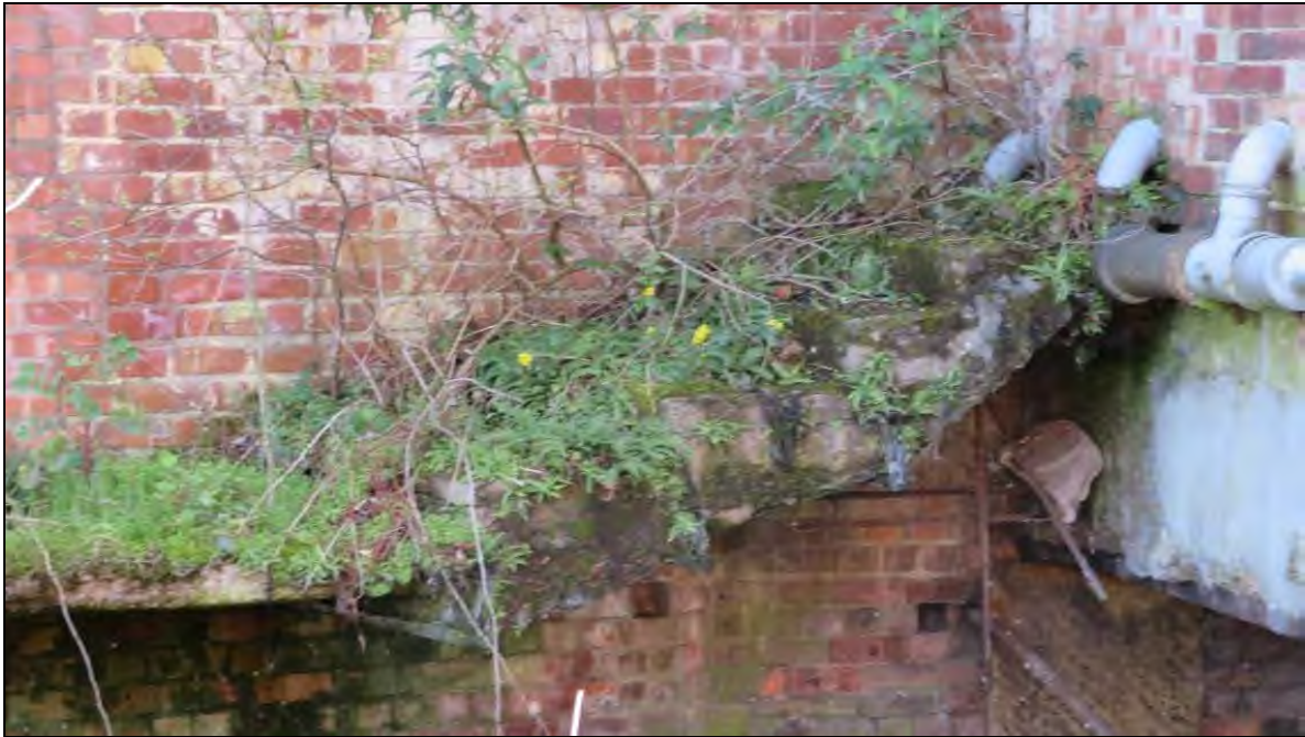
Plate 59: The remains of steps at the site of the Mayfield Printworks, 20 th March 2019
