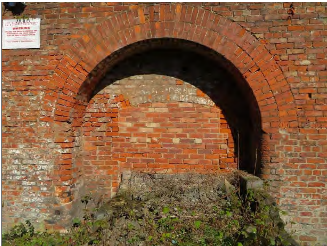
Plate 58: The blocked south-facing arched doorway of the Mayfield Printworks, 20 th March 2019
