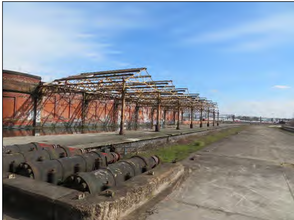
Plate 39: Platforms and part of the roof skeleton at Mayfield Railway Station
