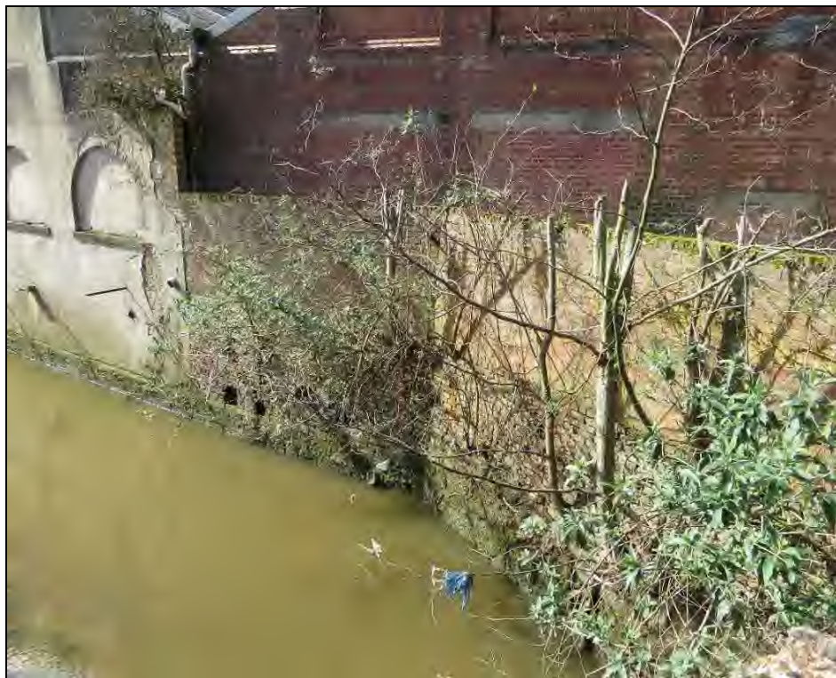
Plate 35: Stone and brick-built river retaining walls associated with the Mayfield Printworks survive within Block 2 and Block 5
