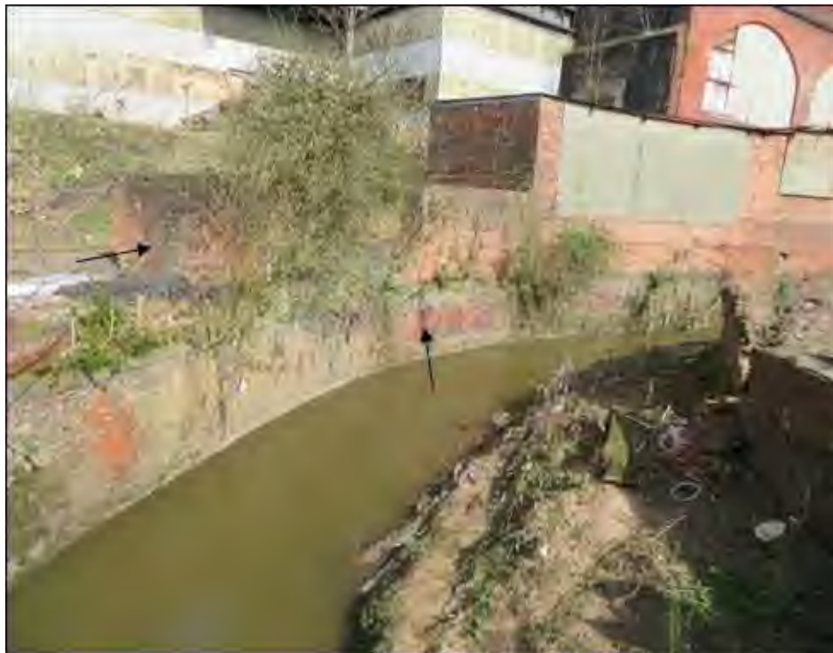
Plate 36: Stone and brick-built river retaining walls associated with the Mayfield Printworks
