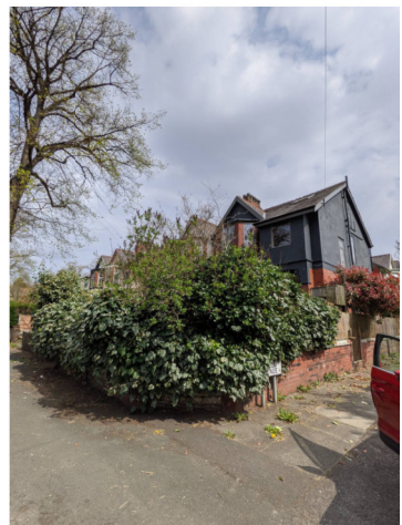
House conditions at the time of purchasing
