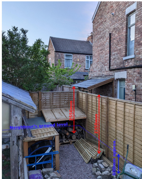
Neighbouring fences and ground level versus N.109 Dudley Rd fence
