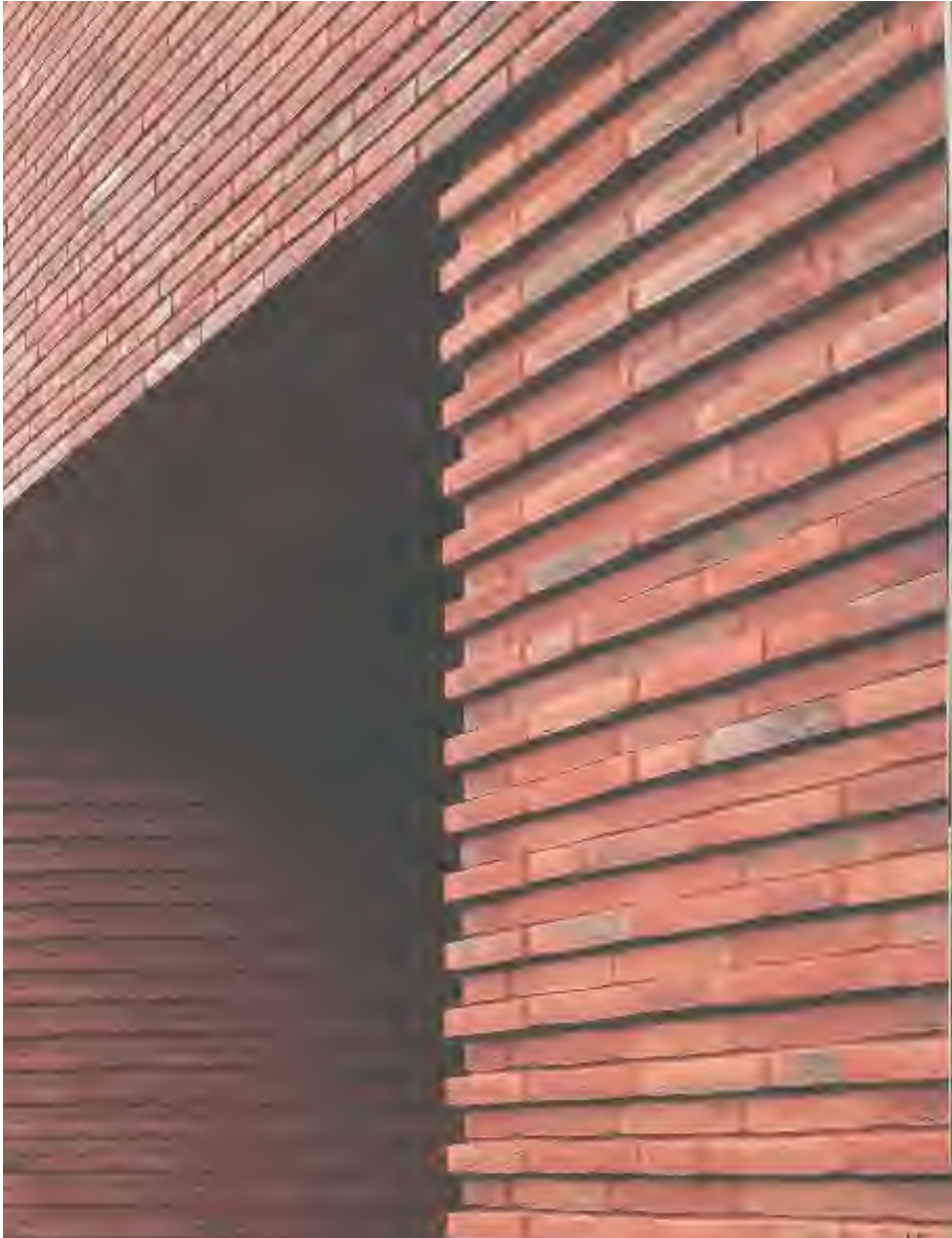
Rusticated brick piers with projecting bricks
