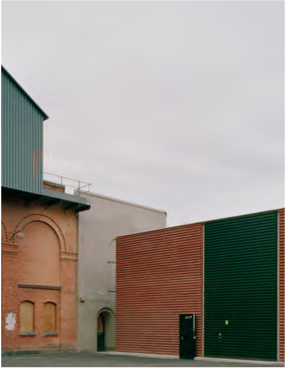
Image showing composition of bricks and green louvres
