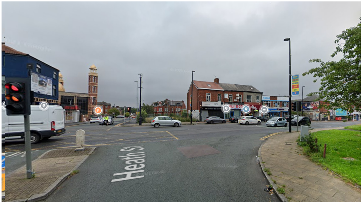
View of site from Heath Street,
