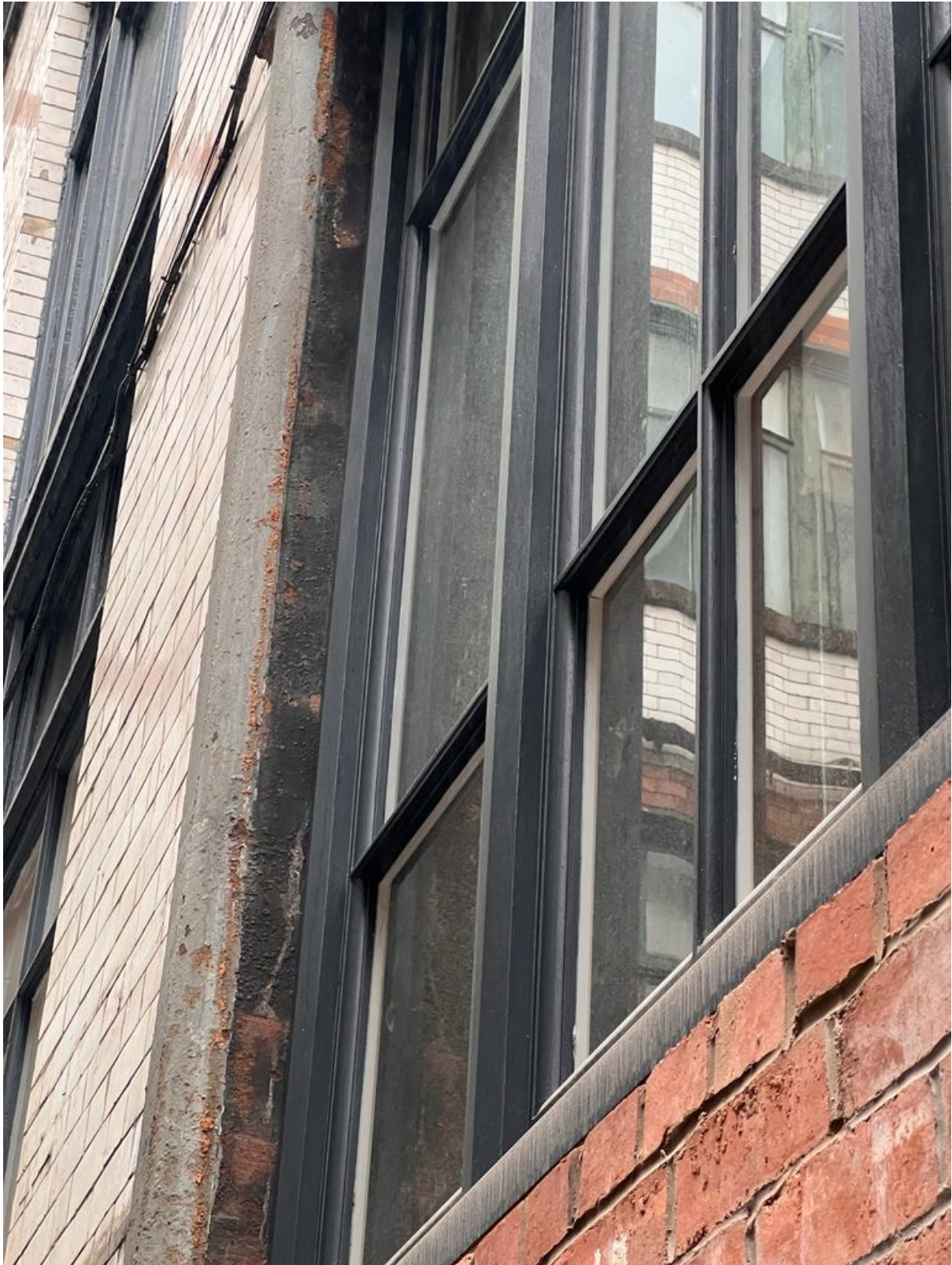
Figure 38: WP.0.09 Internal (Credit CubicWorks 2023)
