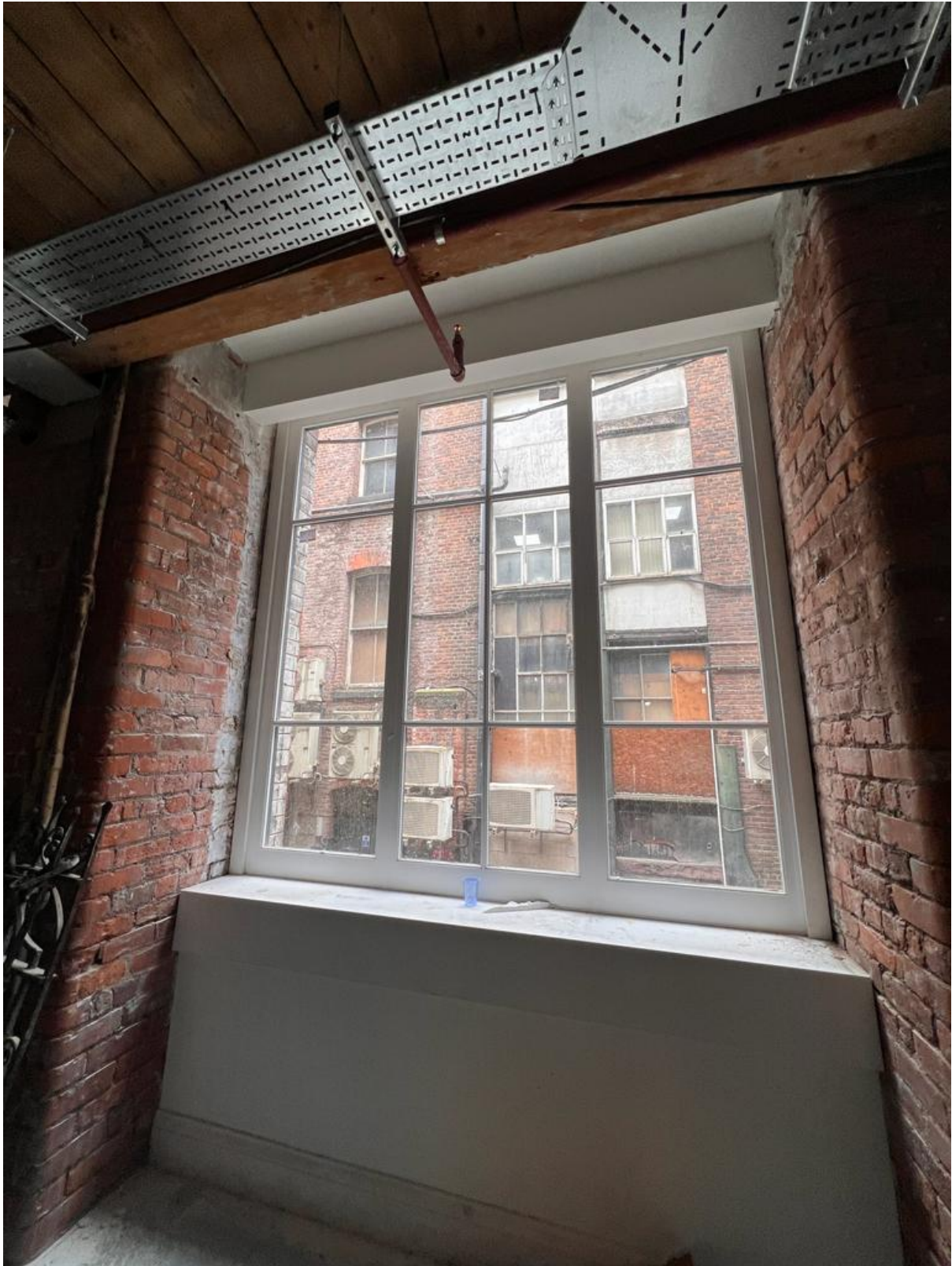
Figure 66: WP.0.14 Internal (Credit CubicWorks 2023)
