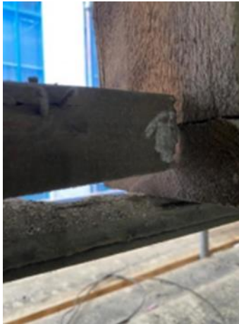
Figure 19: WP.0.08 External, Credit Fairhurst 2022
