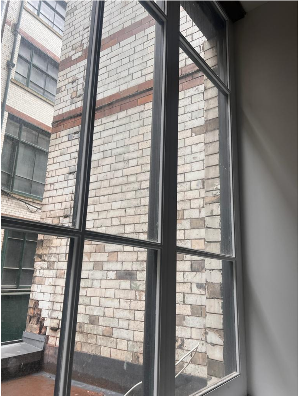
Figure 54: WP.0.13 Internal (Credit CubicWorks 2023)
