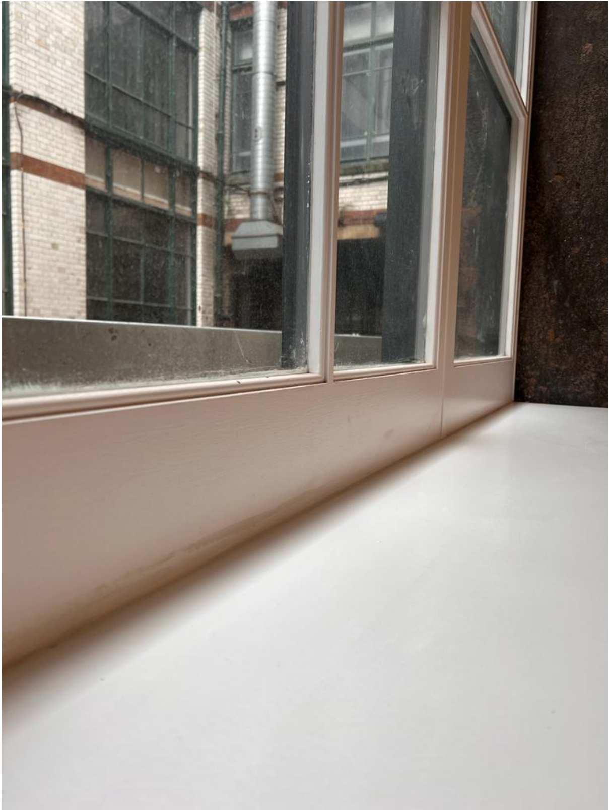
Figure 36: WP.0.09 Internal (Credit CubicWorks 2023)
