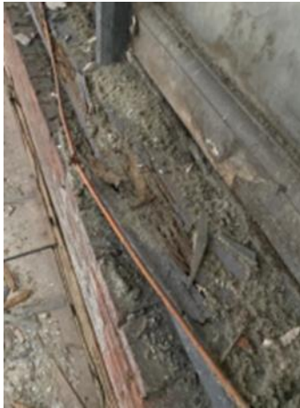
Figure 17: WP.0.08 External (Credit Fairhurst 2022)
