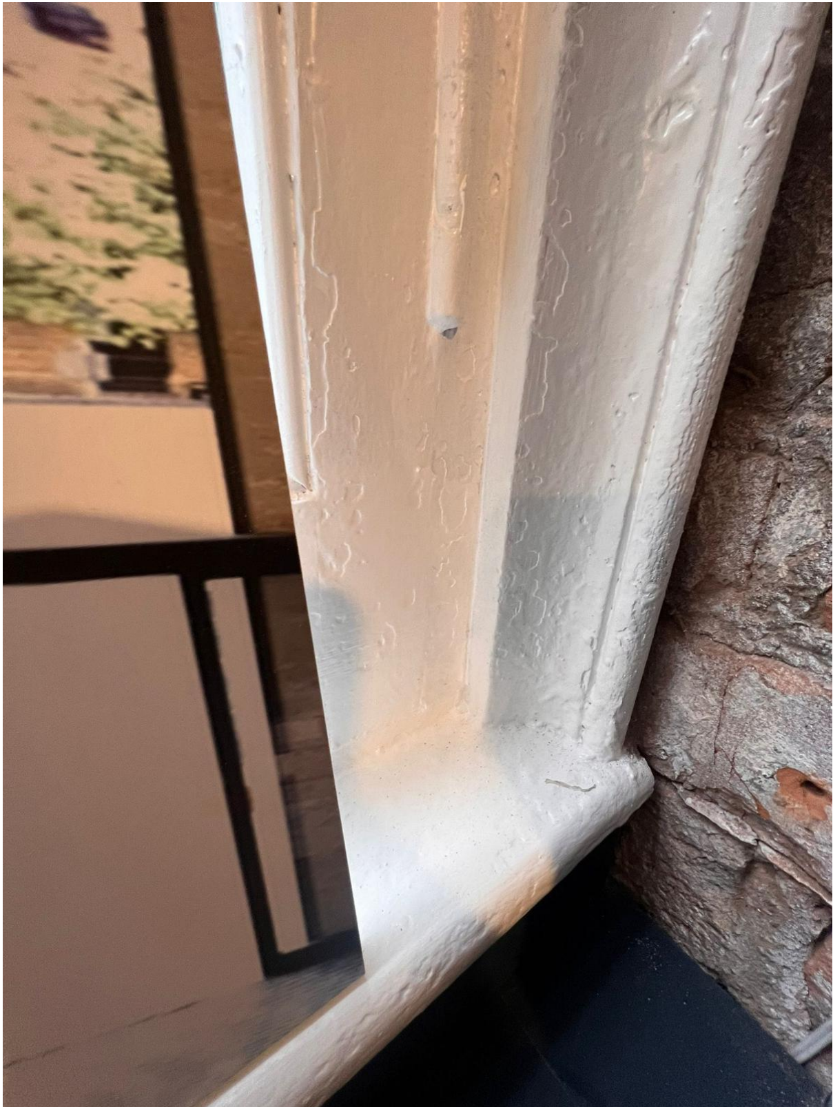
Figure 24: WP.0.08 Internal (Credit CubicWorks 2023)
