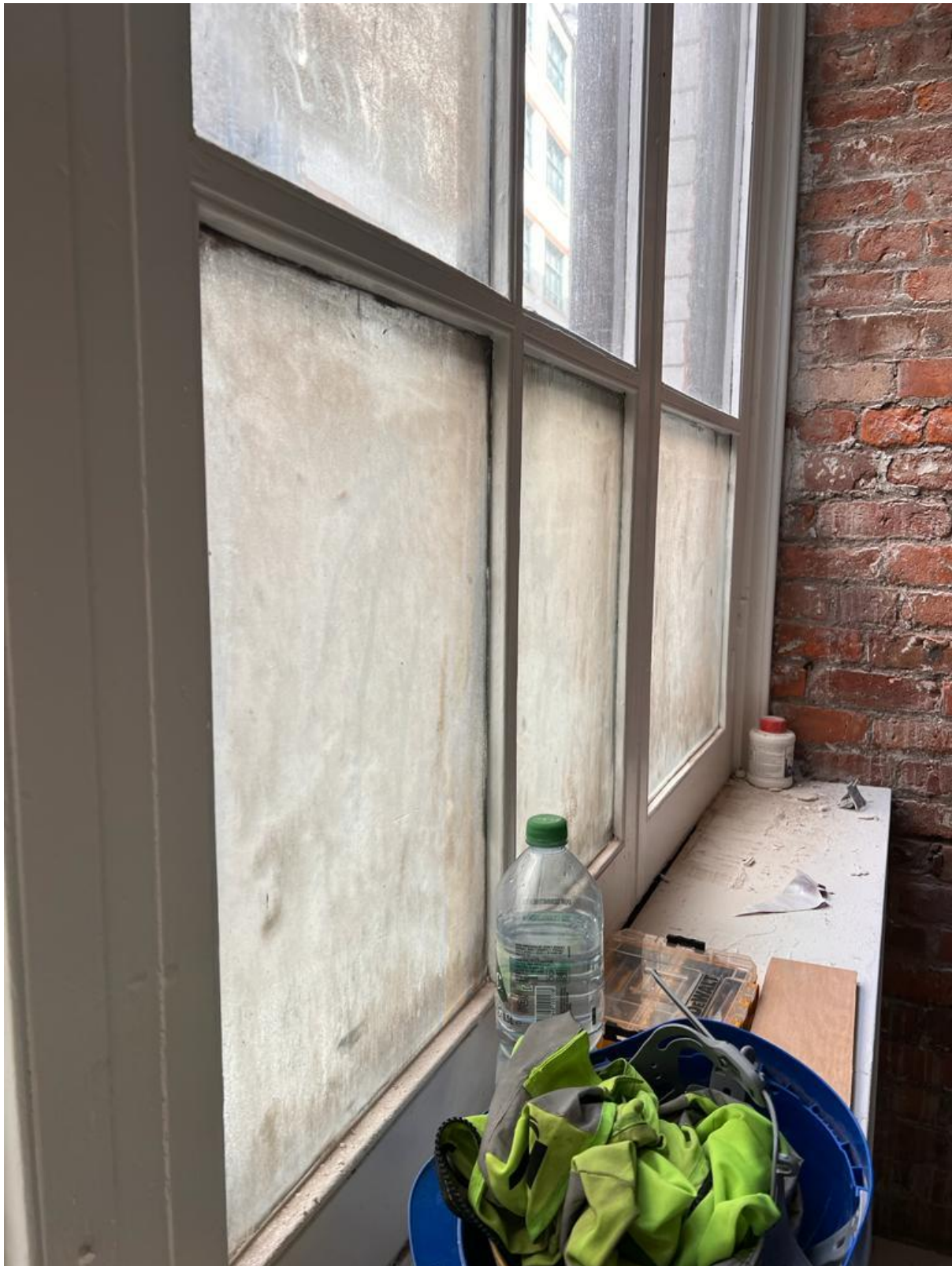
Figure 74: WP.0.15 Internal (Credit CubicWorks 2023)
