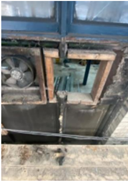
Figure 16: WP.0.08 External (Credit Fairhurst 2022)
