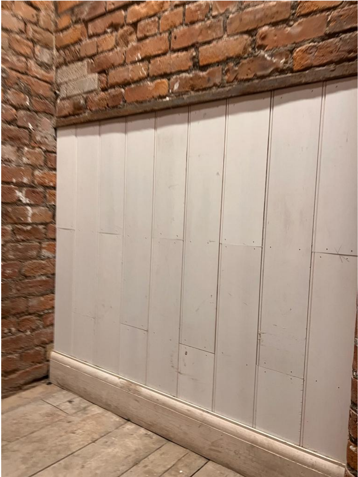
Figure 41: WP.0.10 Internal (Credit CubicWorks 2023)
