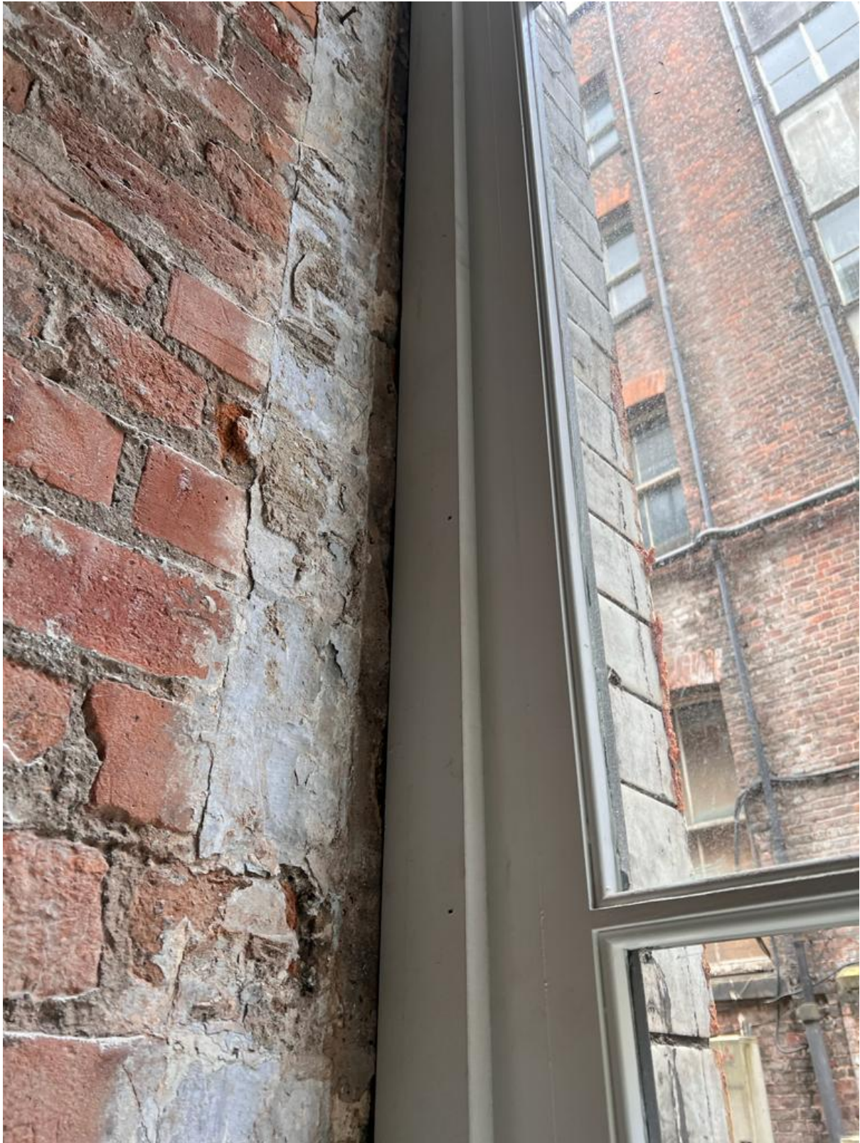
Figure 68: WP.0.14 Internal (Credit CubicWorks 2023)
