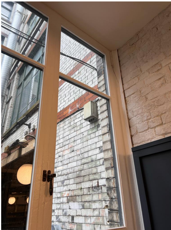
Figure 11: WP.0.07 Internal (Credit CubicWorks 2023)
