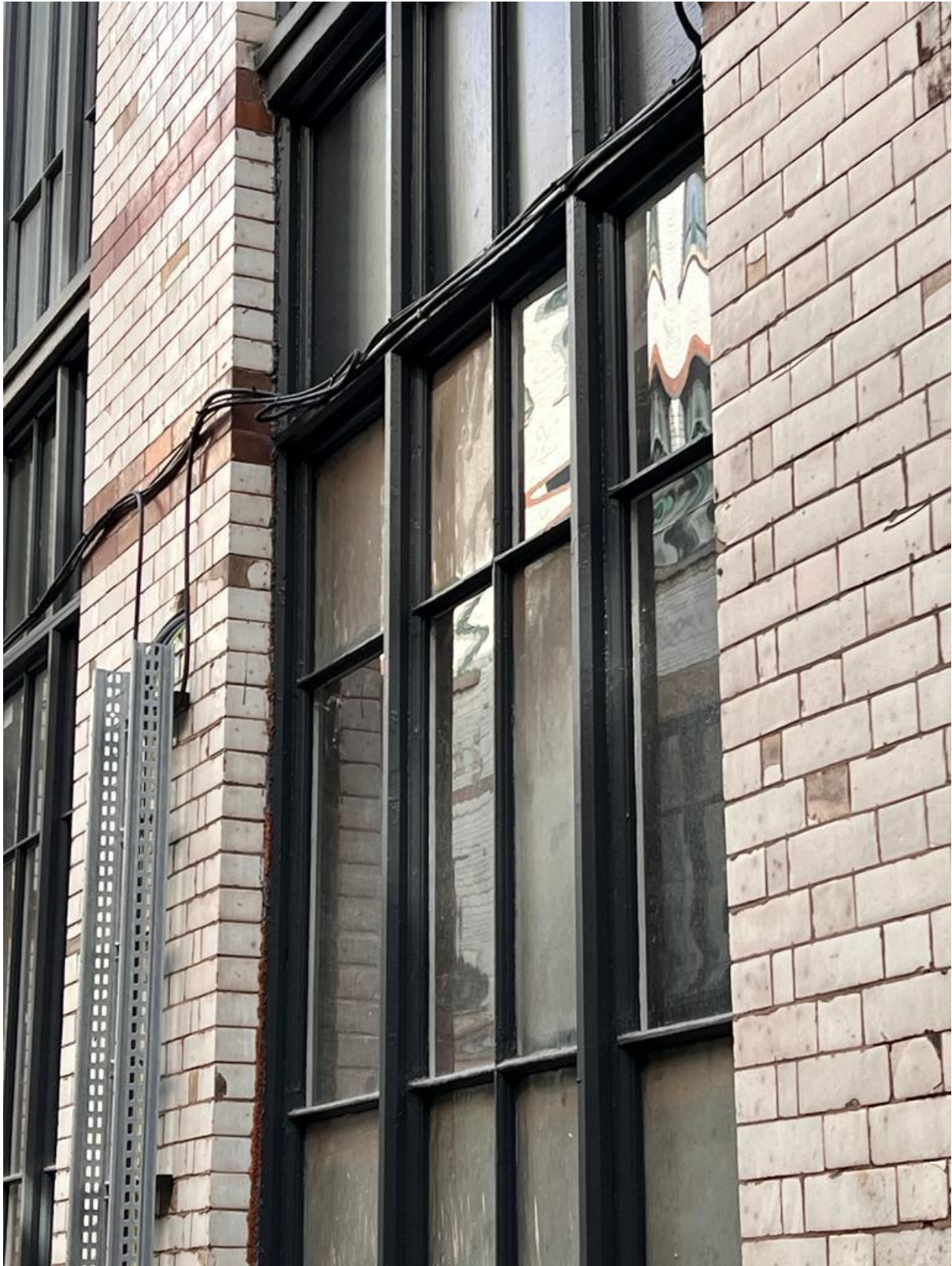
Figure 76: WP.0.15 Internal (Credit CubicWorks 2023)
