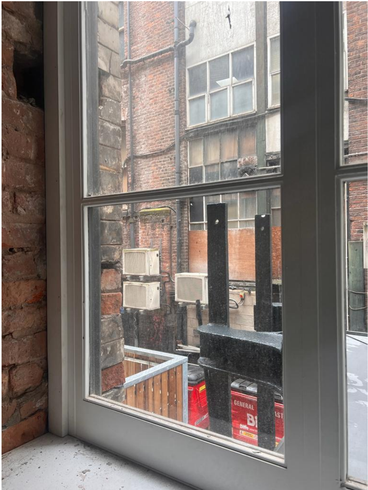
Figure 53: WP.0.13 Internal (Credit CubicWorks 2023)
