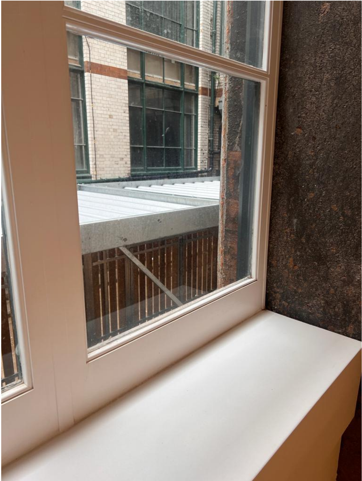
Figure 35: WP.0.09 Internal (Credit CubicWorks 2023)
