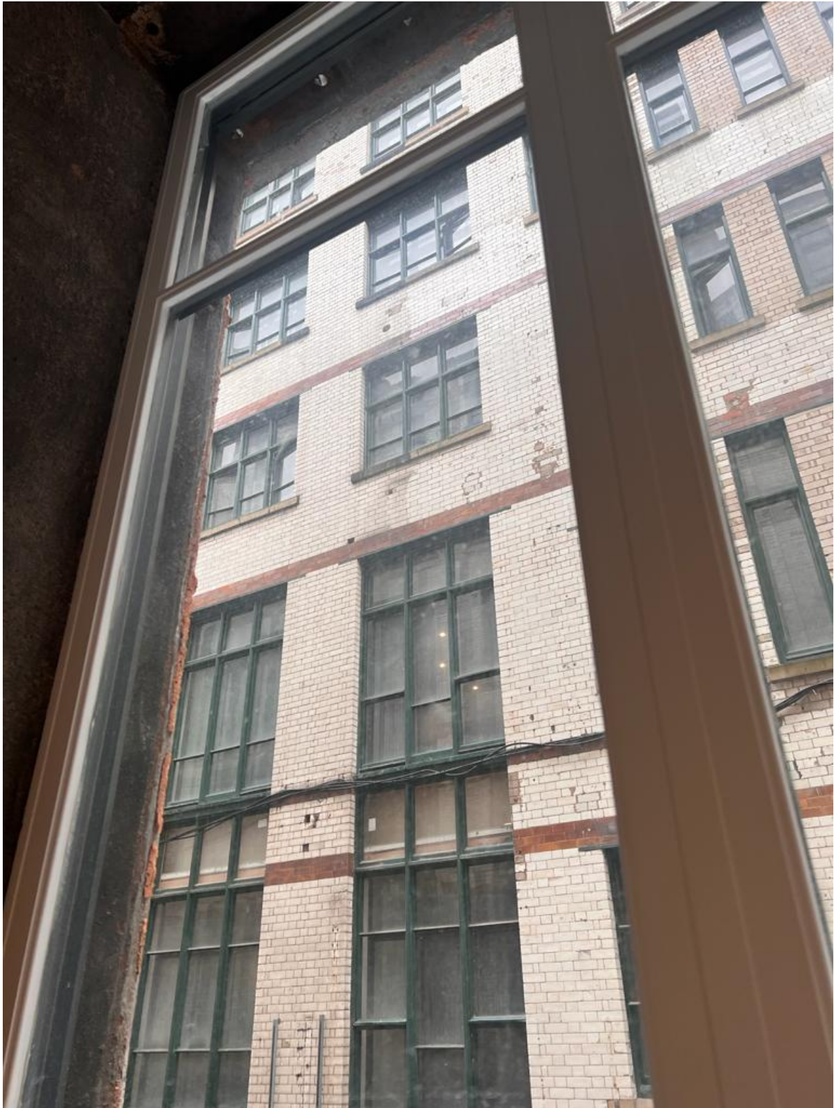
Figure 35: WP.0.09 Internal (Credit CubicWorks 2023)
