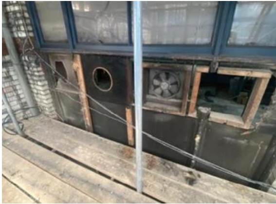
Figure 15: WP.0.08 External (Credit Fairhurst 2022)
