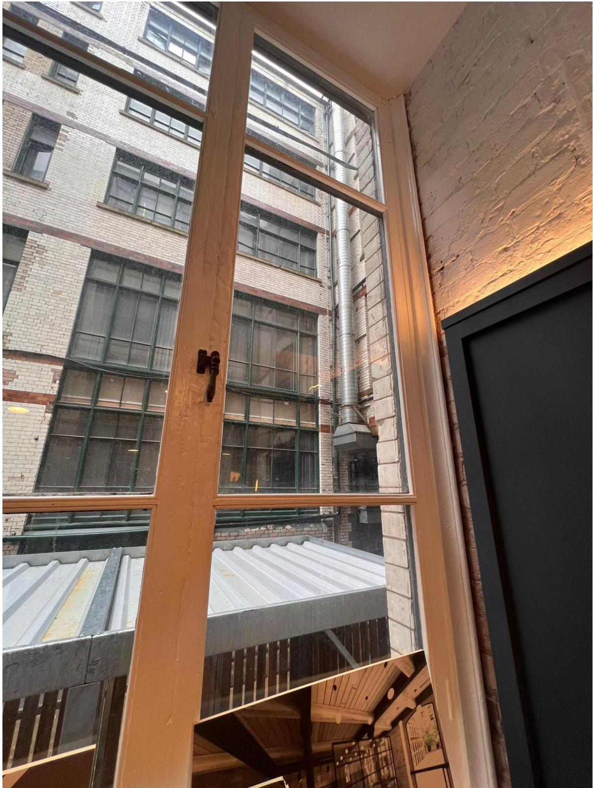
Figure 23: WP.0.08 Internal (Credit CubicWorks 2023)
