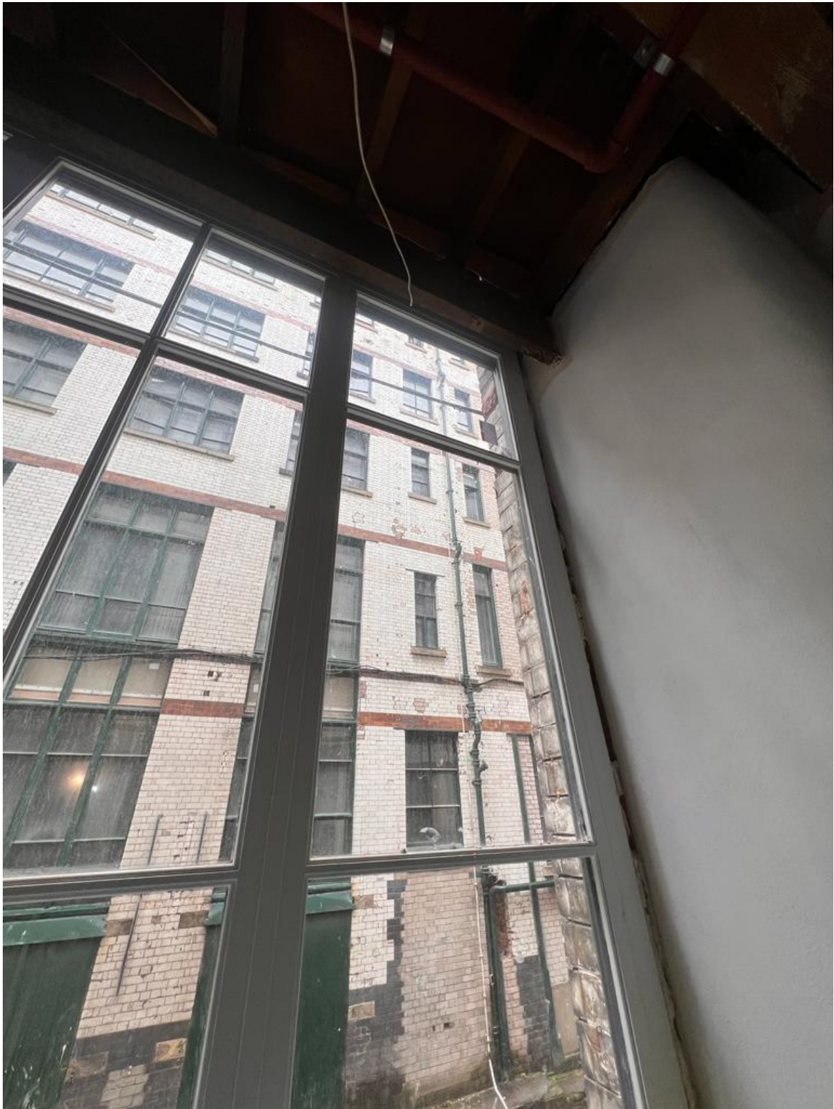
Figure 45: WP.0.11 Internal (Credit CubicWorks 2023)
