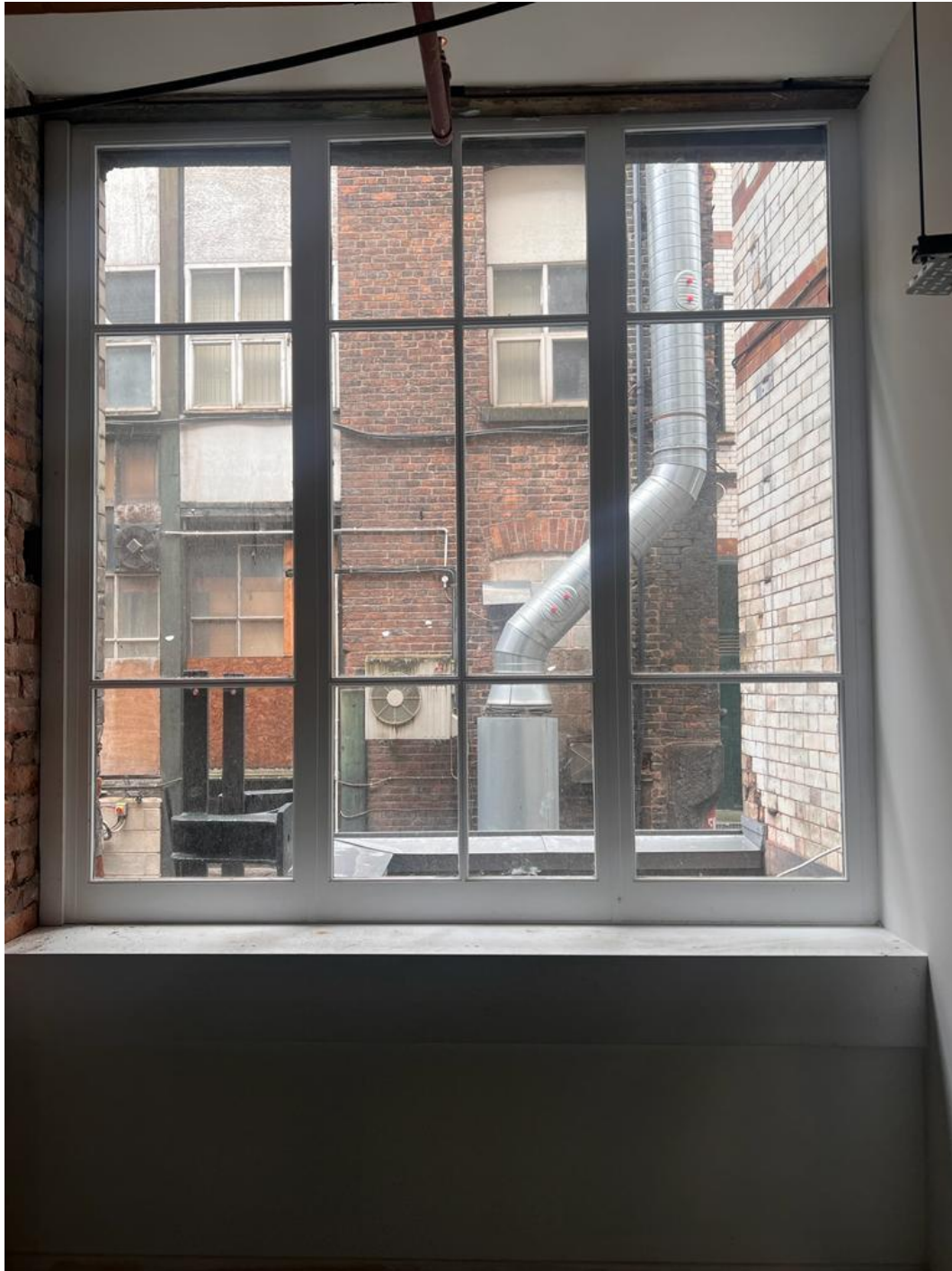
Figure 52: WP.0.13 Internal (Credit CubicWorks 2023)
