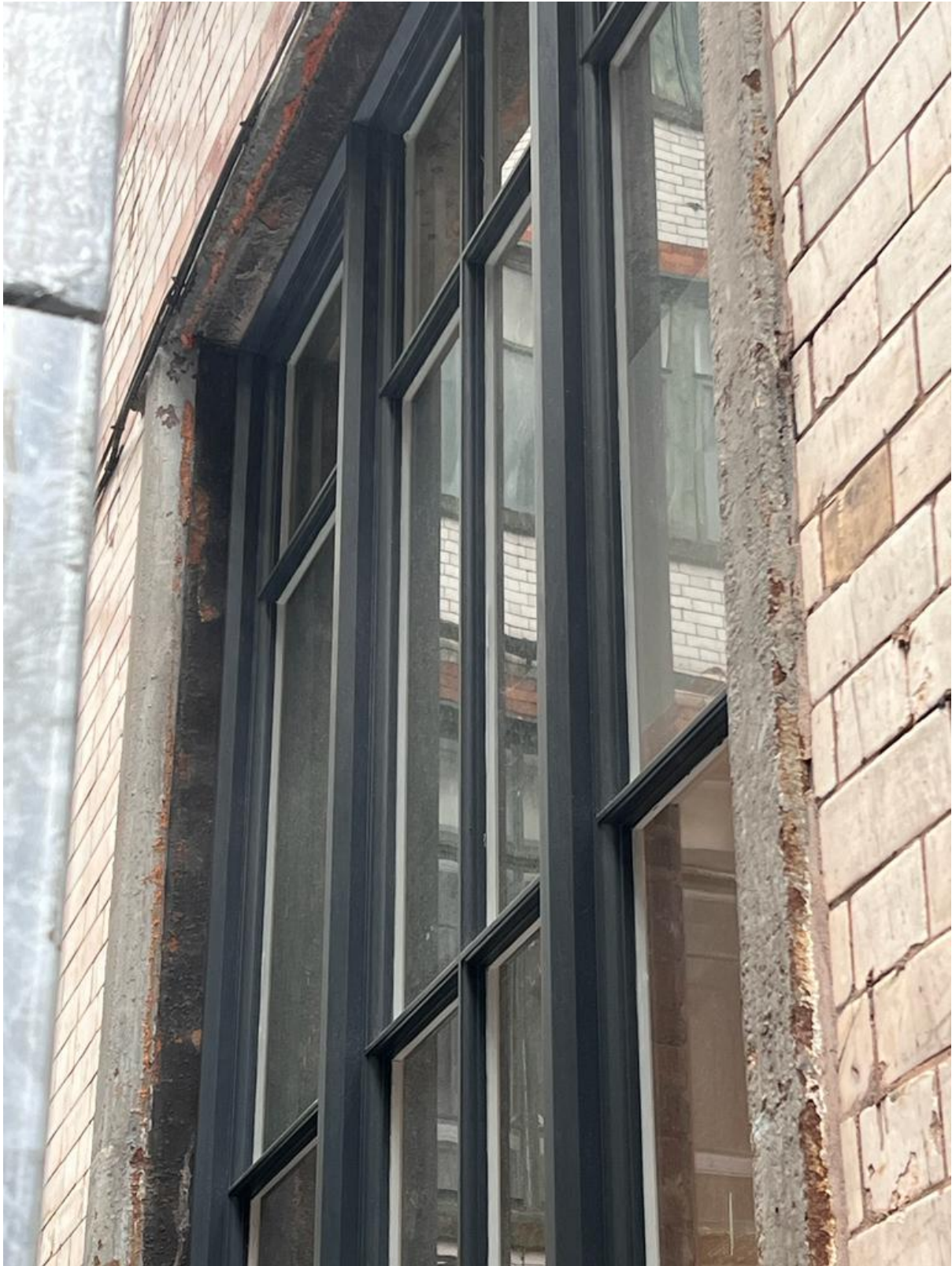
Figure 37: WP.0.09 Internal (Credit CubicWorks 2023)
