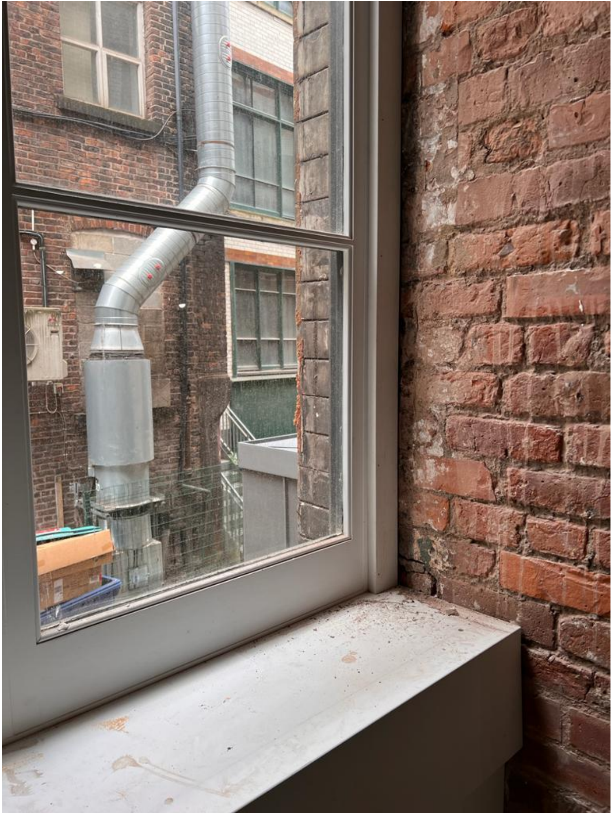
Figure 67: WP.0.14 Internal (Credit CubicWorks 2023)
