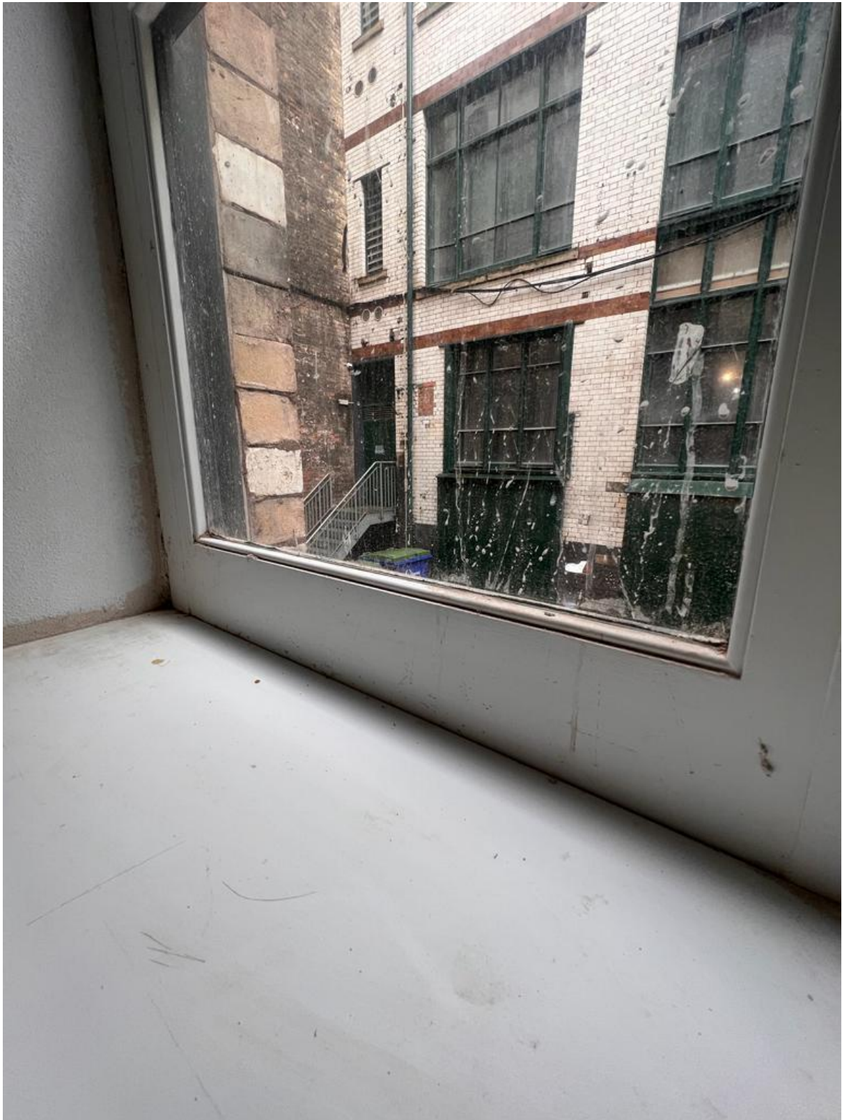
Figure 46: WP.0.11 Internal (Credit CubicWorks 2023)
