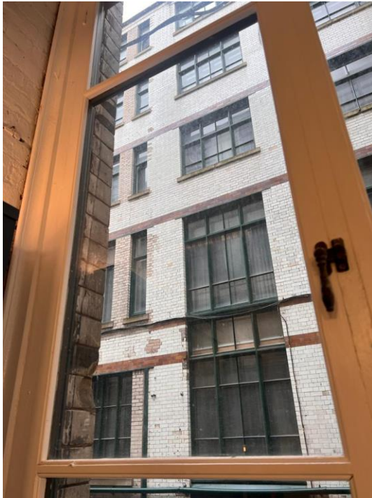
Figure 10: WP.0.07 Internal (Credit CubicWorks 2023)
