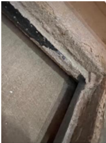
Figure 20: WP.0.08 External, Credit Fairhurst 2022
