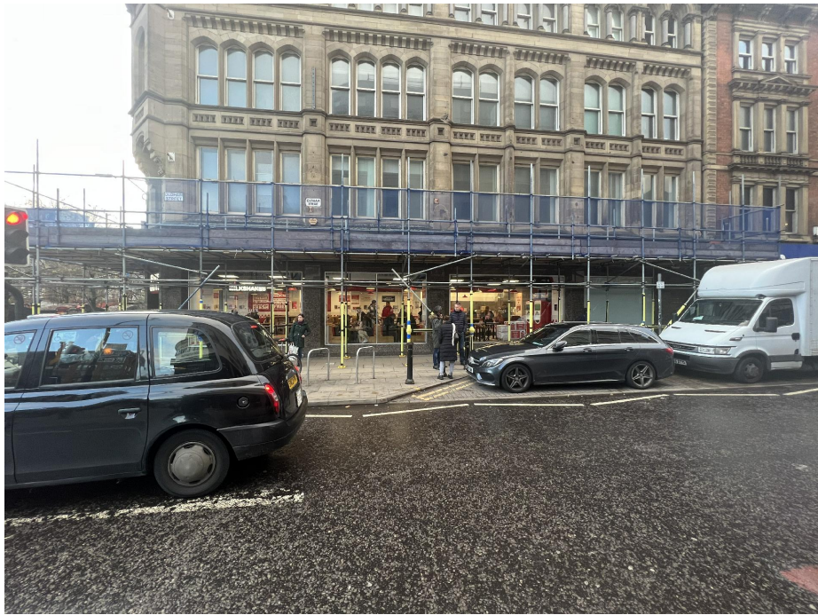
04 PHOTO OF SCAFFOLDING ON OLDHAM STREET SCALE NTS@A3
