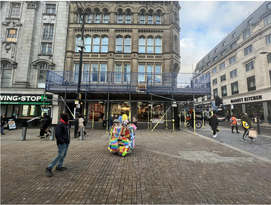
03 PHOTO OF SCAFFOLDING ON PICCADILLY SCALE NTS@A3
