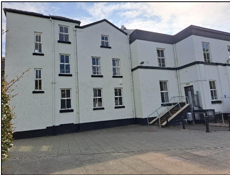
Photograph 2 showing the eastern elevation
