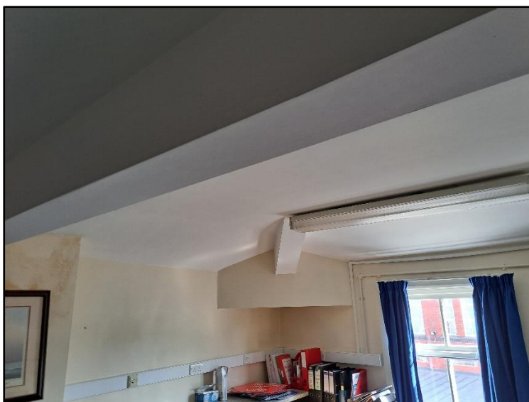
Photograph 4 showing the interior ceiling
