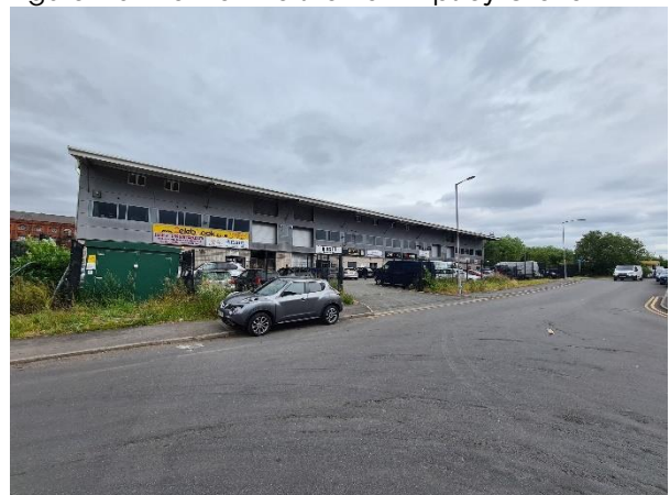
Figure 2.7: View of the adjoining commercial building to the east.
