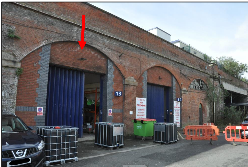
Close up image showing external view of Arch 13 (red arrow)
