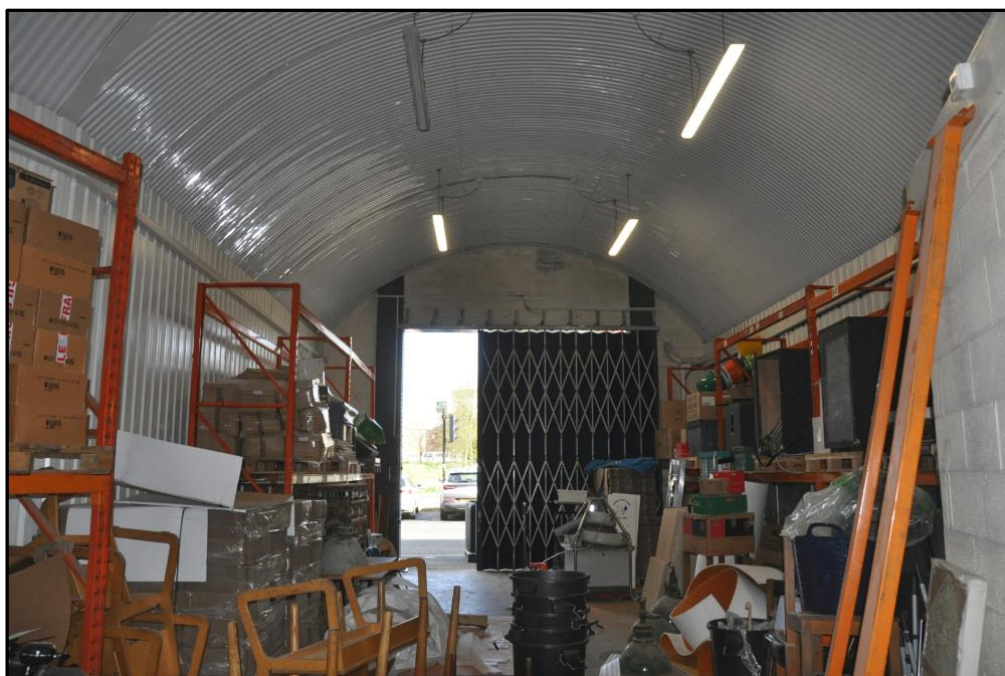
Internal view of Arch 13 looking north east
