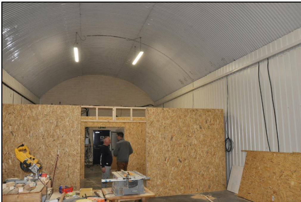
Internal view of Arch 13 looking south west
