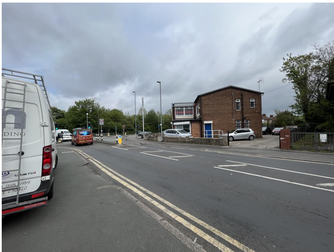
Figure 2. Photo of proposed location – from the corner of Burnside Drive
