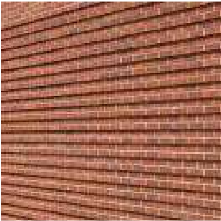
Red Brickwork Detailing
