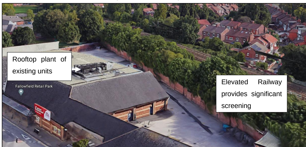
Figure 1: The existing site
