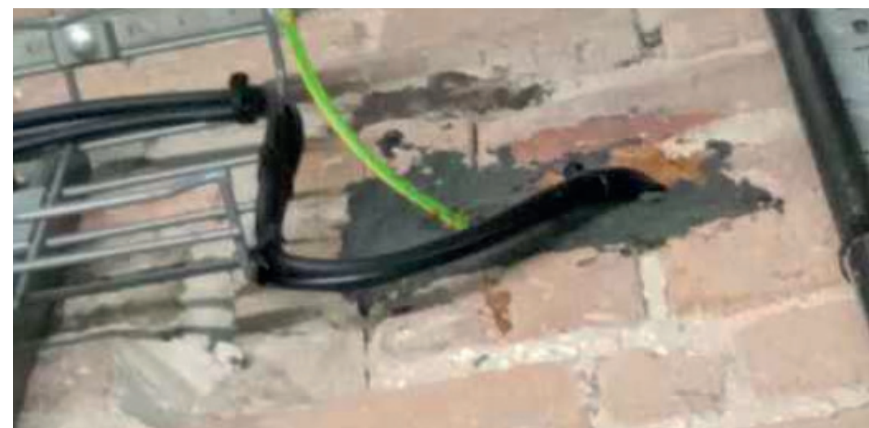
Example photo of localised cleaning of brickwork to remove mastic
