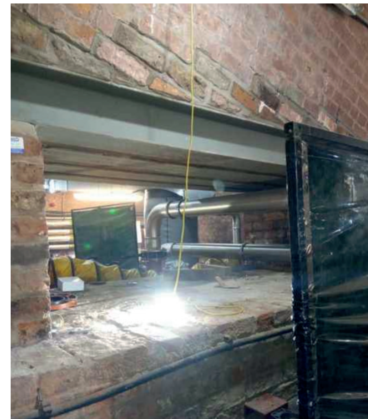
Opening between two spaces to be filled with fire rated partition
