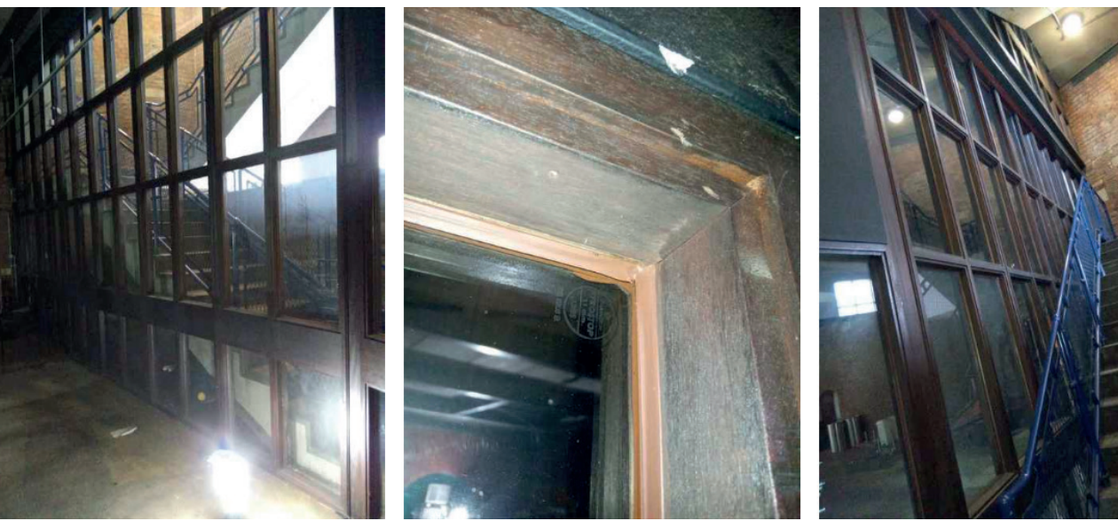
Example photo of non fire rated glazing within non historic partition
