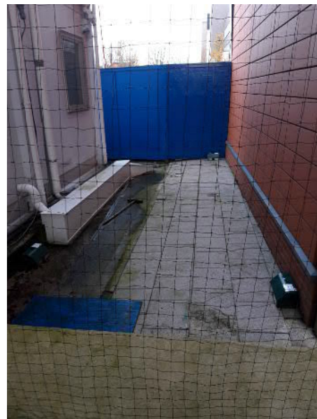
View to the west - wooden fence.
