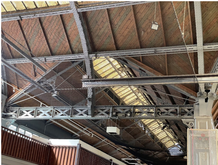
Figure 5 Duo Pitch / Arched Roof Interface
