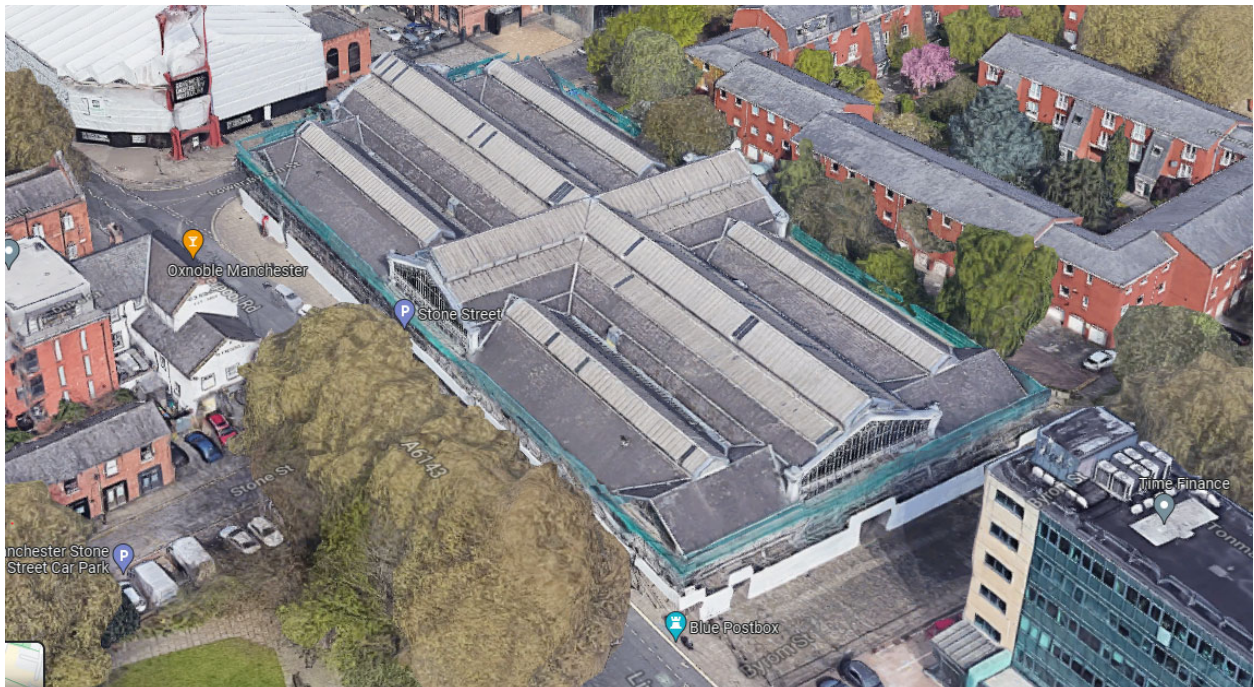
Figure 2 - Aerial View of Roof
