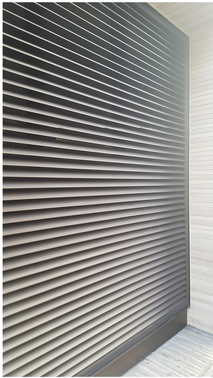
5. Inverted louvres to external plant area
