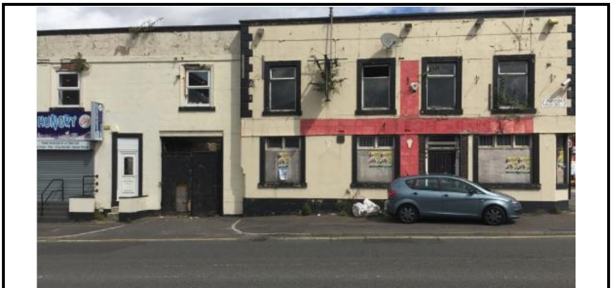
The view to site frontage.
