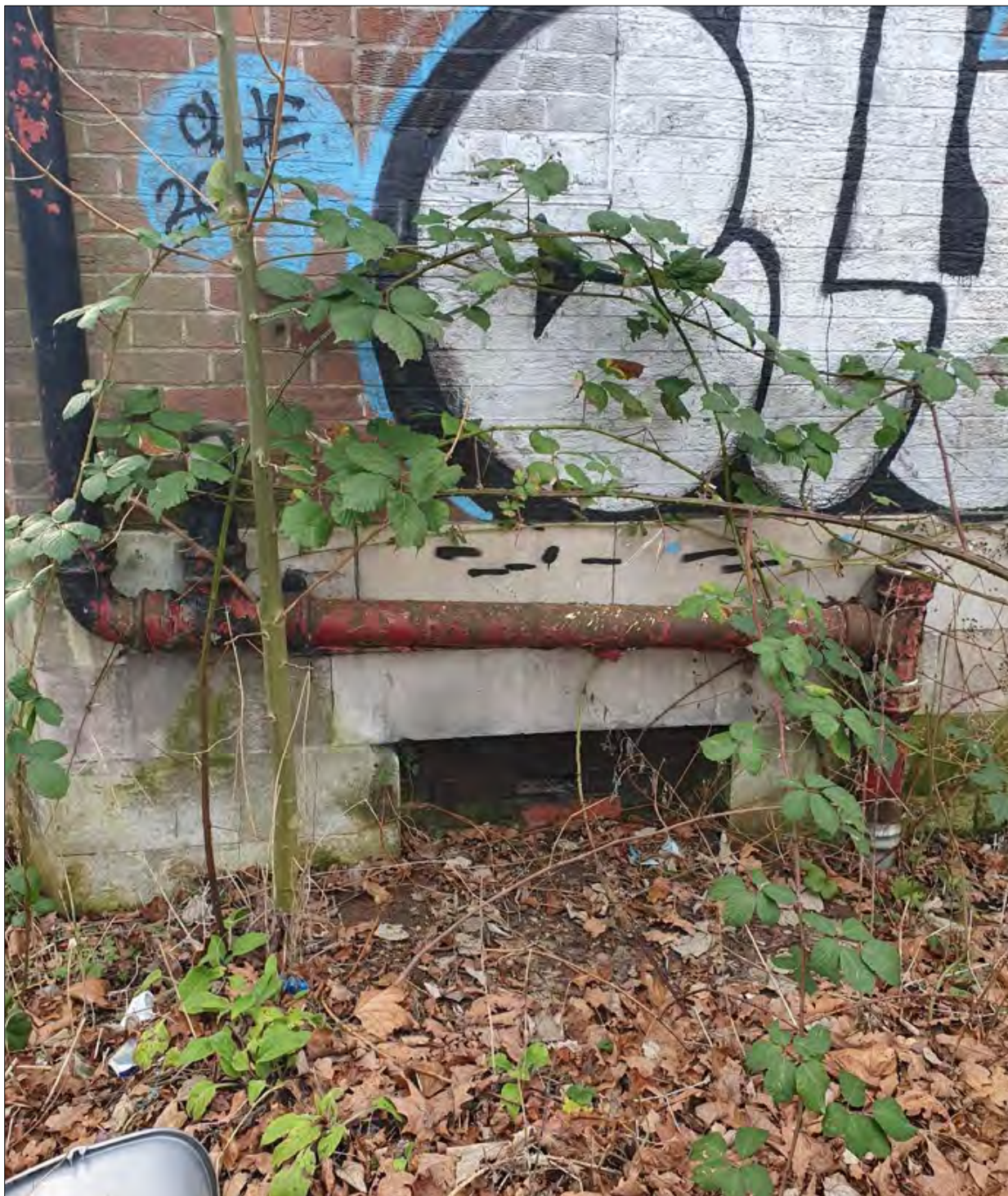
Plate 14 Photograph of Chorlton Baths, showing a cellar light, later bricked up, facing west
