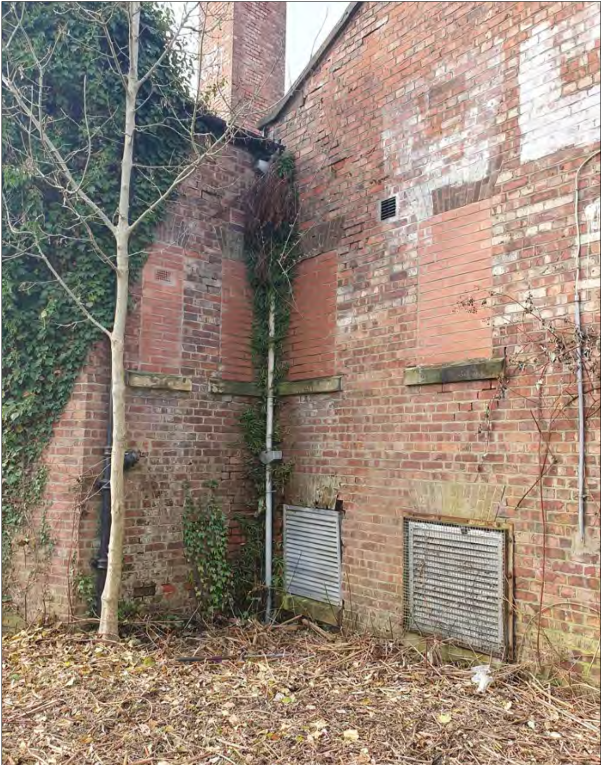
Plate 13 Photograph of Chorlton Baths, showing windows bricked up, facing south-west
