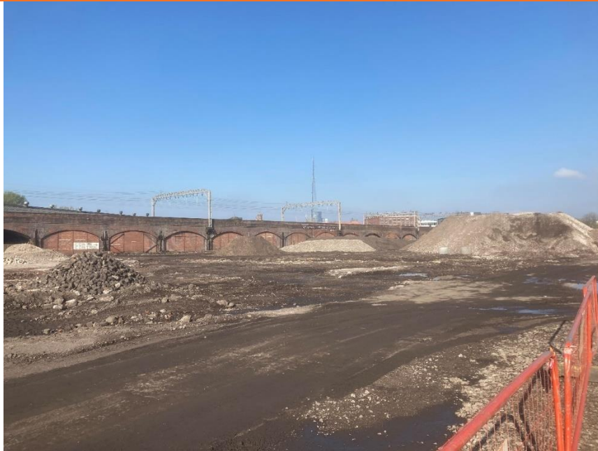
PLATE 6 COBBLES (AND COAL TAR) REMOVED – APRIL 2023
