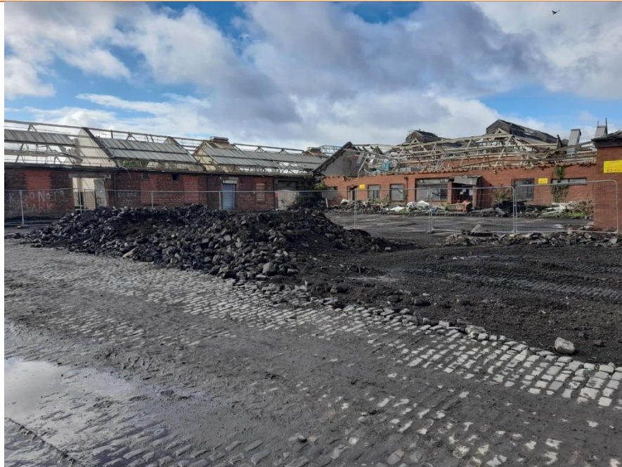
PLATE 3 COBBLE REMOVAL STARTING IN SOUTH OF THE SITE IN AUGUST 2022
