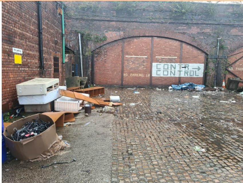
PLATE 1 COBBLES WITH COAL TAR SEALANT DURING E3P 2021 INVESTIGATION
