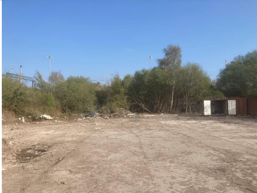
PLATE 5 COBBLES (AND COAL TAR) REMOVED – APRIL 2023
