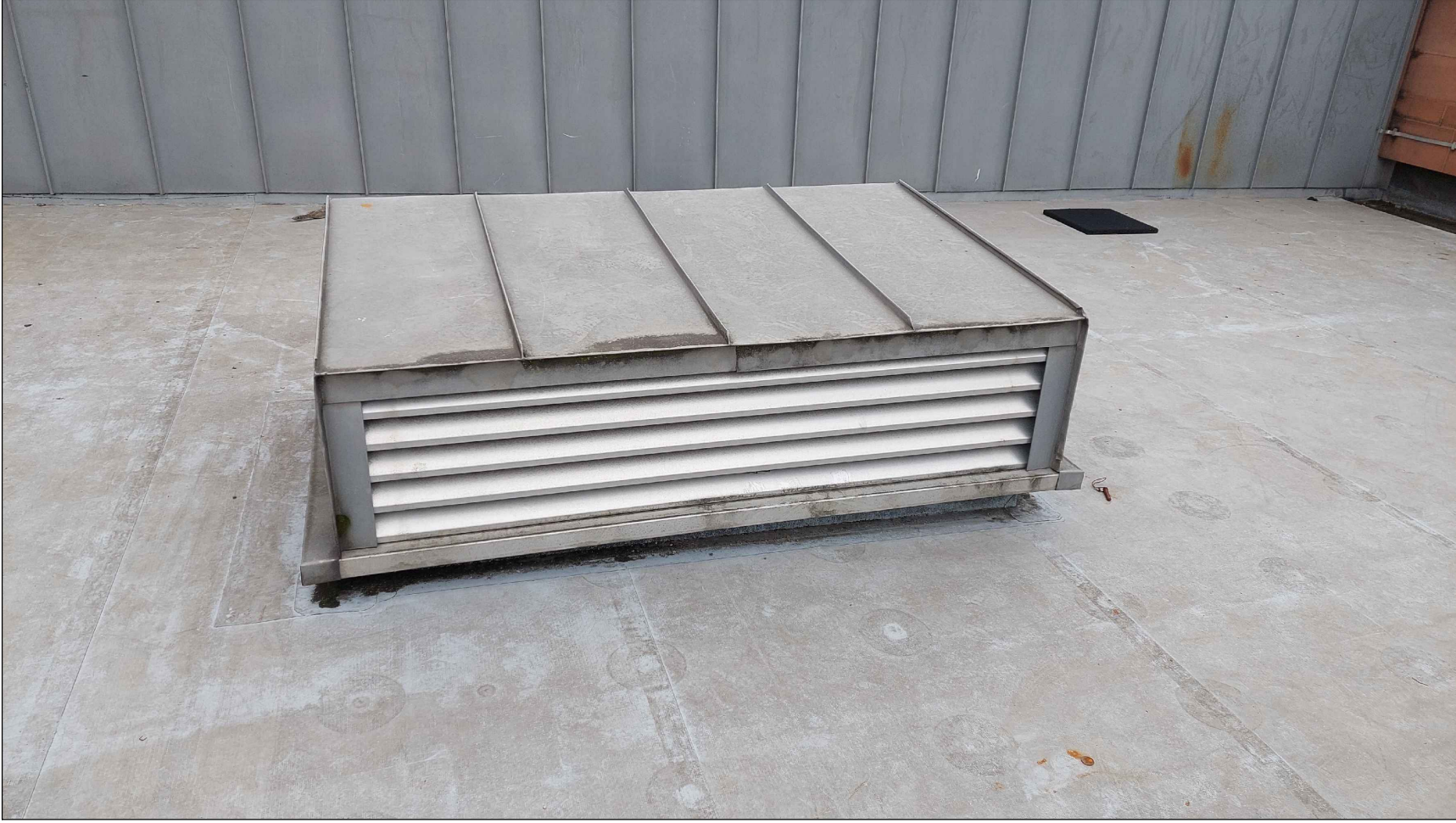
PHOTO 6 – EXISTING FRESH AIR AND EXHAUST PENTHOUSE LOUVRE TO BE REPLACED FOR NEW PENTHOUSE LOUVRE. COLOUR AND FINISH TO MATCH EXISTING
