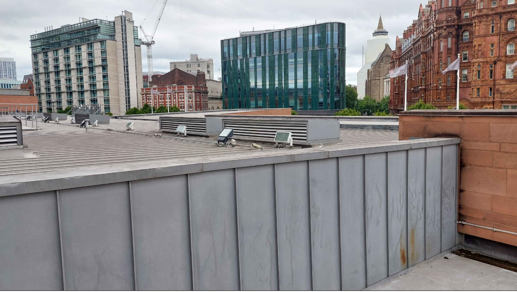
PHOTO 7 – EXISTING FRESH AIR AND EXHAUST PENTHOUSE LOUVRE TO BE REPLACED FOR NEW PENTHOUSE LOUVRE. COLOUR AND FINISH TO MATCH EXISTING
