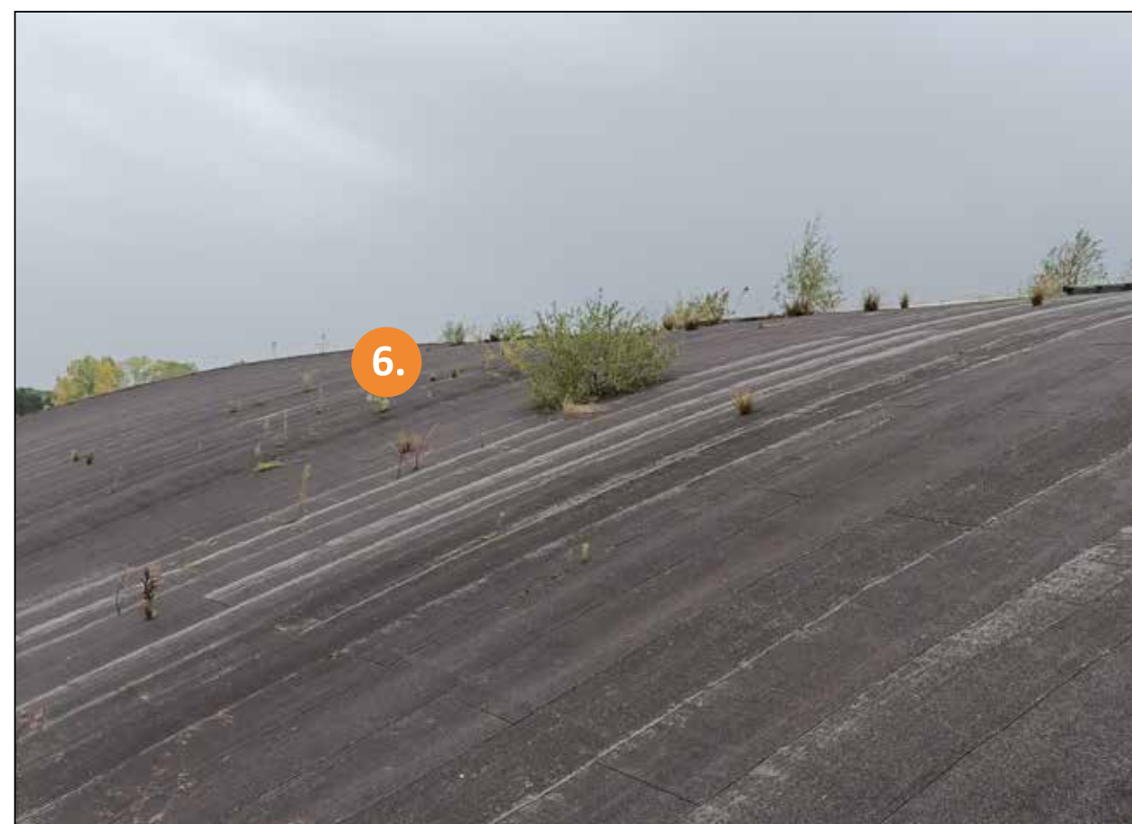
Photo of non-original felt roof covering
