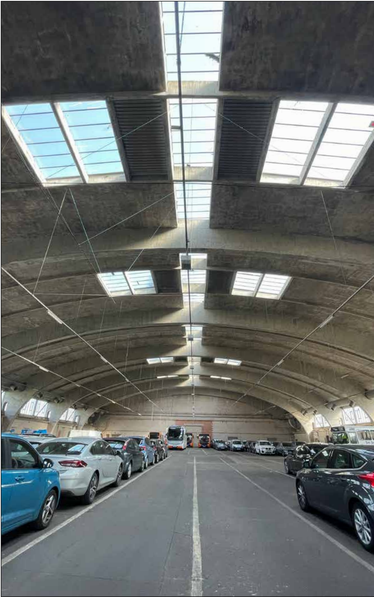
Internal photo of the Bus Garage
