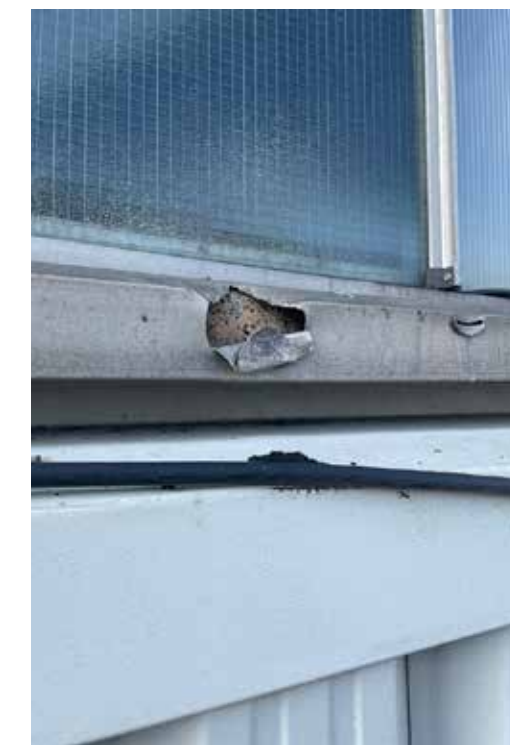
Existing glazing (wired).
