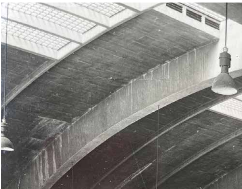
Detail of vents and glass block panels. Original design.
