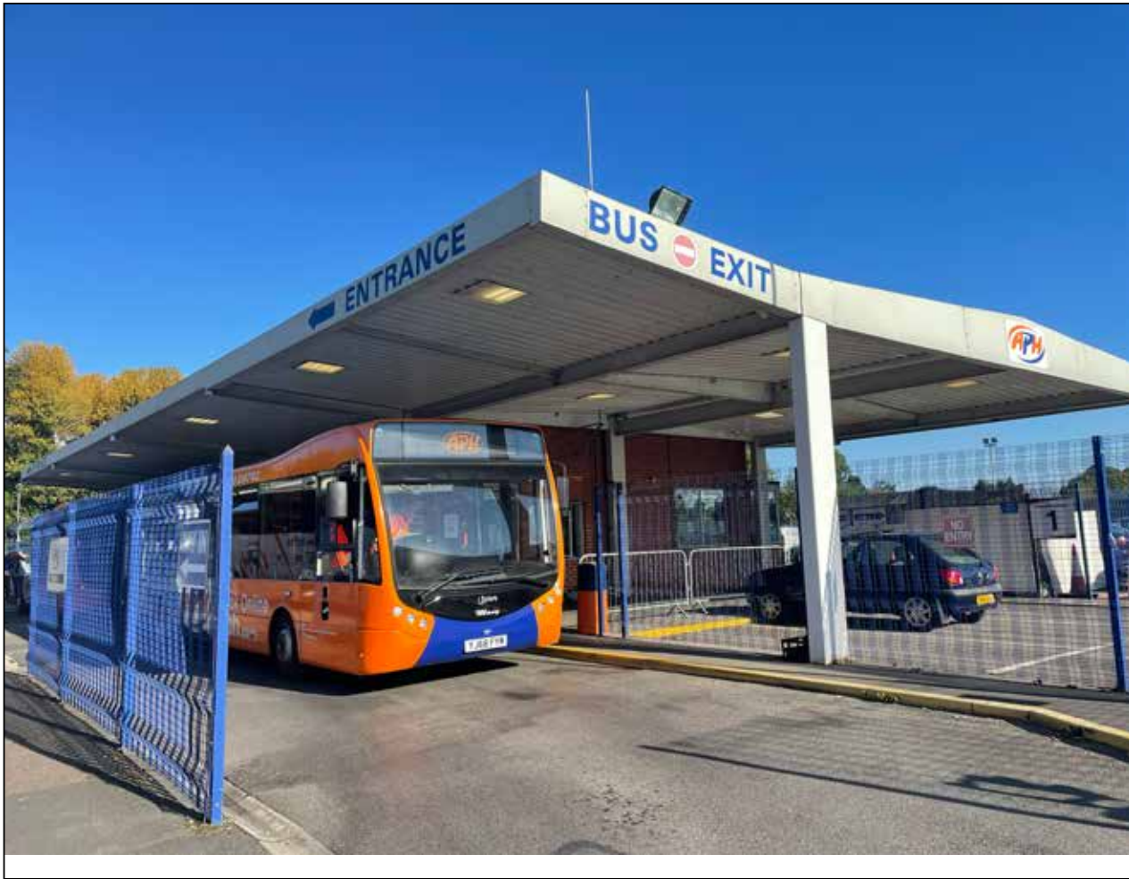
APH Reception Building front
