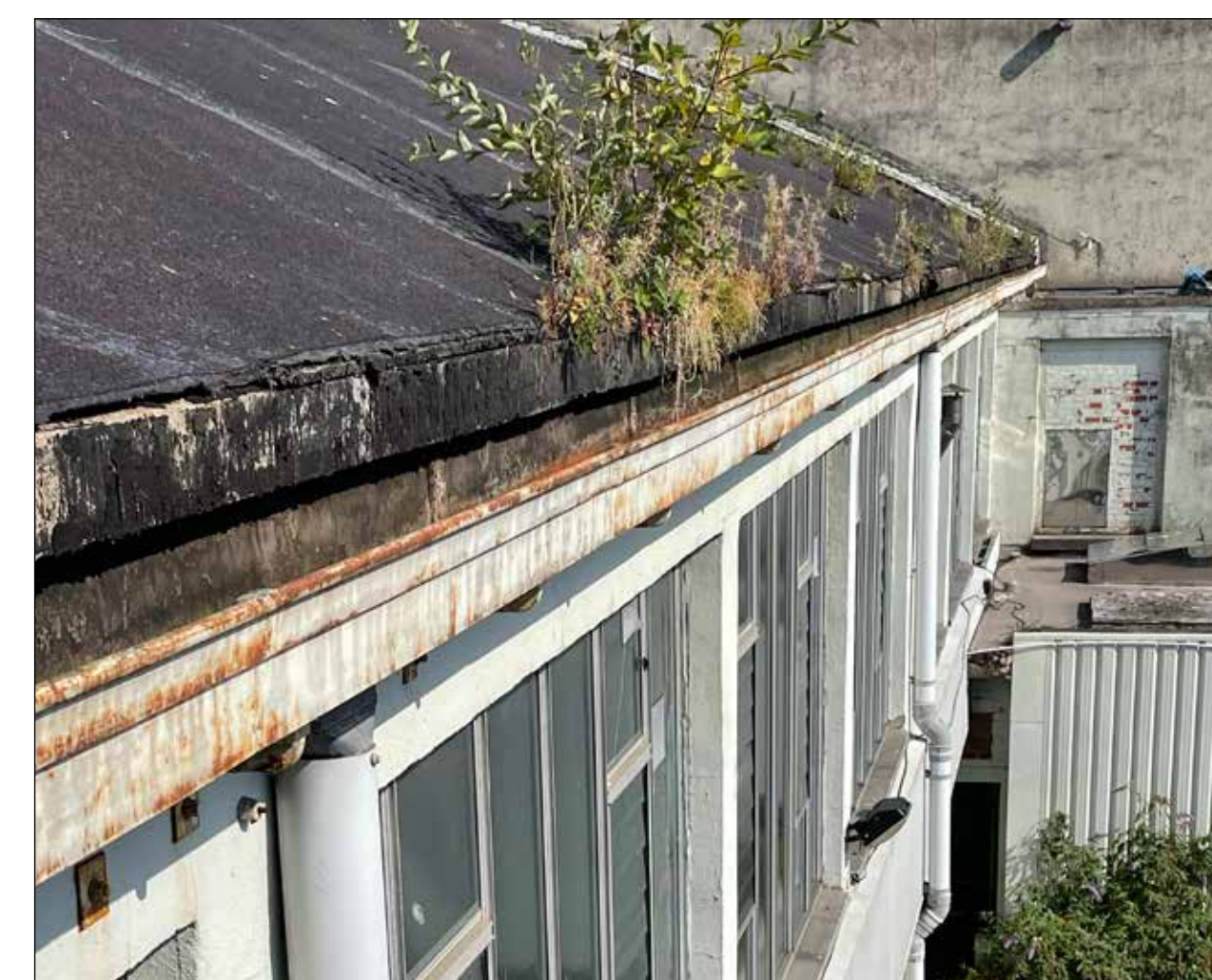
Photo showing vegetation growing on the Bus Garage roof
