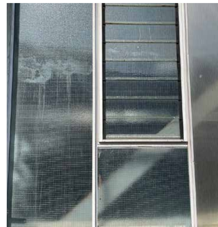
Existing louvred window panes to side elevation.
