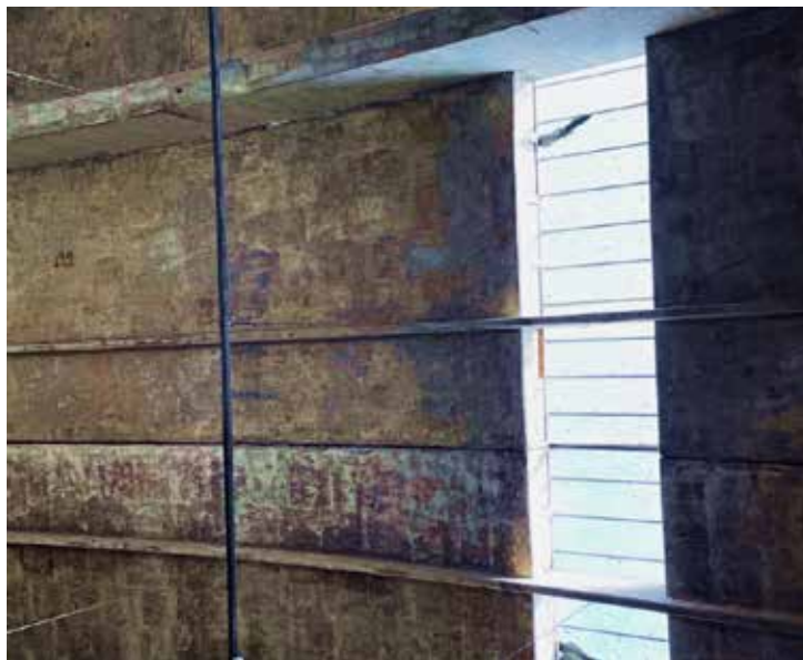
Existing replacement glazing.
