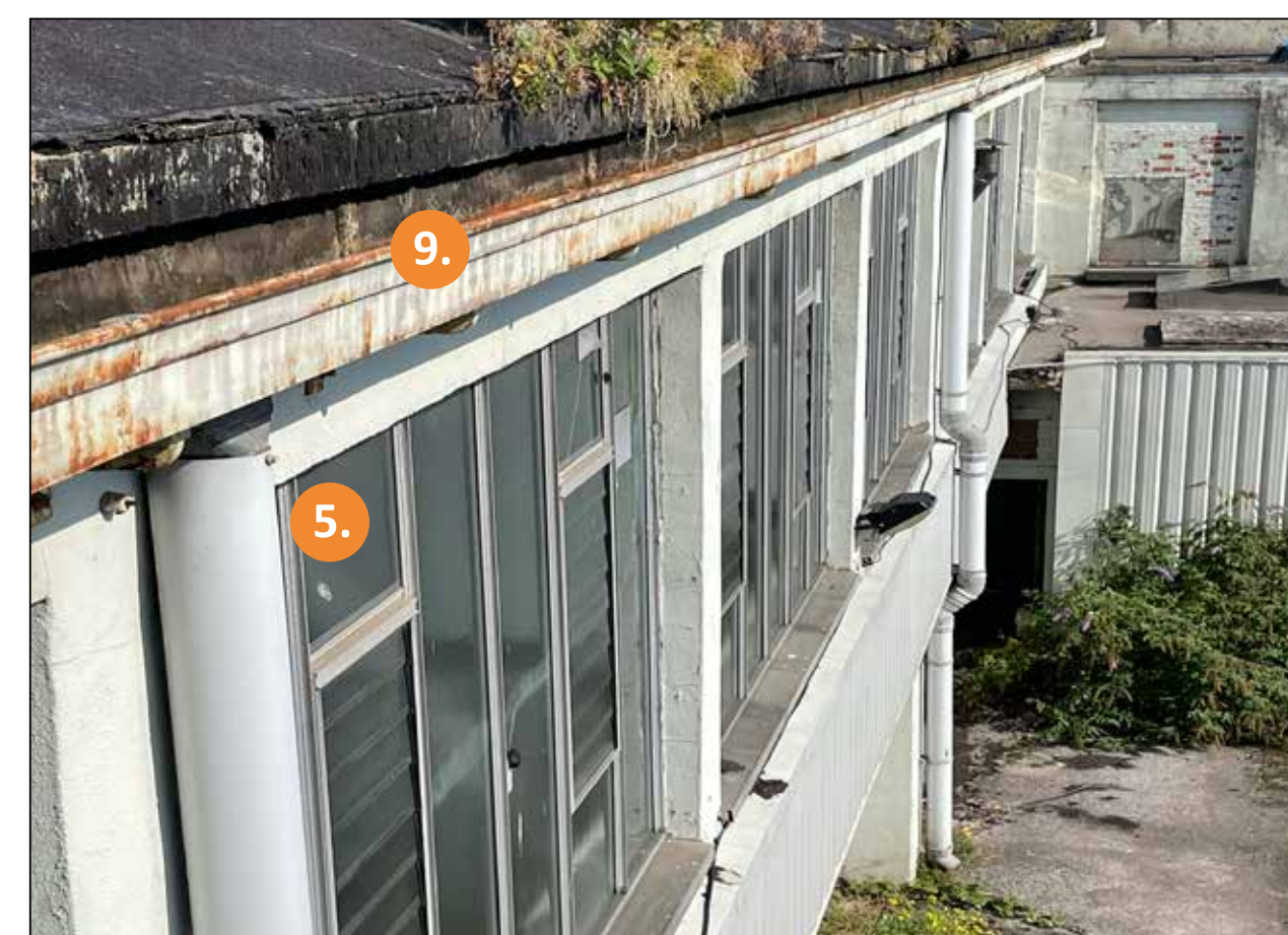
Photo of existing gutters, downpipes and aluminium framed windows
