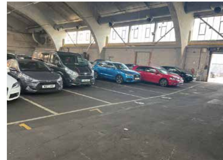
Existing side windows.
