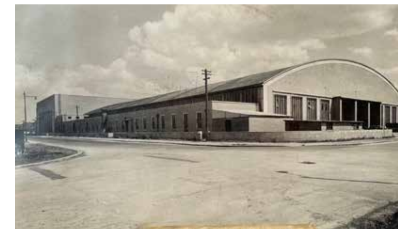
Original windows to side, with wing (now demolished).
