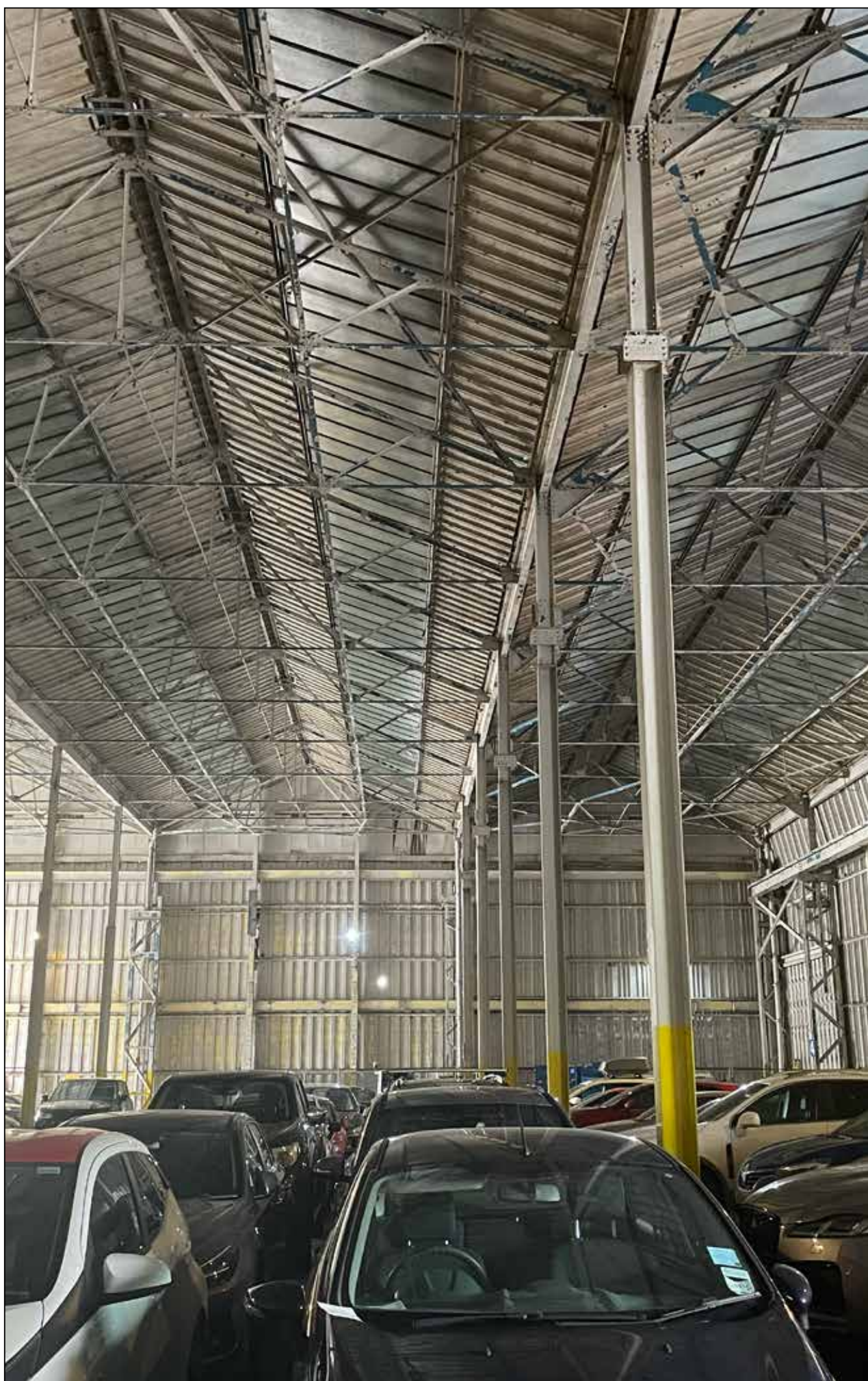
Internal photo of the warehouse, to be removed
