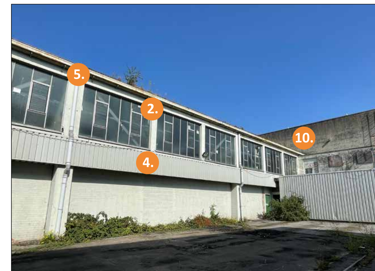
Photo of south east elevation showing some of the non-original windows and metal cladding
