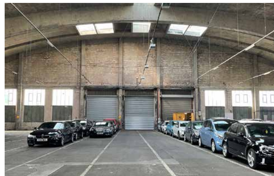
Current arrangement to front, with lower windows blocked.
