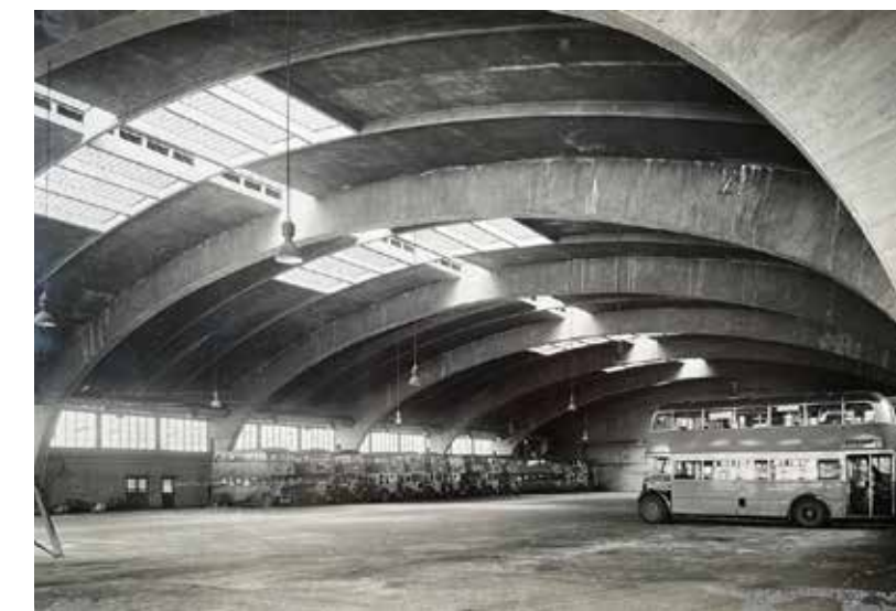
Former windows to side elevations, internal view.
