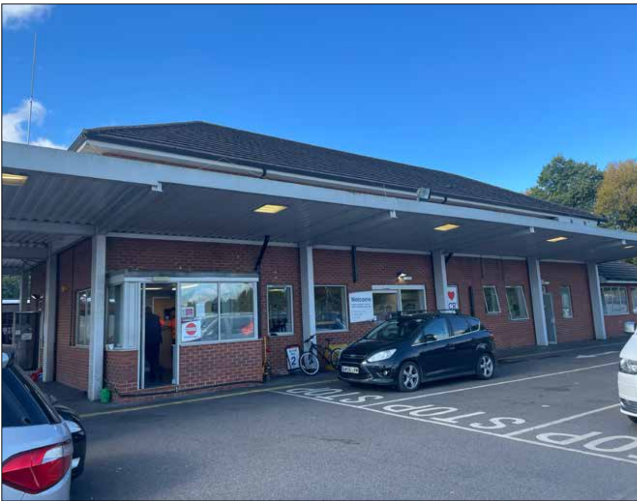
APH Reception Building rear
