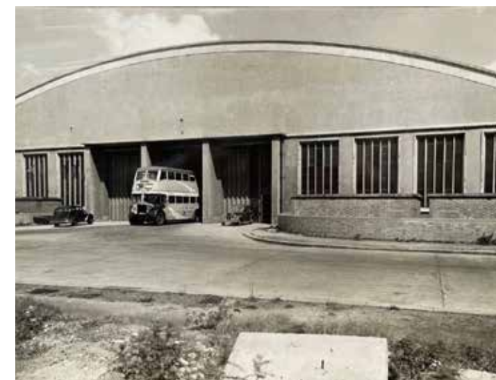
Original front windows, almost full height.
