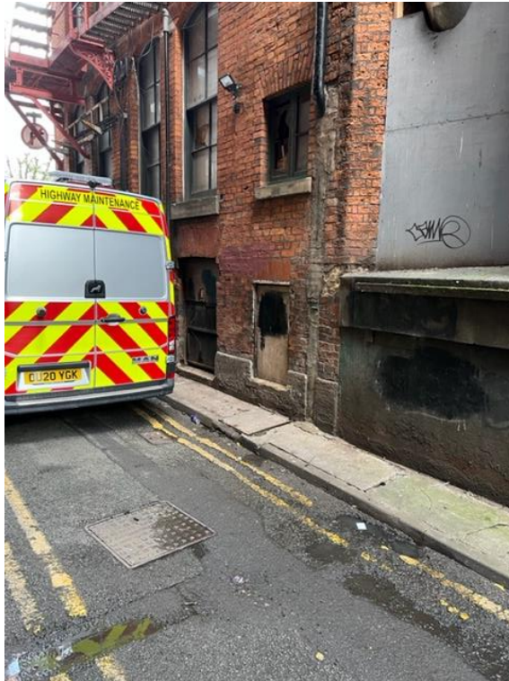
Photo 9, Public sewer manhole location
