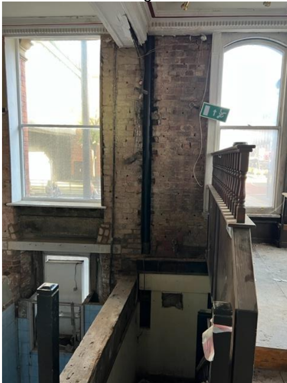
Photo 2, A number of rainwater pipes have been exposed in the wall - assumed to discharge to MH02 and MH01
