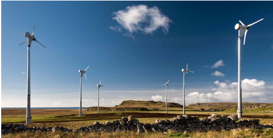
Figure 16: Typical Small Scale 6kW Wind Turbine
