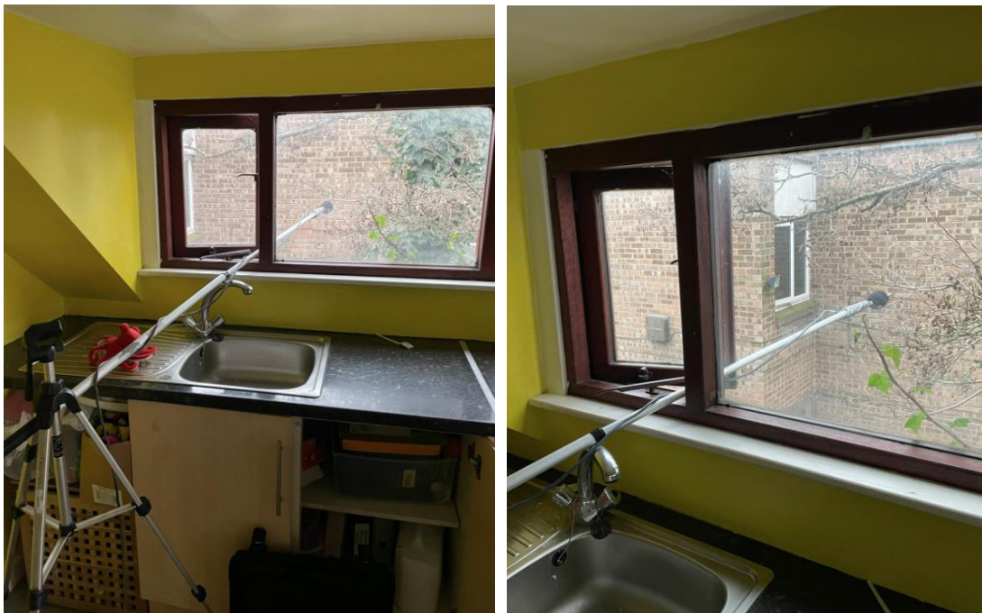
Figure 3 - Noise Measurement Position Photographs (Internal)
