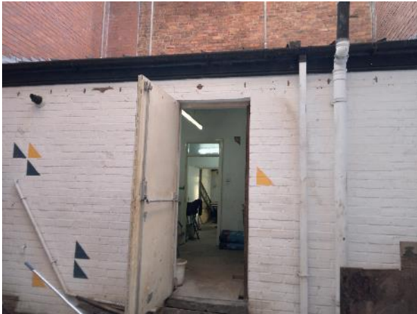
Single storey extension on northeast elevation
