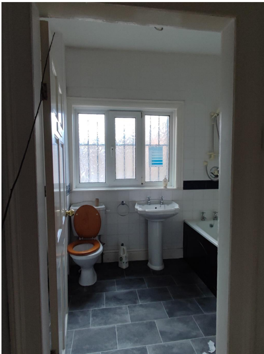
Figure 31 – View Southeast towards the existing first floor WC.
