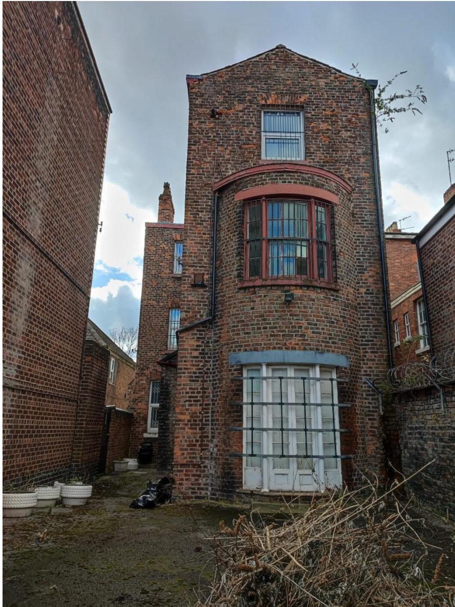
Figure 05 – View Southwest towards rear elevation
