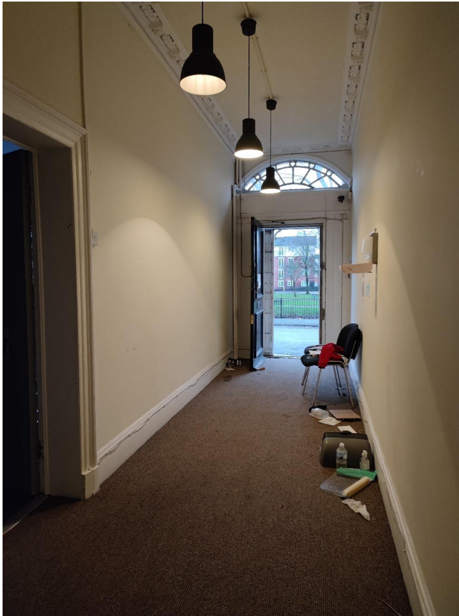
Figure 09 – View Southwest towards front entrance Existing to be retained
