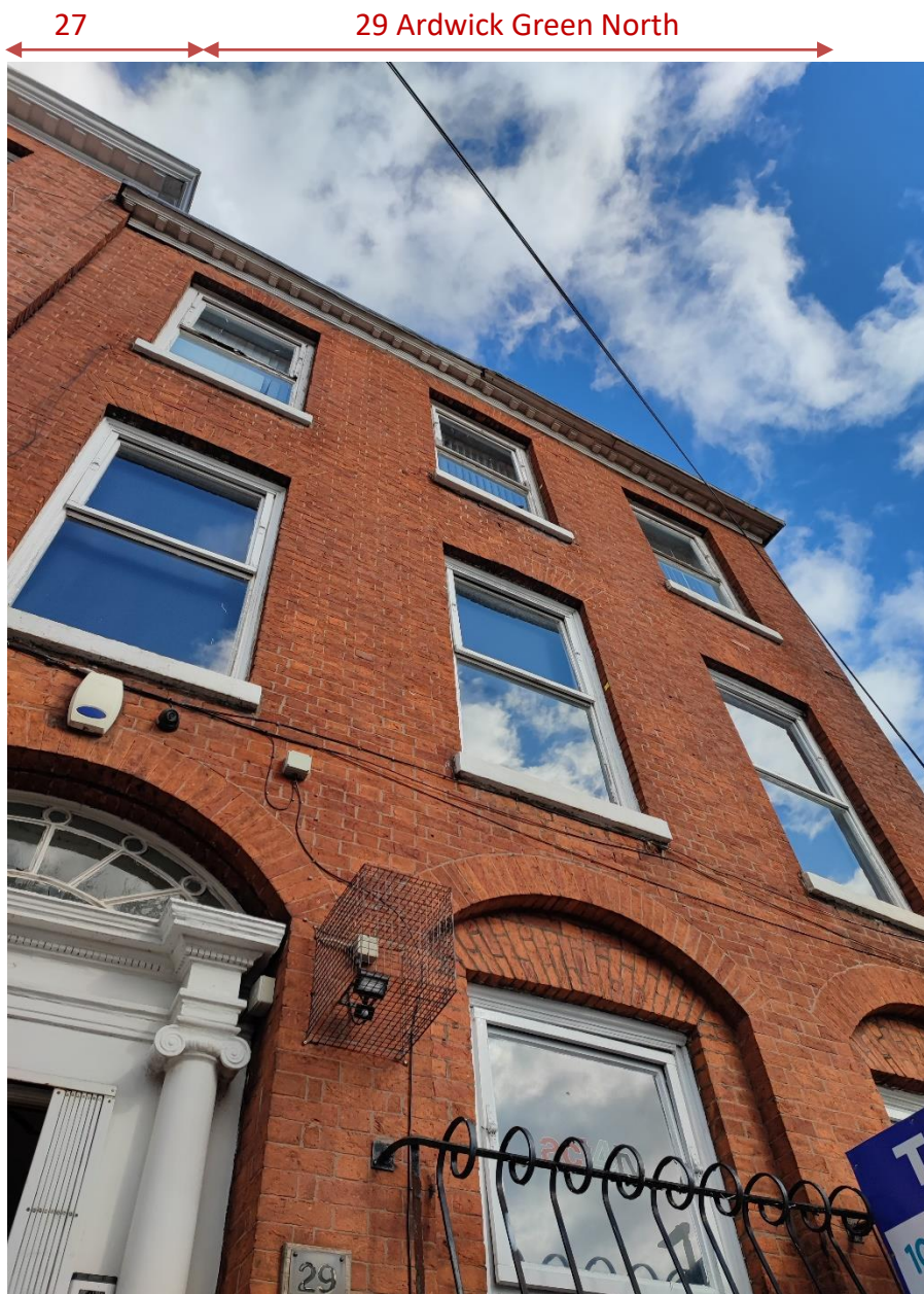
Figure 02 – Front Elevation view towards to the windows on the upper floors No change to front windows
