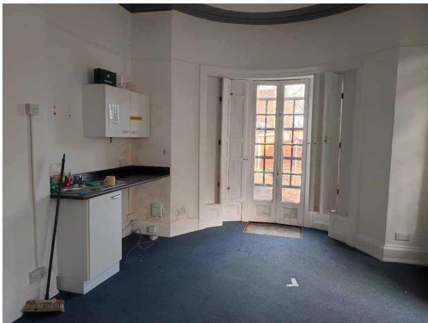
Figure 17– View Northeast towards rear yard from the rear office room. Existing kitchenette to be removed. Make good where required.
