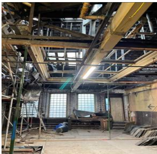
IMAGE 22: Upper floor number 12 post removal of ceiling.
