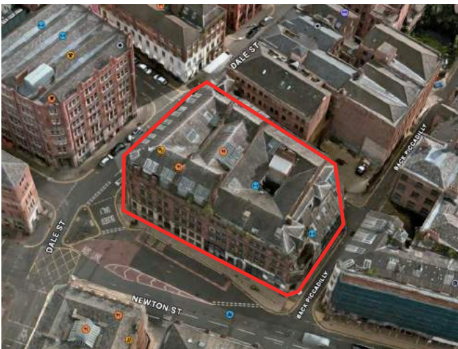
IMAGE 24: Aerial view of 8-16 Newton Street.
