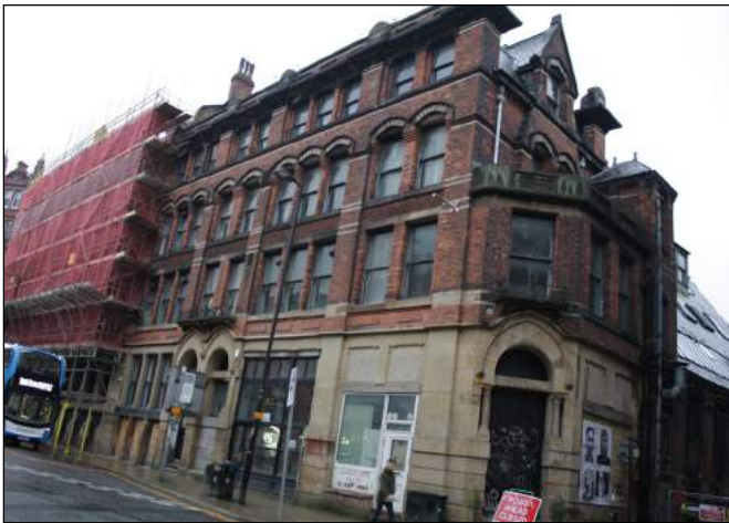
IMAGE 2: External street view of 8-16 Newton Street.
