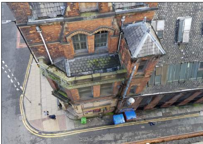
IMAGE 21: Existing Aerial View - Second Floor Breakout Space
