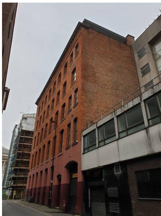
Image 5: North and visible part of west elevation
