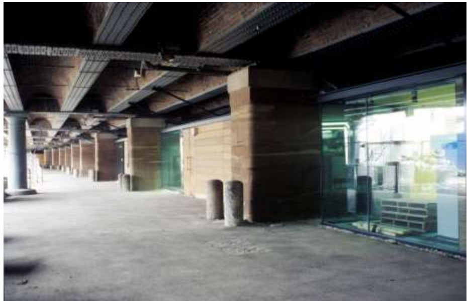
Underside of Viaduct (Colonnade) with Collection Stores
