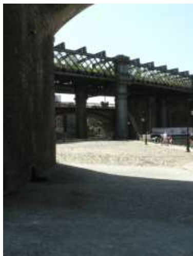
Cast-iron lattice-work and columns of viaduct
