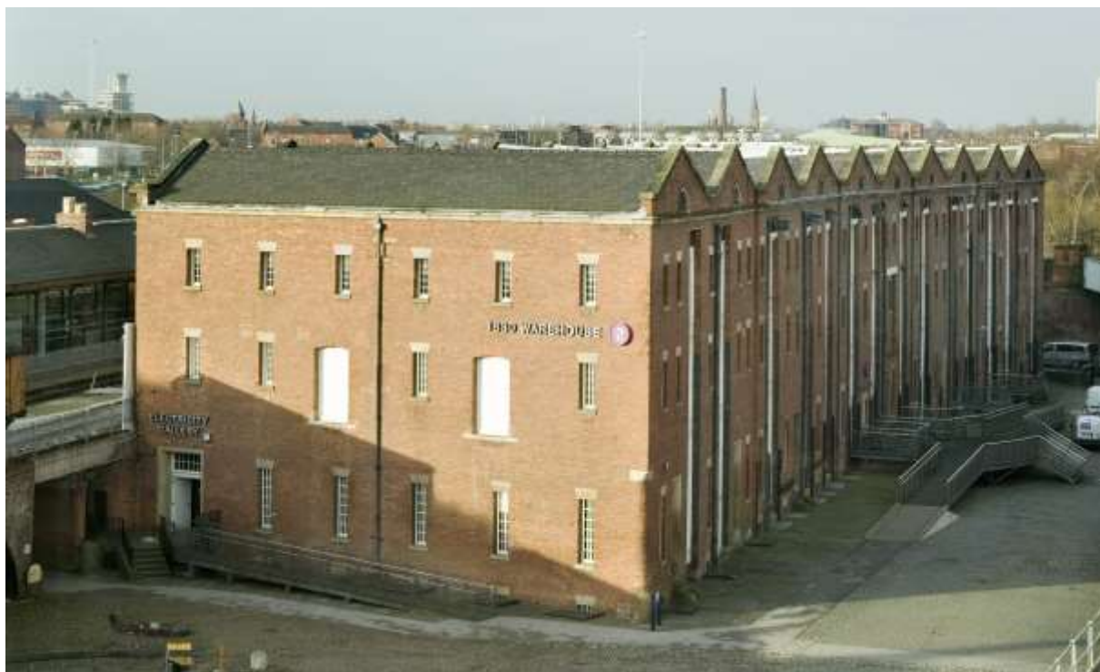
East and north elevations of 1830 Warehouse.
