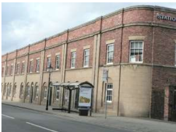
Liverpool Road elevation of former Carriage Shed & Shops
