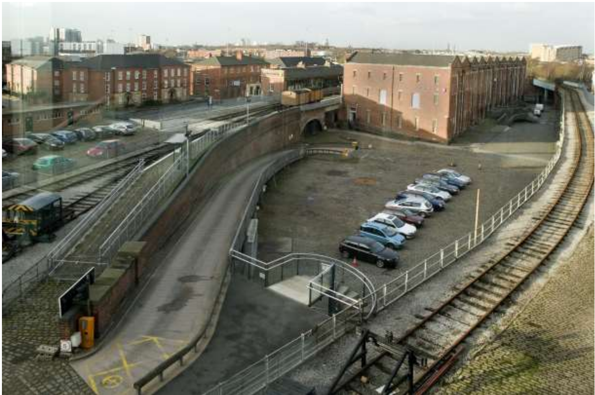
Lower Yard: with 1830 Viaduct and Car Ramp to left and 1867 Viaduct to right
