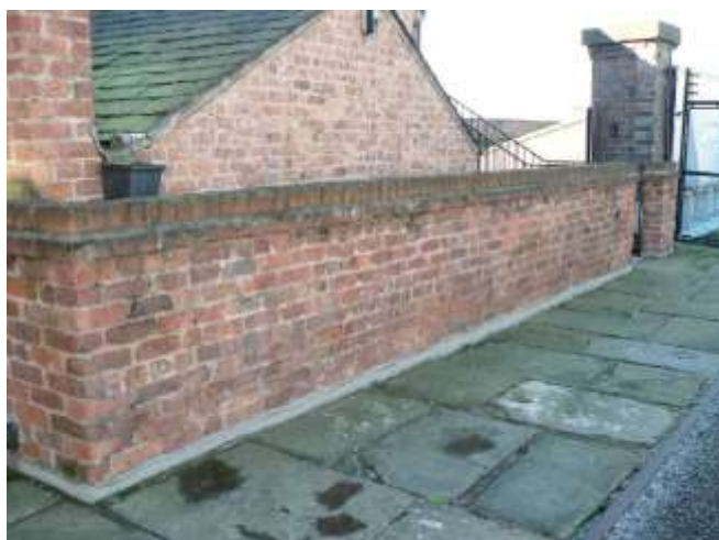
Rear of Station Master's House, as seen from the platform
