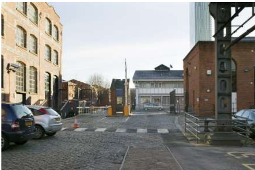
Upper Yard and Lower Byrom Street entrance, with crossing from Main Building to Power Hall
