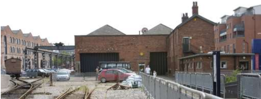
View of buildings at eastern end of site: Main Building, Power Hall & Gantry, Curatorial Centre
