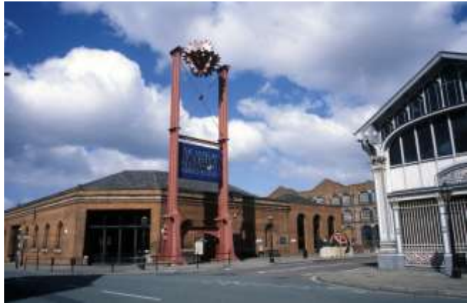
Corner of Liverpool Road and Lower Byrom Street
