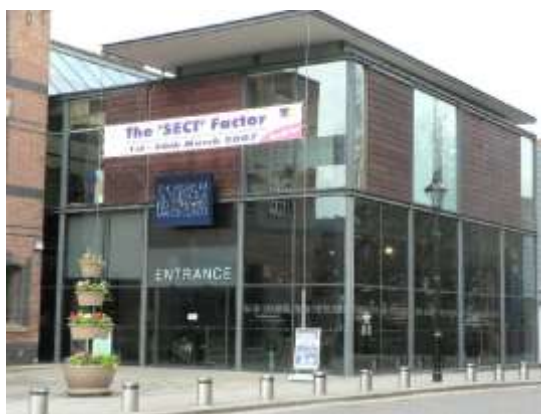
Modern entrance on north-east corner of Main Building
