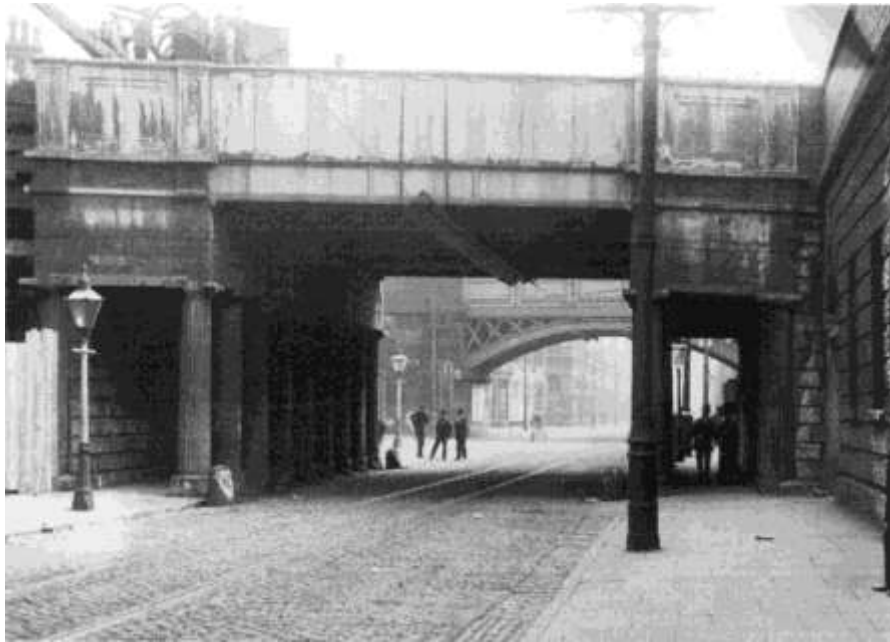
Original (1830) Water Street Bridge
