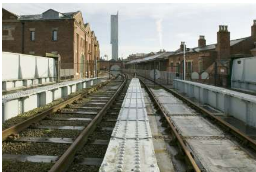
View of Viaduct, looking along tracks from Water Street Bridge
