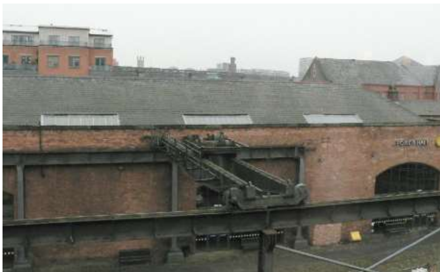
Power Hall and Gantry from north
