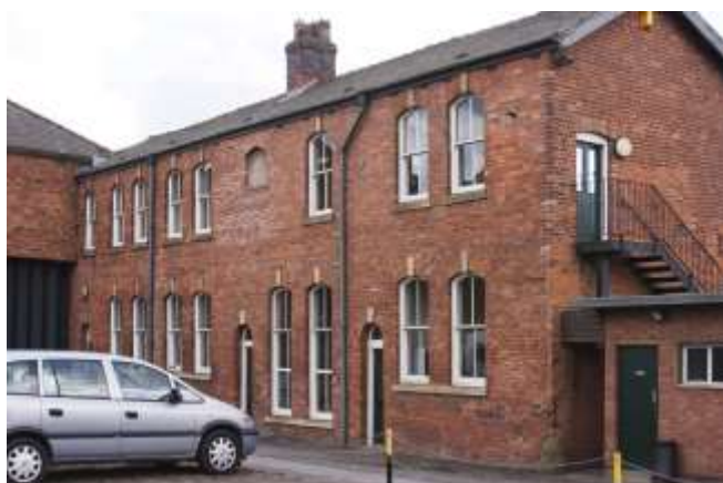
Curatorial Centre from central Upper Yard
