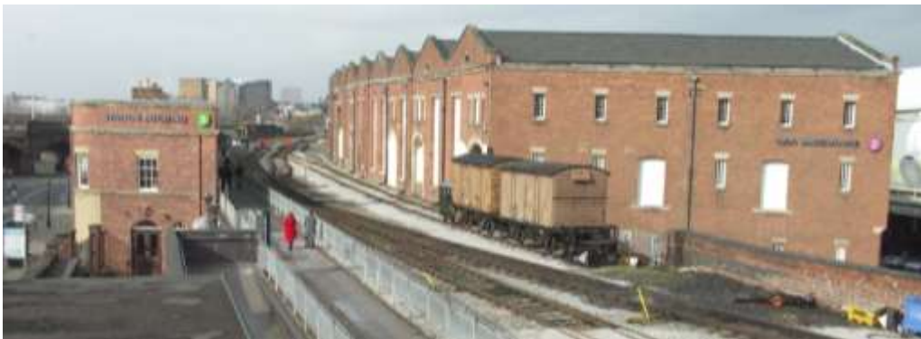
View of buildings at western end of site: Station Building and 1830 Warehouse
