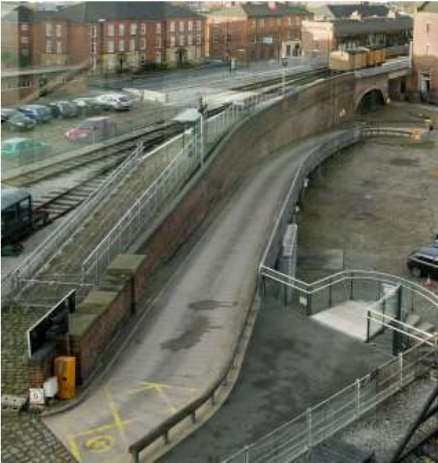
Car Ramp from Upper Yard end
