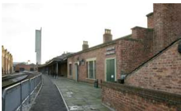
Station Building looking towards Power Hall
