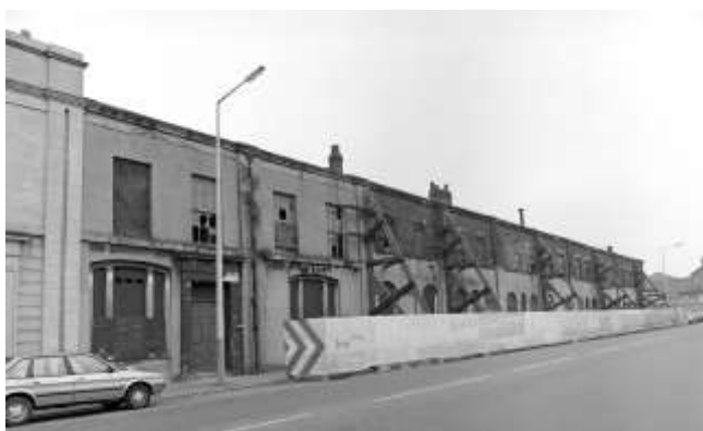
Liverpool Road façade
