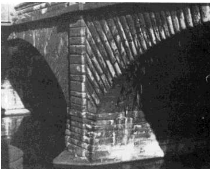
Central pier of the Irwell Bridge
