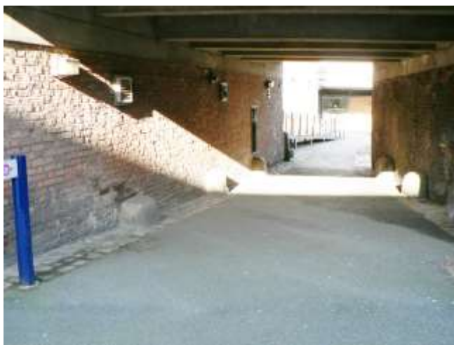
Tunnel under Viaduct through to Lower Yard
