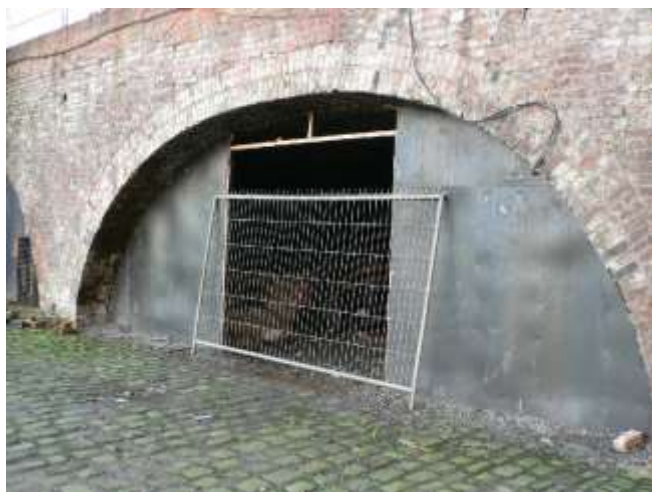
External view of lower Viaduct
