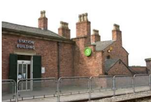
Station Building from tracks and Station Master's House to right
