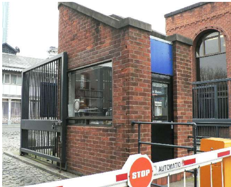
Gatehouse, metal gates and automatic barriers
