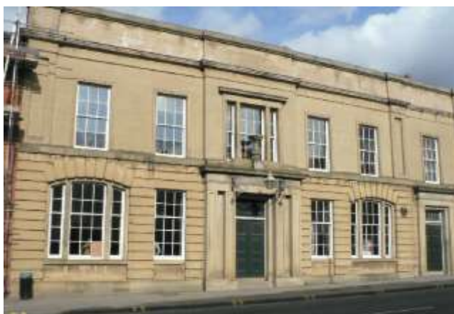
Station Building. To left is Station Master's House (not shown) and to right are former Shops and Carriage Shed
