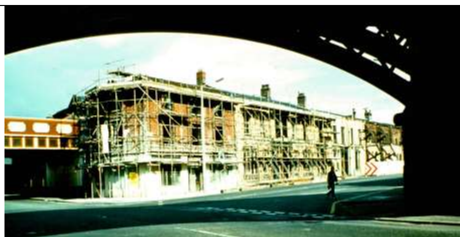
The Station Master's House and Passenger Station scaffolded during restoration, 1981
