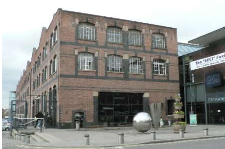
Lower Byrom Street elevation of Main Building, with modern entrance extension to right
