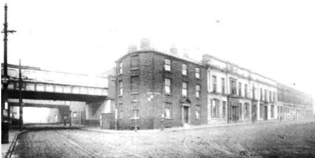
New (1905) Water Street Bridge
