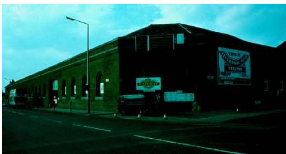
The Power Hall from the south-east, 1980
