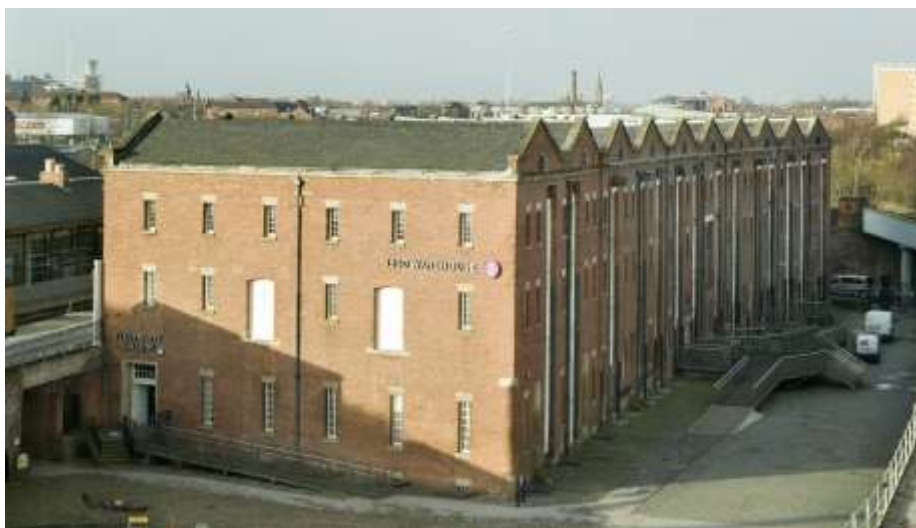
Disabled access to ground floor of 1830 Warehouse on north (Reception) and east (Electricity Gallery) sides
