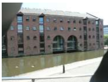
Merchants' Warehouse, Castlefield Basin
