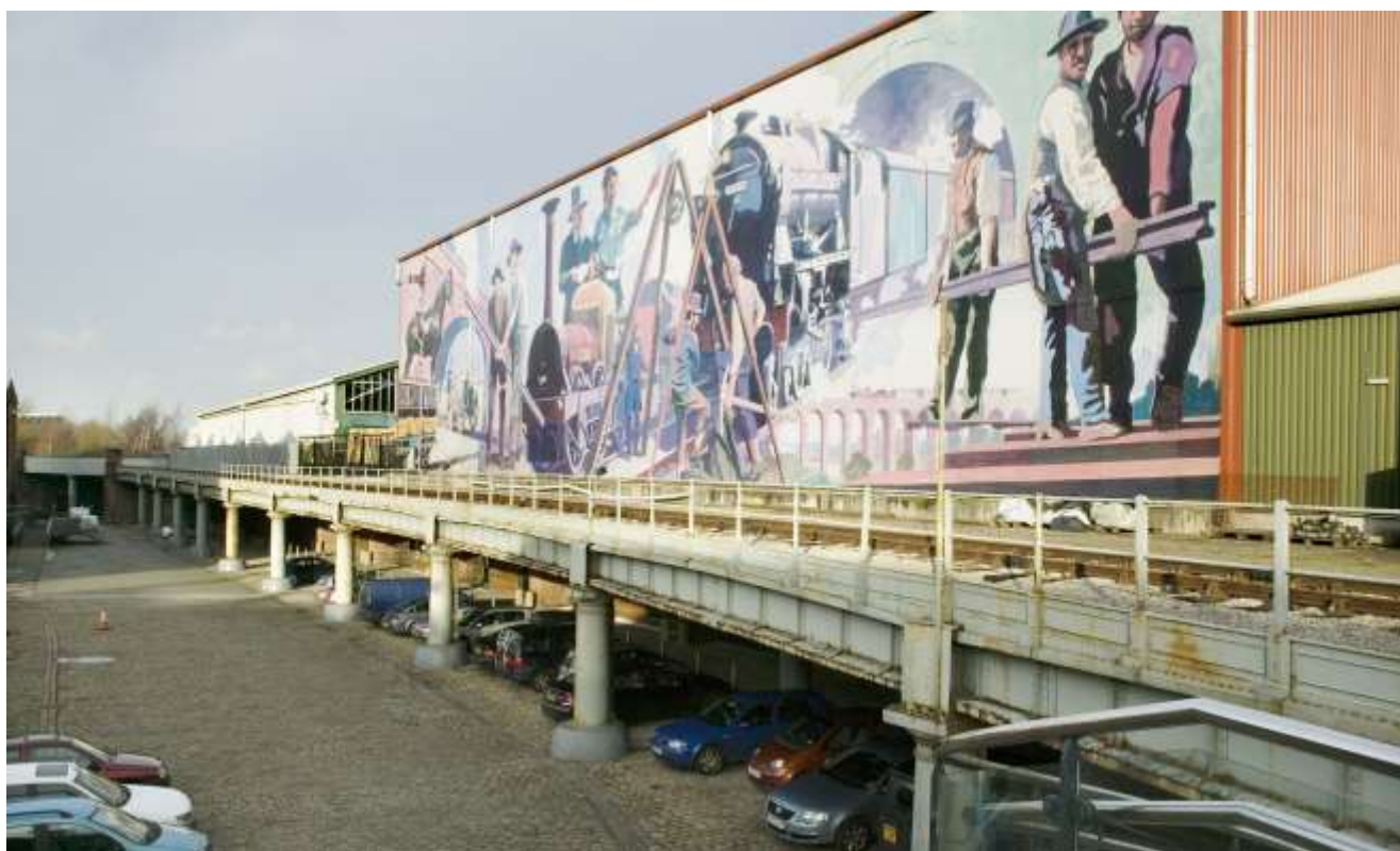
Recent photo showing 1867 Viaduct, including Colonnade and mural on side of a Granada Television shed.
