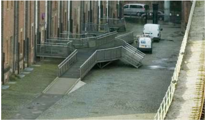
Ramps in Lower Yard for access to ground floor of 1830 Warehouse
