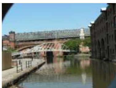
Curvilinear bridge in front of railway viaduct
