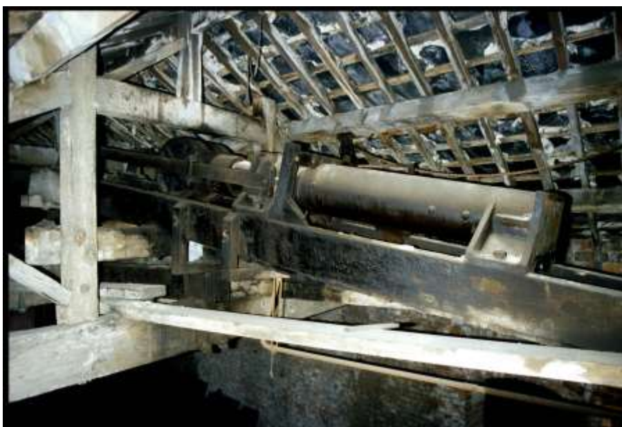
Hydraulic jigger in 1830 Warehouse
