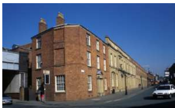
Station Building from Water Street, looking along Liverpool Road
