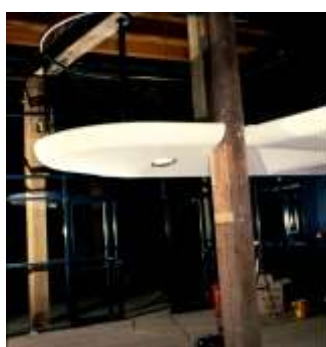
New stairwell in Bay 3, ground floor with mezzanine-level landing
