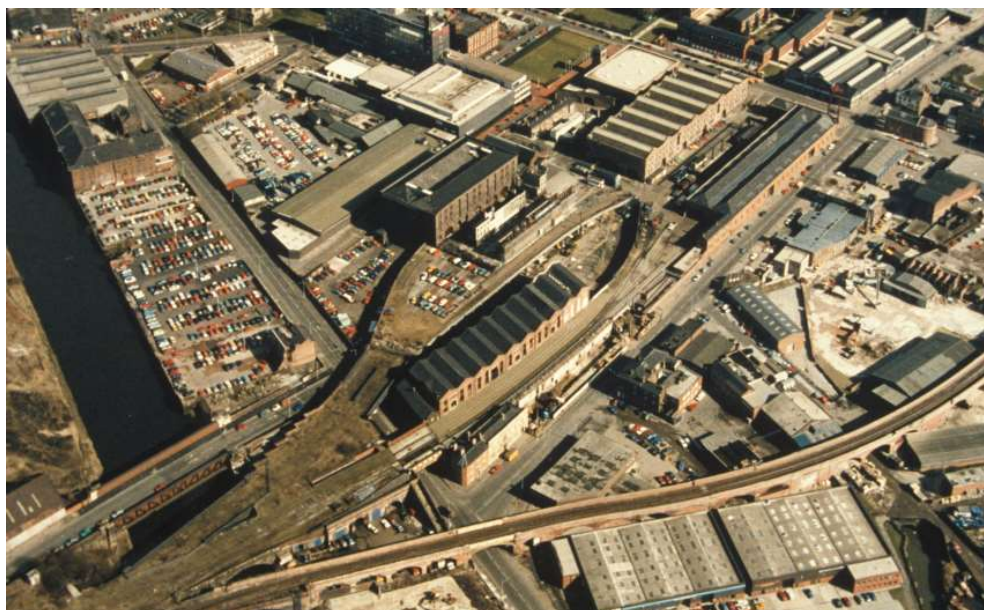
Aerial view of site
