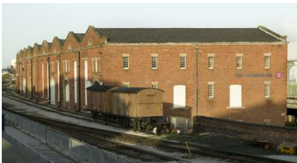
The 1830 Viaduct and the 1830 Warehouse
