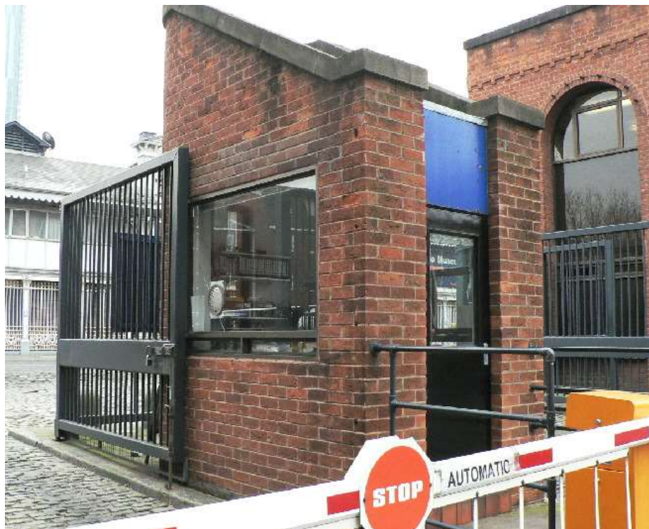
Intrusive: Gatehouse and Barriers at Lower Byrom Street Entrance
