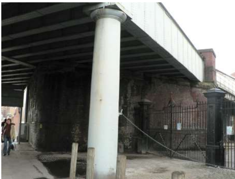
Bridge over Water Street with 1867 Viaduct entering Liverpool Road Station
