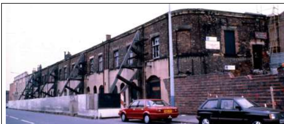
Propped Liverpool Road elevation of the Carrier's Offices, Shops and Carriage Shed prior to restoration
