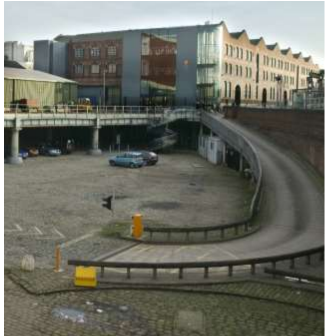
Car Ramp from Lower Yard end
