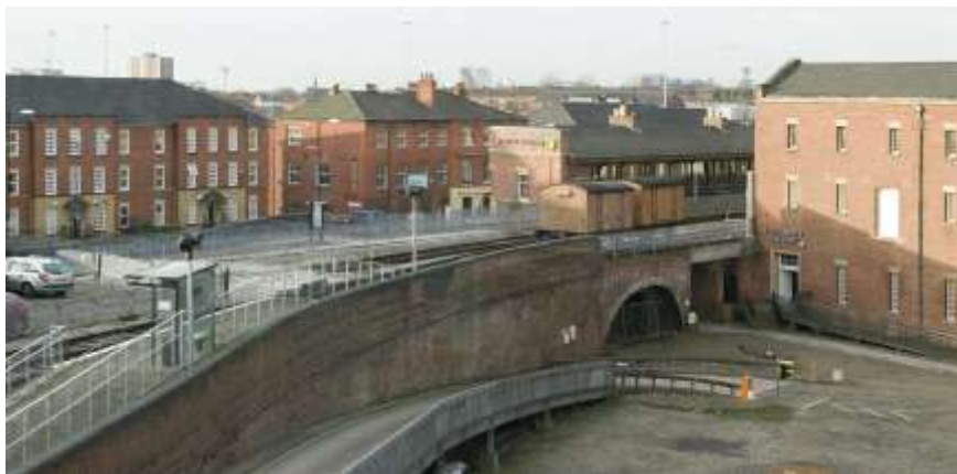
Eastern end of Viaduct, looking across Lower Yard
