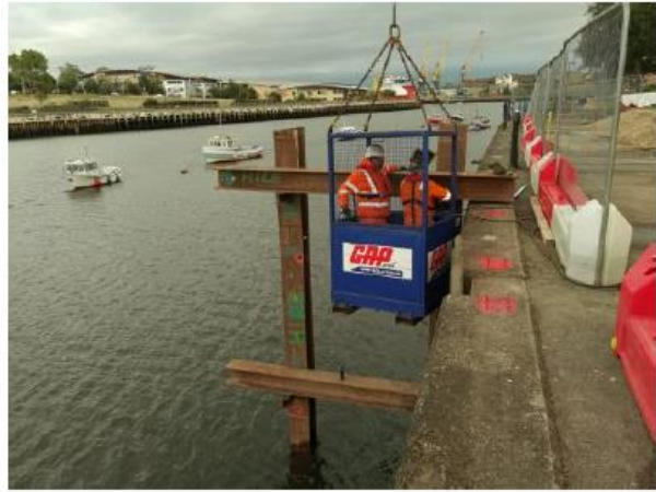
Cross head beams
