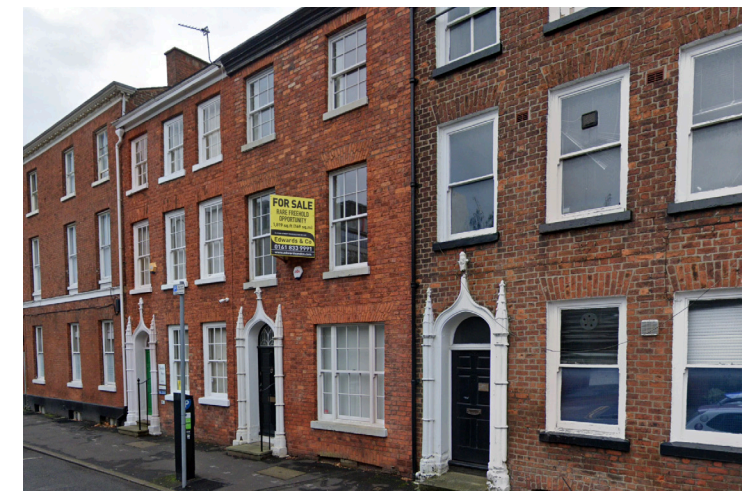
Georgian terraces on Byrom Street
