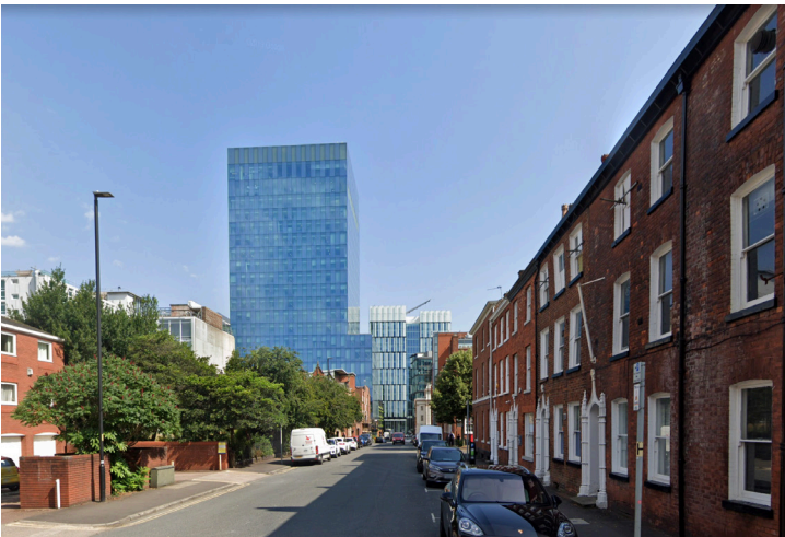
View down Byrom Street from Camp Street
