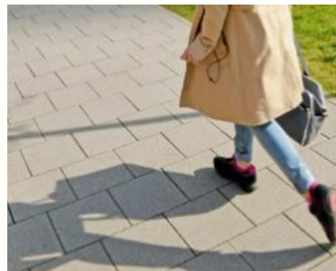
Concrete slab footpath
