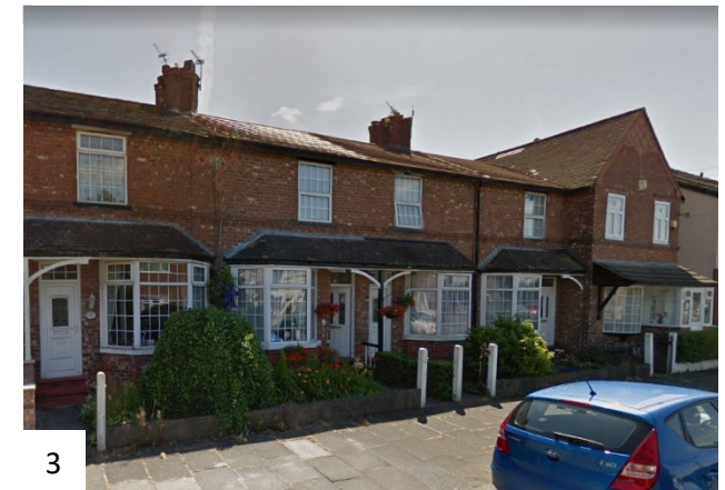
3 Residential House (C3 Use – Terraced Houses) (All images taken from Google Maps, 2015)
