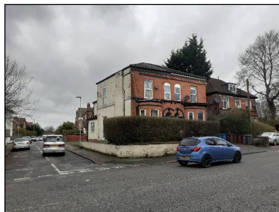
Figure 4: View of the site from Middleton Road.
