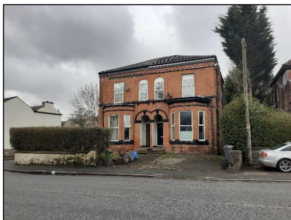
Figure 3: View of the site from Middleton Road.
