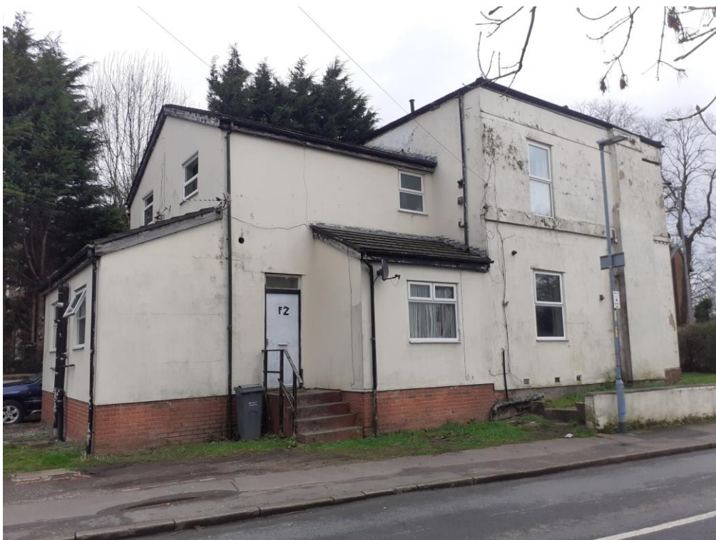
Moxley Road and rear elevation of 27 -29 Middleton Road.
