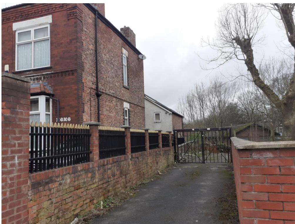
Driveway at the rear of the site adjacent to 2 Moxley Road.
