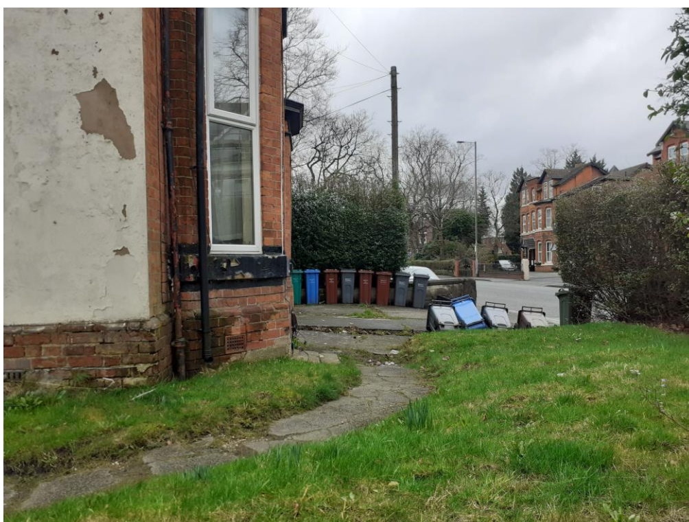
View across the front of 27 -29 Middleton Road.
