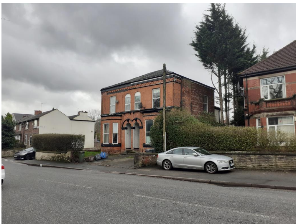
27 - 29 Middleton Road with 25 Middleton Road visible in the background.
