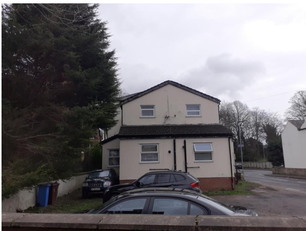
Rear of 27 – 29 Middleton Road.
