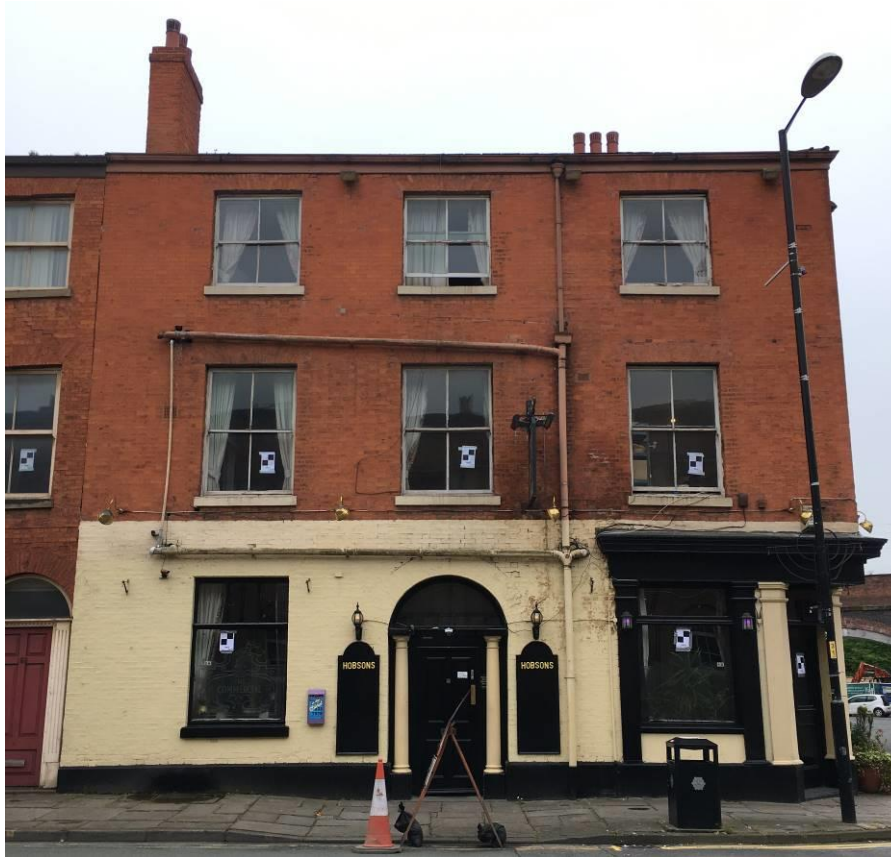
Figure 39 – The front (north) elevation of the Commercial Hotel (No. 125 Liverpool Road).
