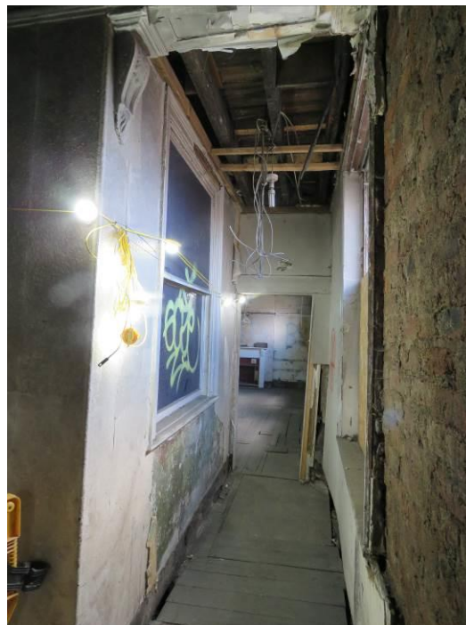
Figure 143 – Looking south from corridor 1F07 into the 1830s extension (1F09/10/11).
