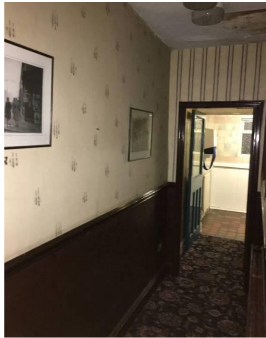
Figure 53 – The rear corridor (GF3) which would originally have linked the hotel to the original rear buildings in the yard. This corridor was removed when the stables were demolished and now lead into a modern toilet (GF9).
