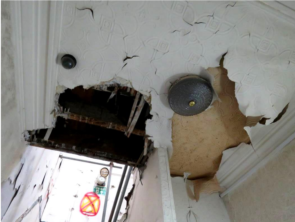
Figure 123 – The original lath and plaster ceiling, cornice and decorative ceiling paper that can be seen to largely survive to the landing ceiling.
