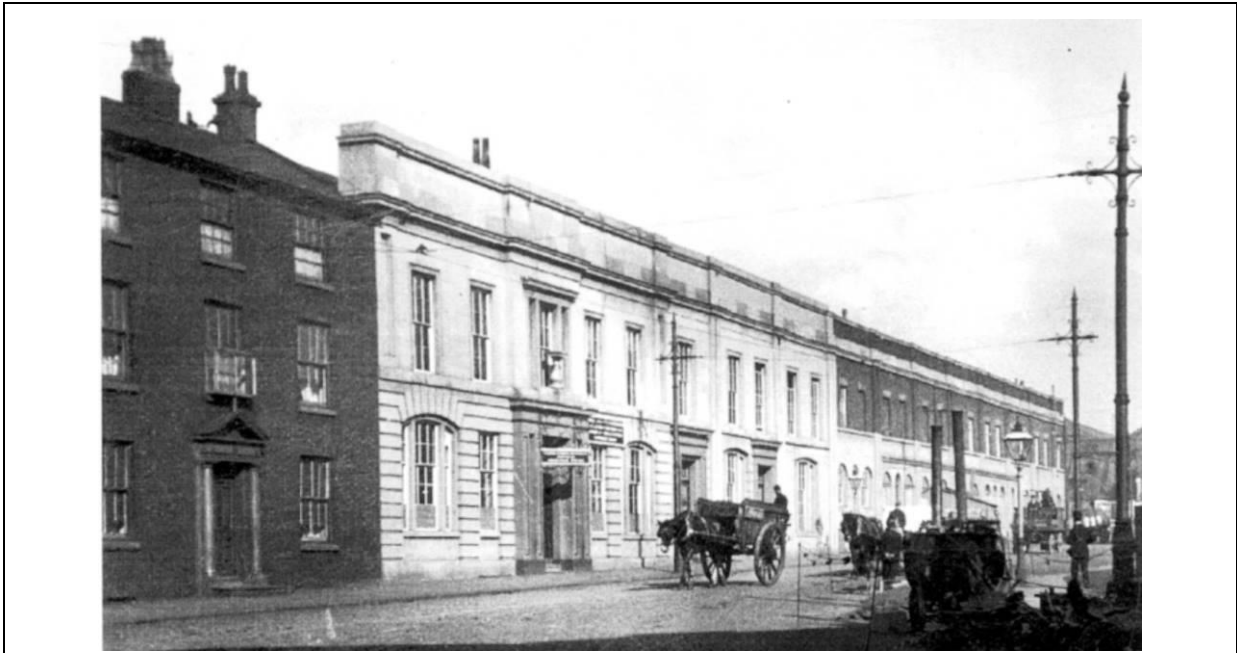
Figure 6: The station buildings as they appeared in 1902 when used as a goods station. The Site is located just off the image to the right. (Source Manchester Local Imaged Archive).
