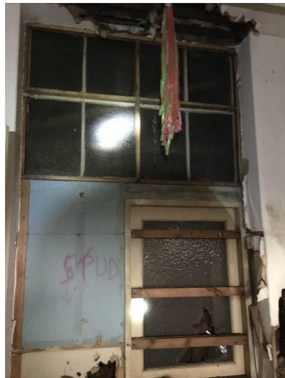
Figure 32 – The last surviving original eight-over-eight
