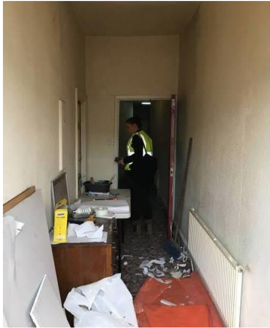
Figure 65 – Looking north along the inserted fire escape corridor (2F10).
