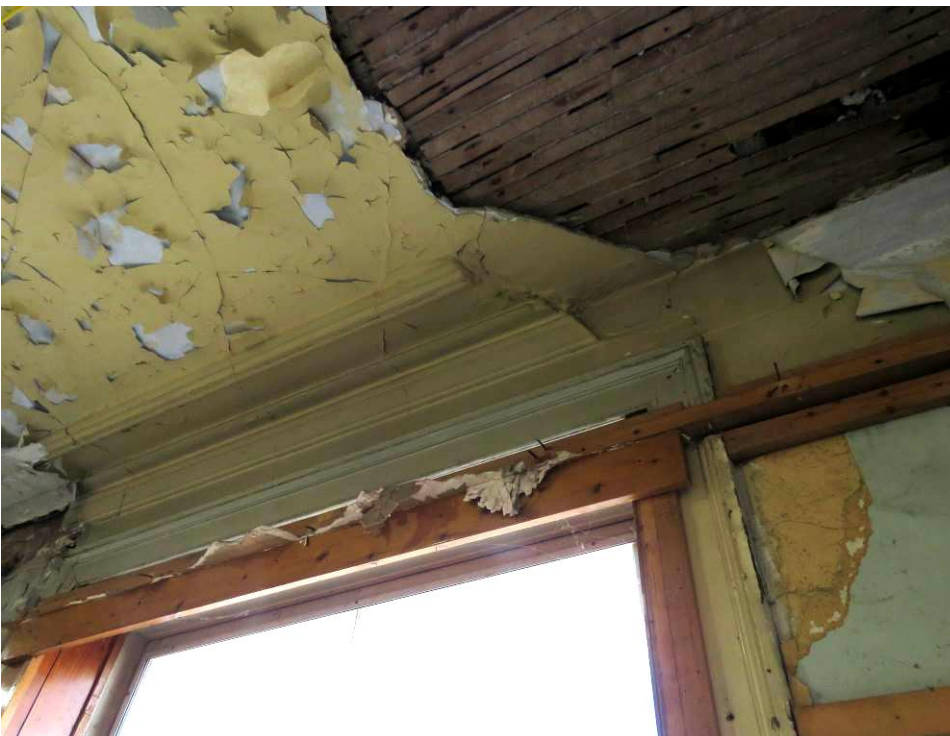
Figure 89 – An area of newly uncovered original moulded timber window surround and plaster cornice above one of the windows in 1F13.
