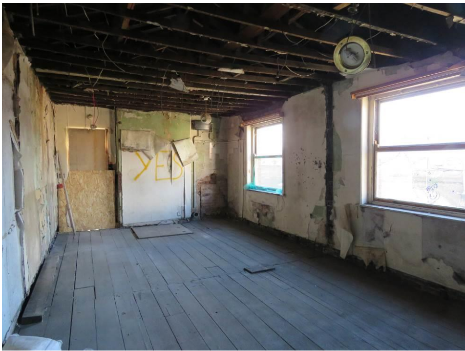
Figure 162 – Looking south through 2F010/11/12, showing removal of skirtings and lath and plaster ceiling.
