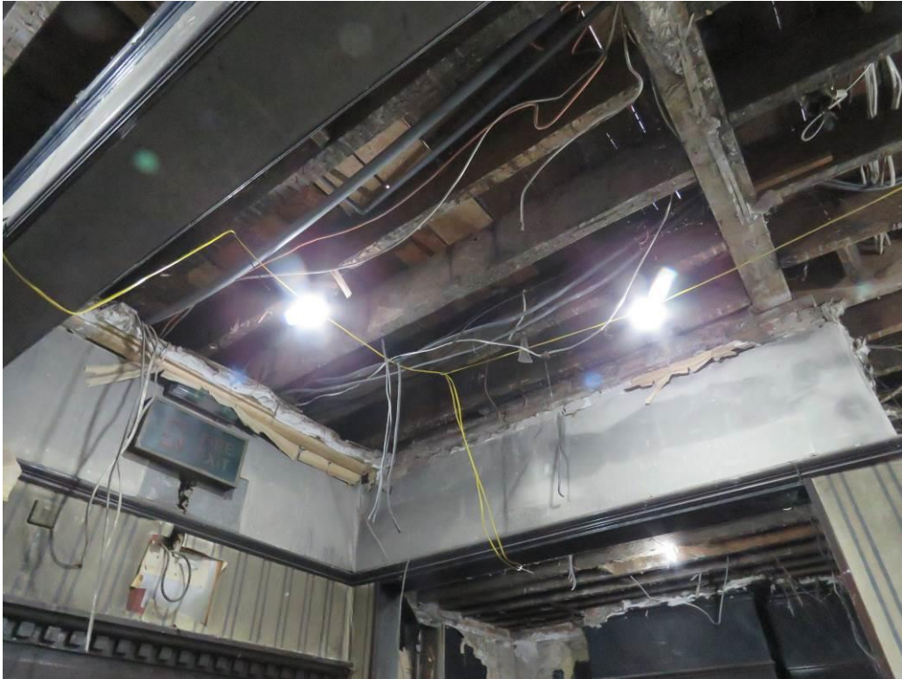
Figure 102 – Looking up at the removed lath and plaster ceiling and cornice to the entrance hall ceiling (GF3)
