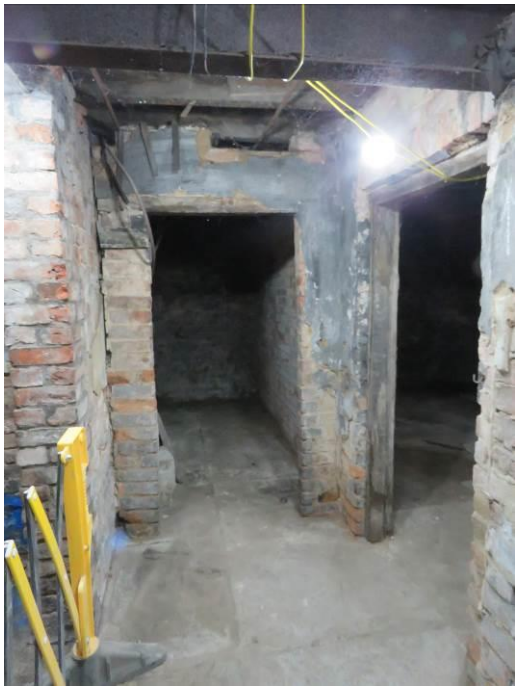
Figure 95 – Entrances into two of the rooms of No. 125.
