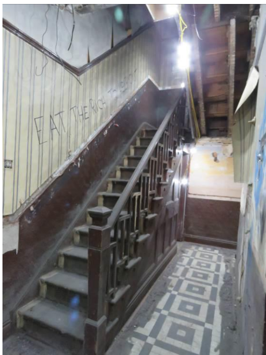
Figure 106 – Looking east towards the main staircase and hall corridor of GF3, showing the uncovered black and white tiled floor/ Note the removal of original ceiling/cornice.
