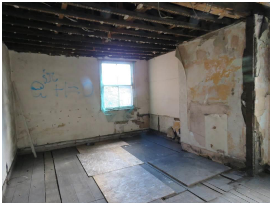
Figure 161 – 2F06, showing removal of lath and plaster ceiling and skirtings.
