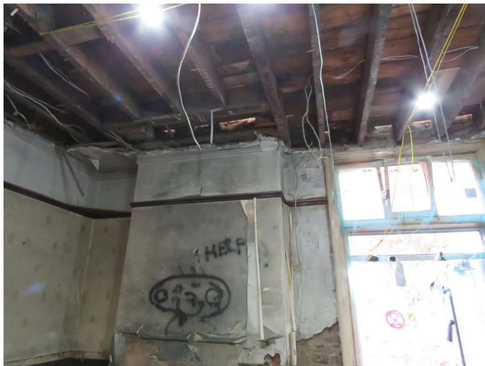
Figure 115 – The rear bar room (GF4) showing the removal of lath and plaster ceiling, cornice, and decorative plaster ceiling decoration.
