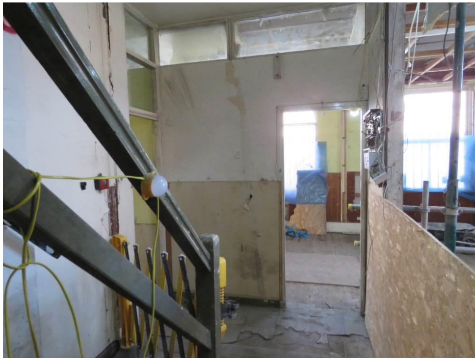
Figure 74 – Looking north through the former staircase hall (GF14).
