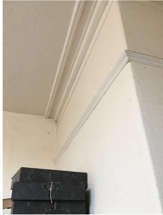
Figure 62 – A view showing the continuation of the same chimney breast as viewed from the western side of the partition. (1F01).
