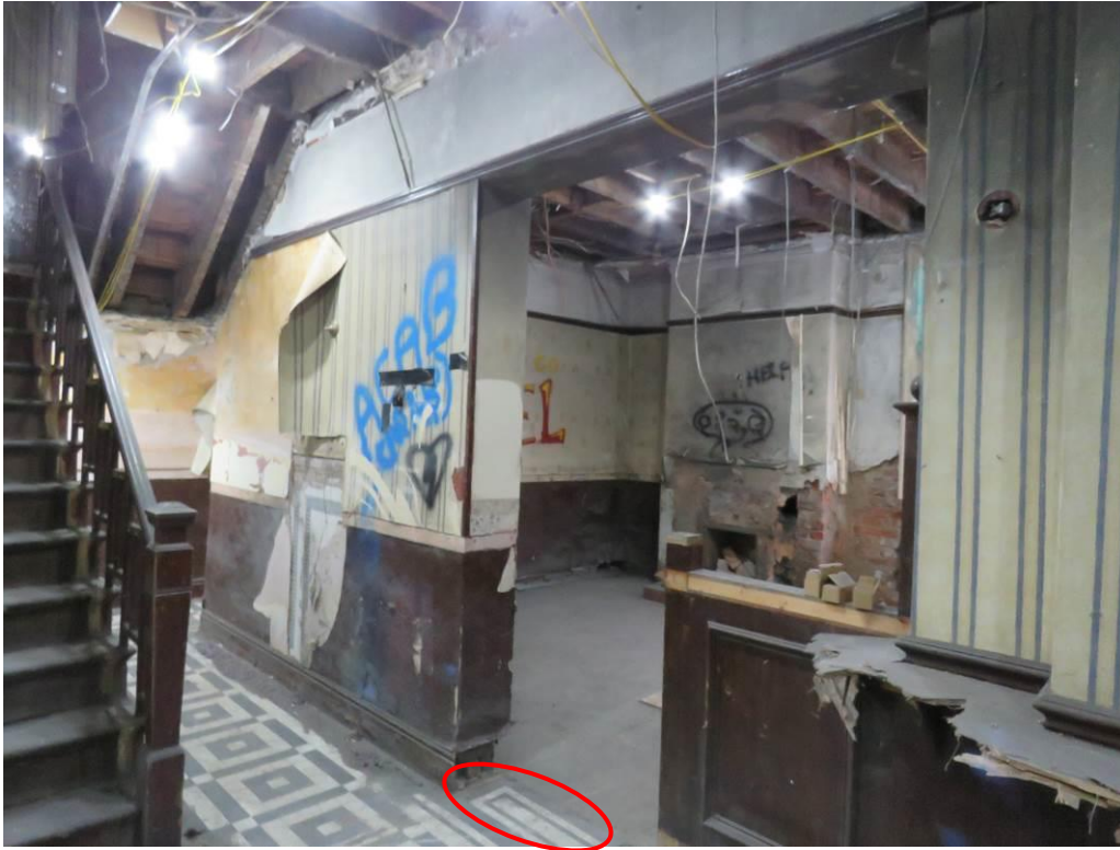
Figure 110 – The entrance hall and stairs (GF3) looking into GF4 (right). The original location of the door into GF4 can be seen in the uncovered floor tiles (circled).
