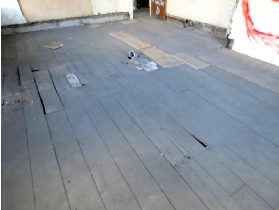
Figure 125 – Original, wide floorboard uncovered in 1F01 and 1F02. Note the removed skirting boards throughout.
