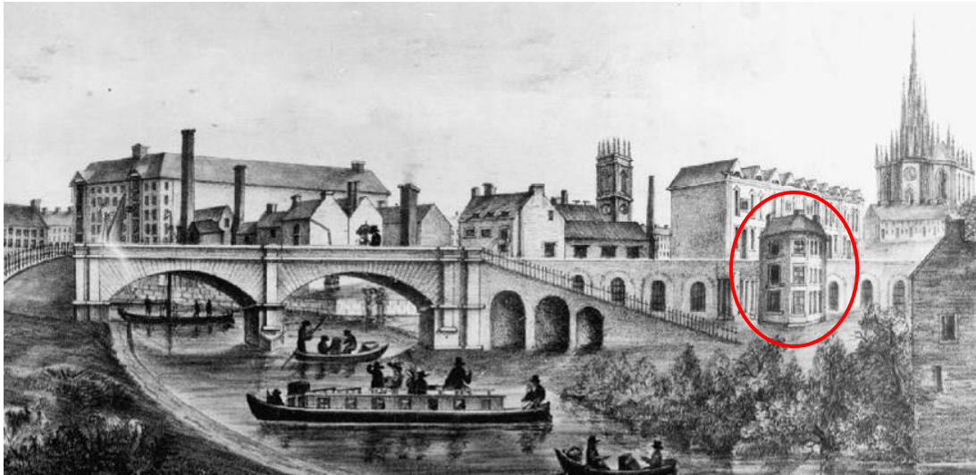
Figure 4 – An etching looking north across the River Irwell towards the newly completed bridge across Water Street in c1829. The former residential townhouse (circled red) marks the corner of Water Street and Liverpool Road. (Source Manchester Local Imaged Archive).
