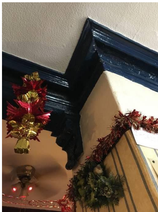
Figure 50 – The former chimney alcove to the corner bar to the west, showing the later removal of a wall and insertion of decorative corbel.(GF1)
