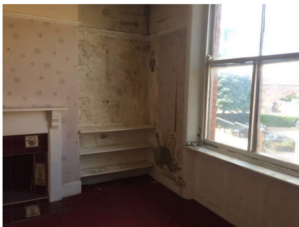
Figure 64b – The corner of the room (1F11), showing the Victorian fire surround and panelling.
