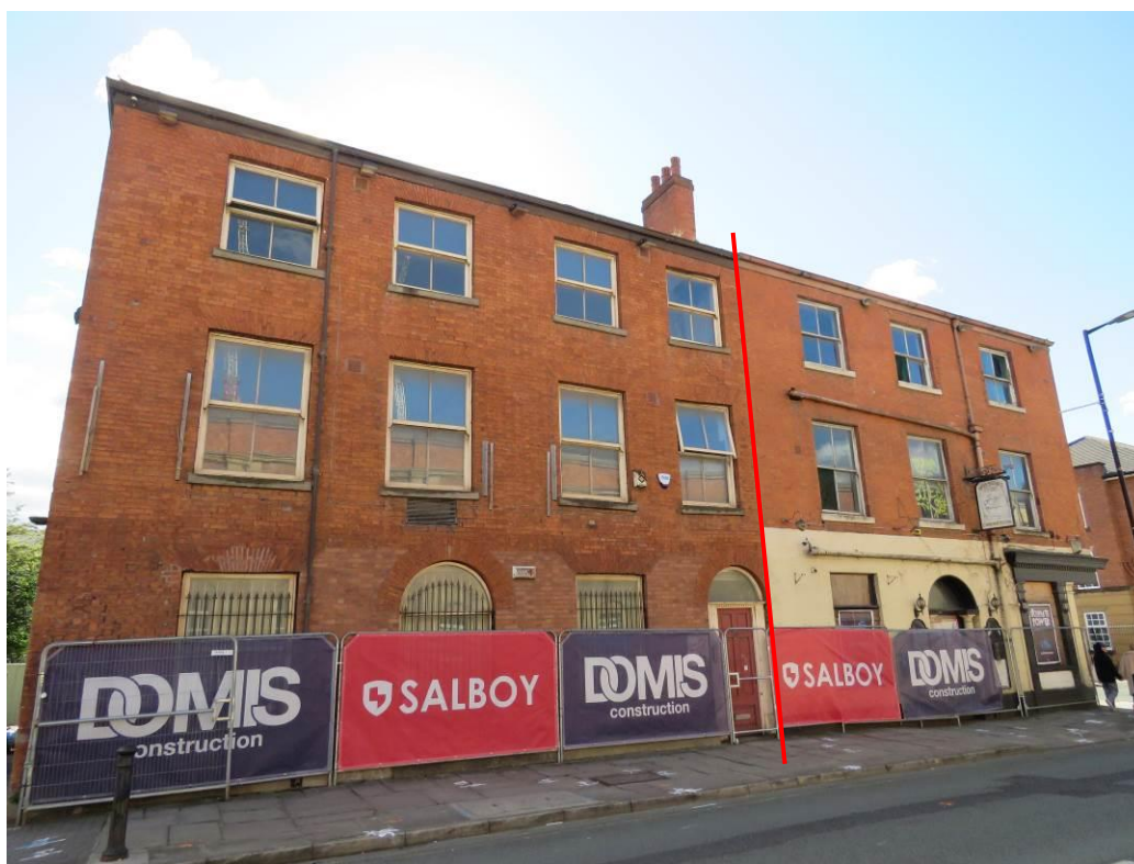
Figure 1 – No. 123 to the left (east) of the red line and No. 125 (the Commercial Hotel) to the right (west). (Source: SLHA Sept 2022)
