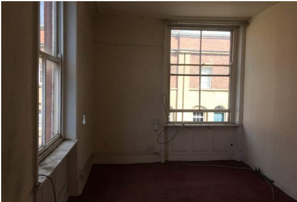
Figure 63 – Looking north into the former commercial room (1F01), showing the original timber panelling beneath the window. The wall on the right is a modern partition which divides the original room into two halves with the adjacent 1F02.
