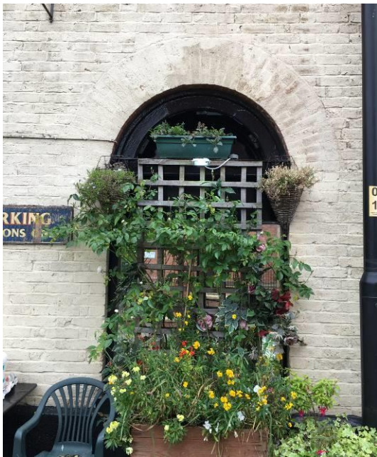
Figure 43 – The now blocked central entrance on Woollam Street (see Figures 8 & 9, which show the c1830 view of the hotel).
