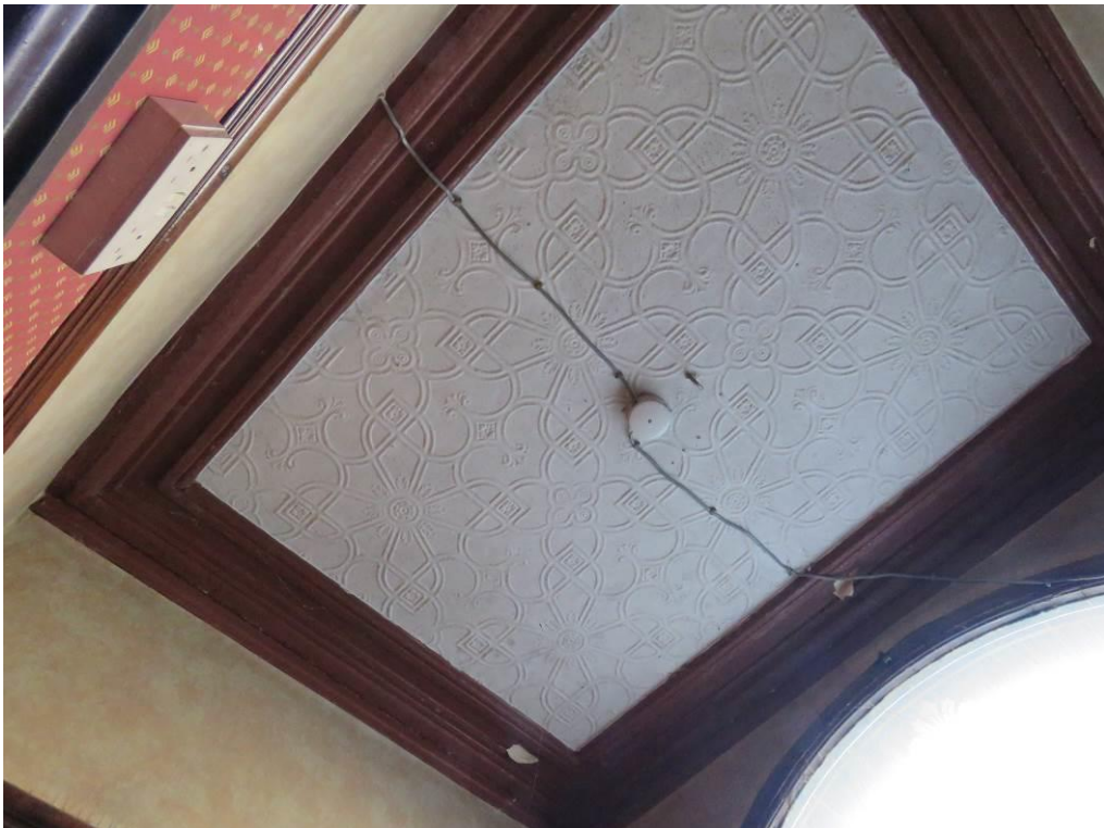
Figure 103 – The surviving original plaster cornice, lath and plaster ceiling and decorative ceiling paper found complete in the entrance vestibule (GF1A).
