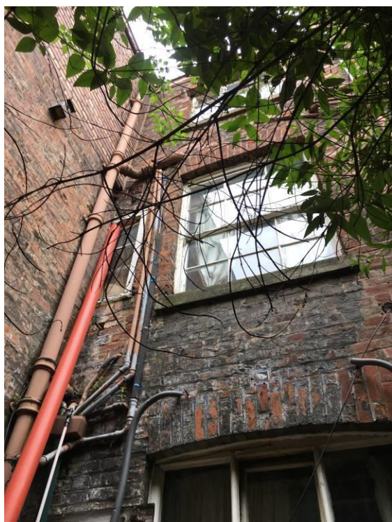
Figure 45 – The rear (south) elevation as seen from the central courtyard space. The structure to the left forms the rear of the 1836 extension.
