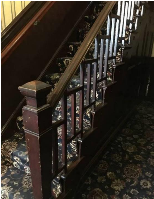
Figure 52 – The altered c1890s-1900s staircase (GF3).
