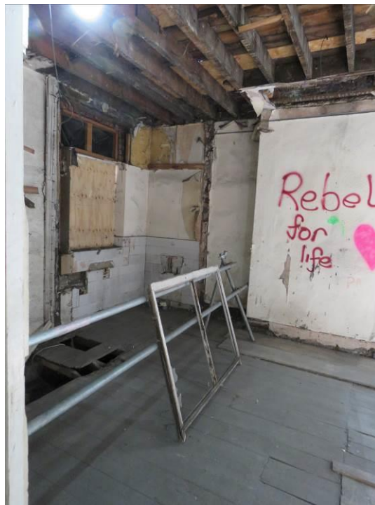
Figure 135 – Looking into 1F06, showing the original location of the now removed partition (with consent) which enclosed the original link corridor (1F05) to the coach house/stables from the landing (1F04).
