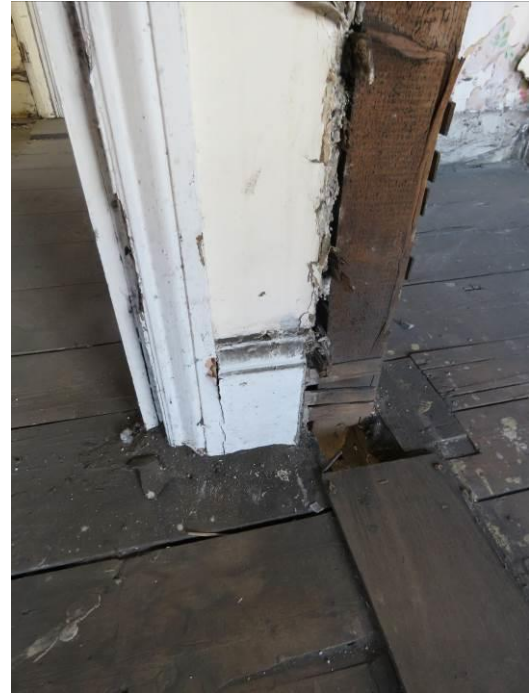
Figure 151 – Small surviving piece of skirting to the corner between 2F03 (left) and 2F02 (right)
