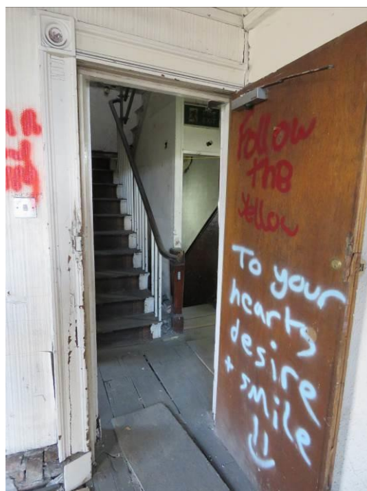
Figure 129 – The original decorative architrave surrounding the door into 1F02 from the landing.
