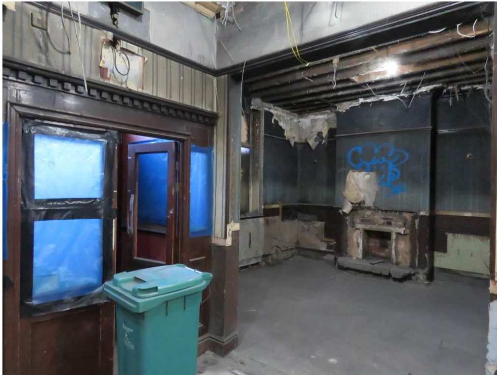
Figure 101 – Looking east from the original entrance hall (GF3) into the adjacent bar room (GF2) which can be seen to have had its original lath and plaster ceiling and cornice removed. The modern doors to the left lead into the entrance vestibule (GF1A).
