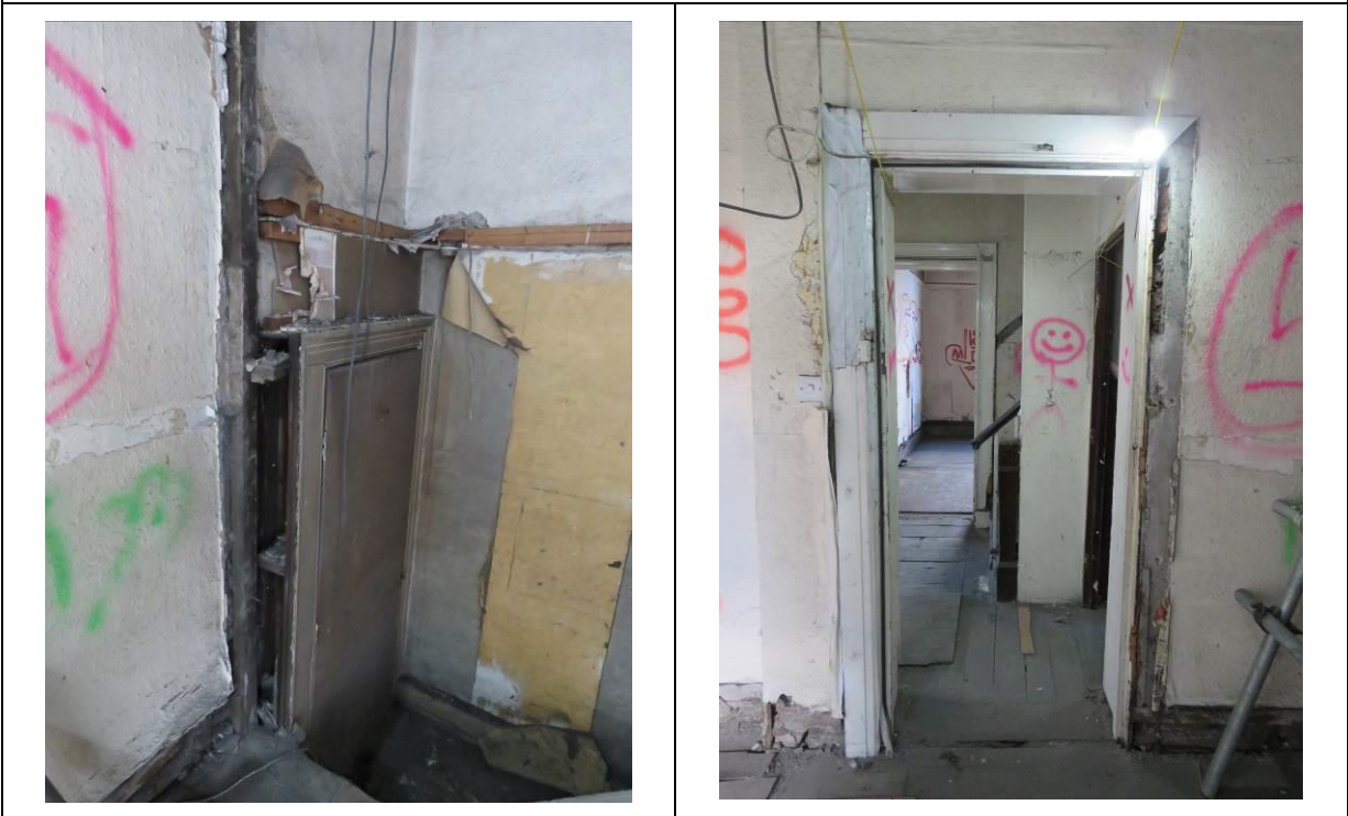
Figure 138 – Looking down into the lower level of the former link corridor (1F05).
