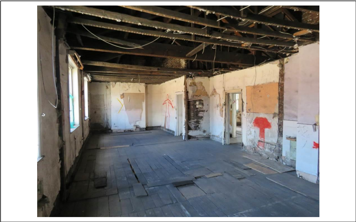
Figure 156 – Looking east from 2F01, through 2F02 and into 2F03.
