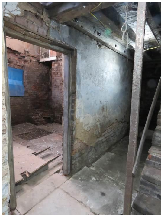
Figure 97 – Looking south towards the basement room beneath GF13 adjacent to the original stairs of No. 125.
