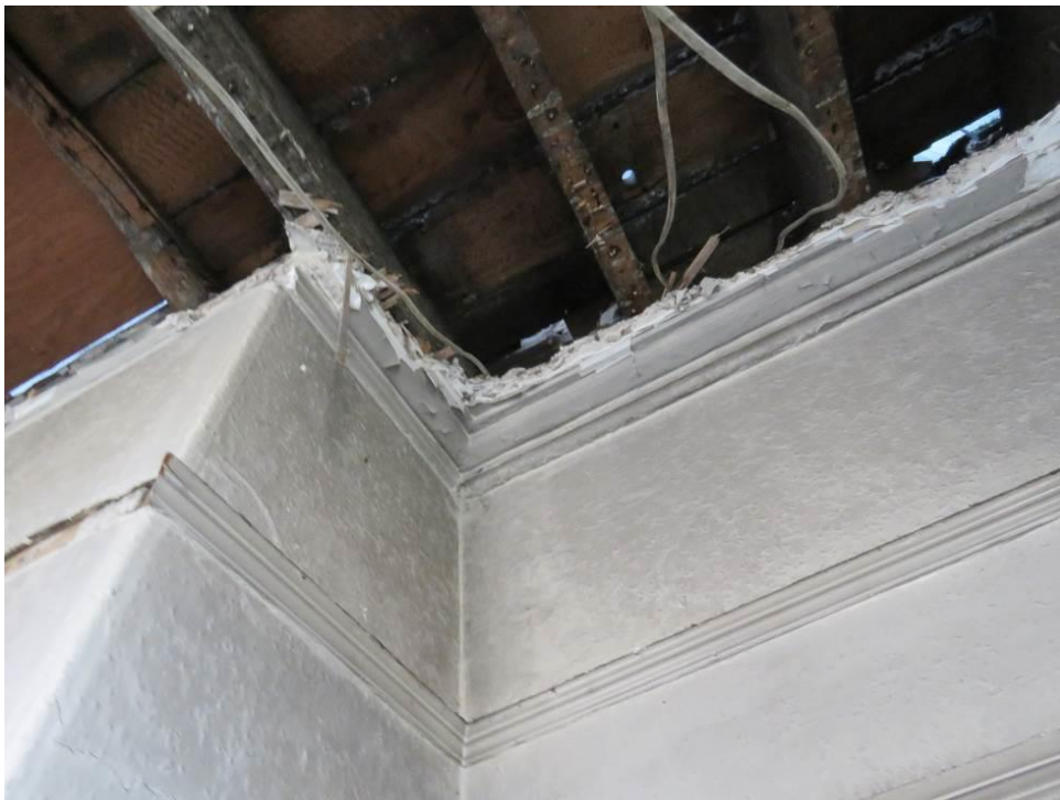
Figure 126 – An area of partially surviving cornice to the alcove of 1F01, and small area of removed picture rail.
