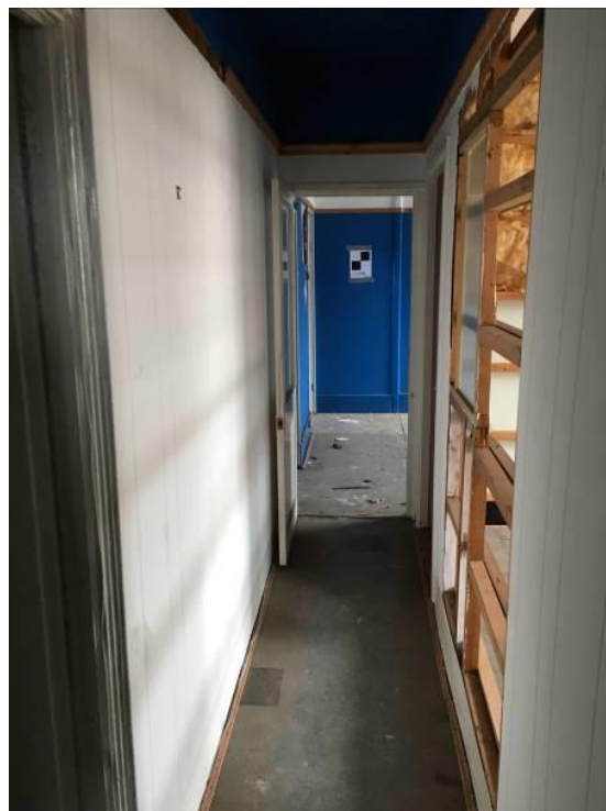
Figure 34 – A view looking across the now combined dwellings (south of 1F13).
