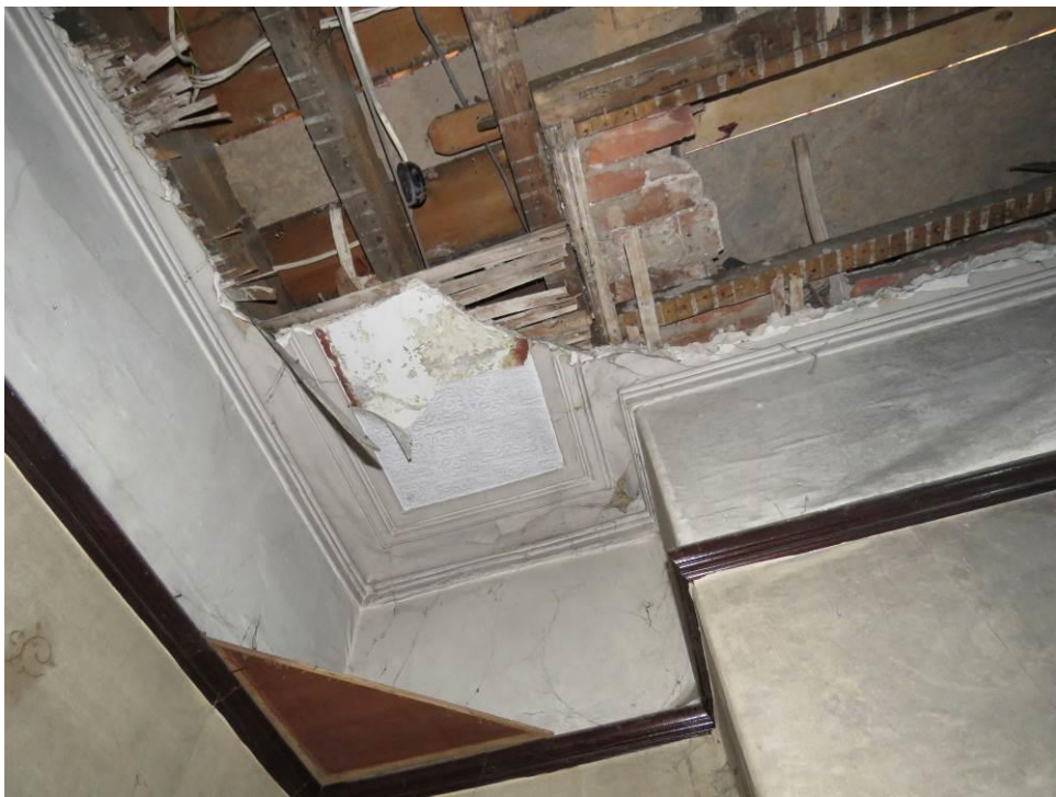
Figure 116 – A detailed view of a small area of surviving plaster cornice to the alcove of GF4.
