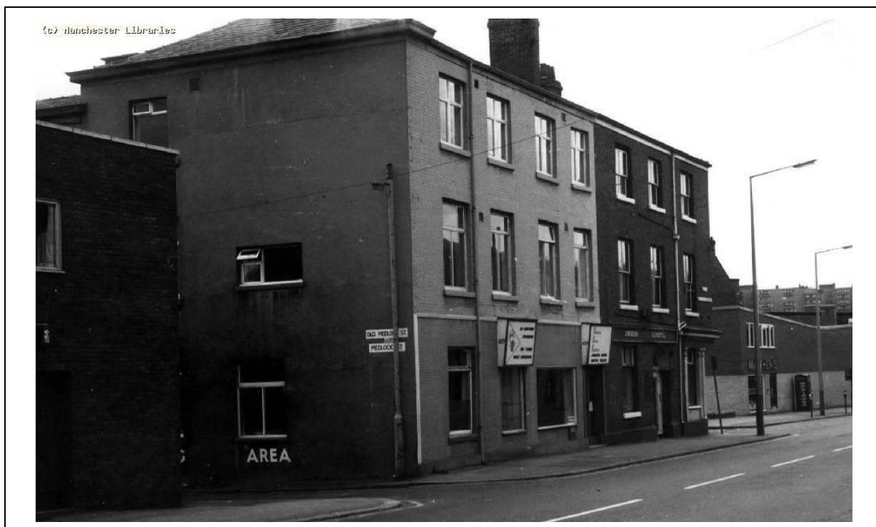
Figure 19 – Looking westerly along Liverpool Road at its junction with Medlock Street (then renamed Old Medlock Street) in 1972. This image shows the modern render coating applied over the front and side elevations of No. 123, along with the insertion of a new window openings on the east and north elevations, and all windows being replaced with casements. (Source Manchester Local Imaged Archive).
