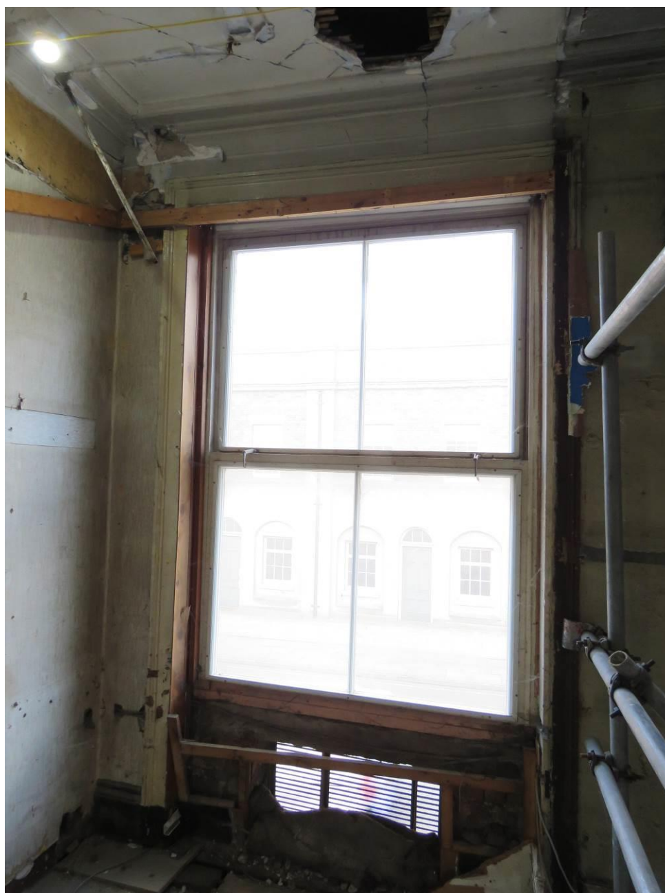
Figure 90a – A length of newly uncovered original moulded timber window surround and plaster cornice above one of the windows in 1F13.
