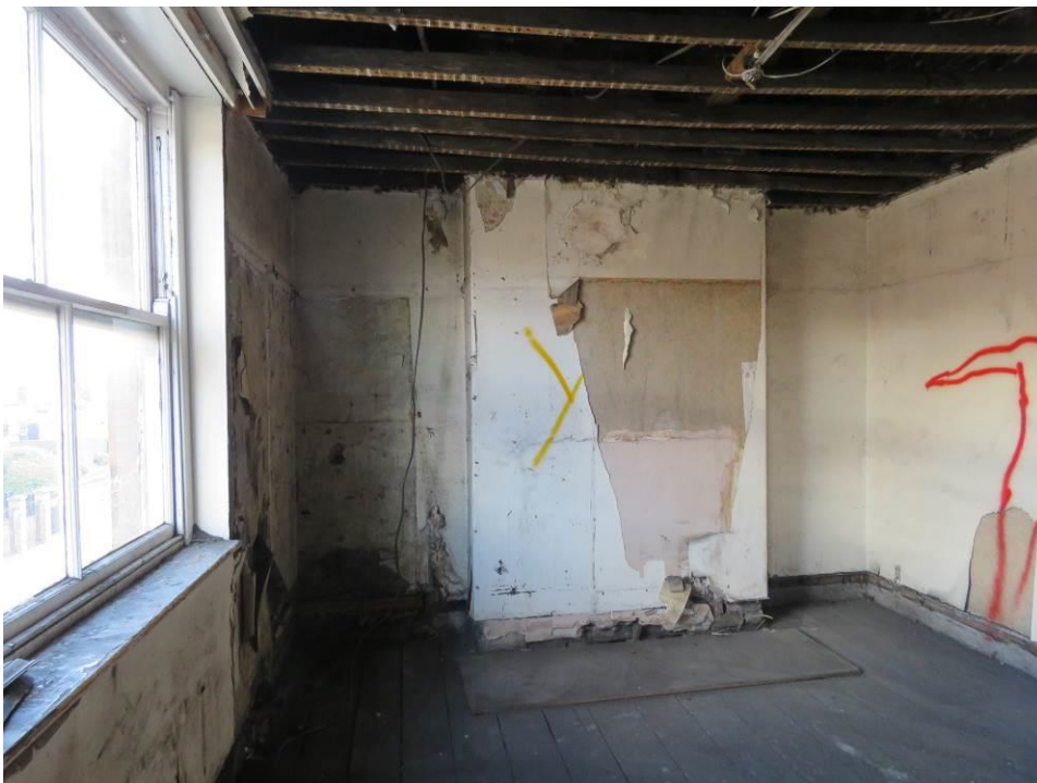
Figure 147 – Looking east across 2F03 showing the removal of skirtings and lath and plaster ceiling.
