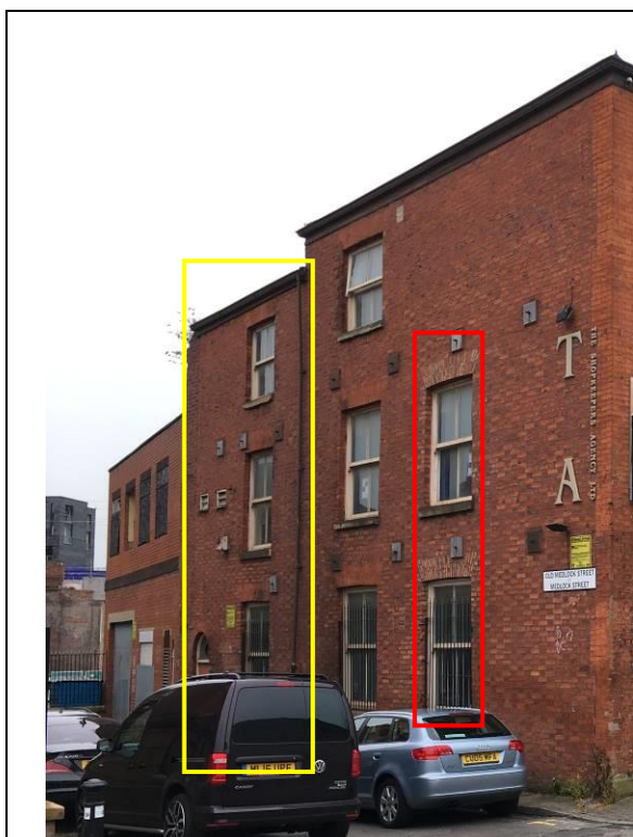
Figure 24 – The east elevation on Old Medlock Street, showing the side aspect of No. 121 to the right with inserted windows outlined in red, and the
