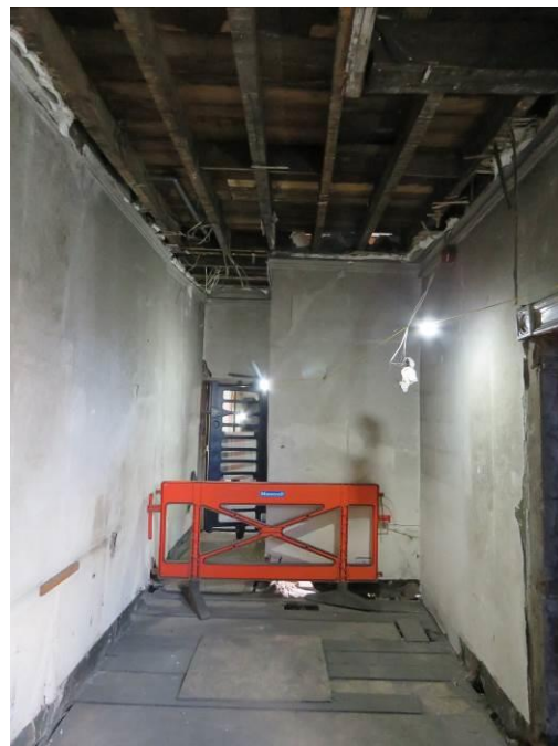
Figure 141 – Looking east along corridor 1F08, showing the removal of original lath and plaster ceiling, cornice and skirtings.
