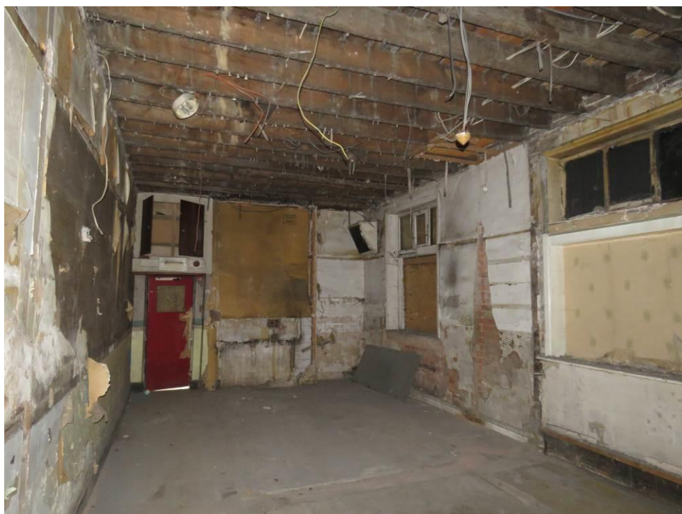
Figure 118 – Looking south through GF6/7 and 8, showing the removal of all modern partitions.
