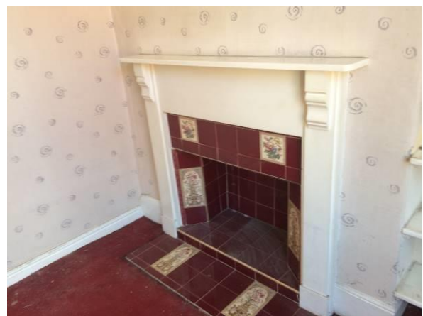
Figure 64c – The Victorian fire surround, showing the inserted modern partition wall to the left (1F11).
