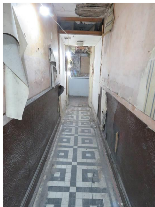
Figure 109 – Looking south into the second half of the dog-leg corridor of GF3.
