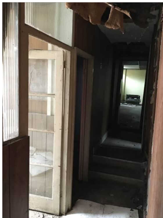
Figure 36 – Looking through the adjoining property.
