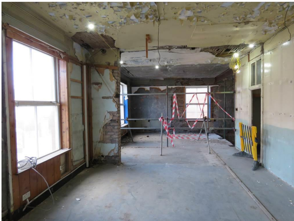
Figure 86 - Looking east from 1F12 through 1F13 into 1F14.
