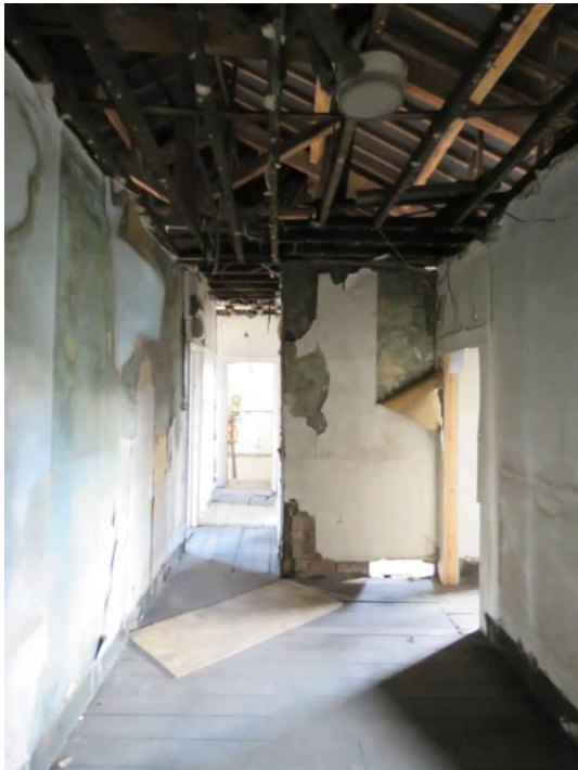
Figure 159 – 2F05 looking east, showing removal of skirtings and ceiling.
