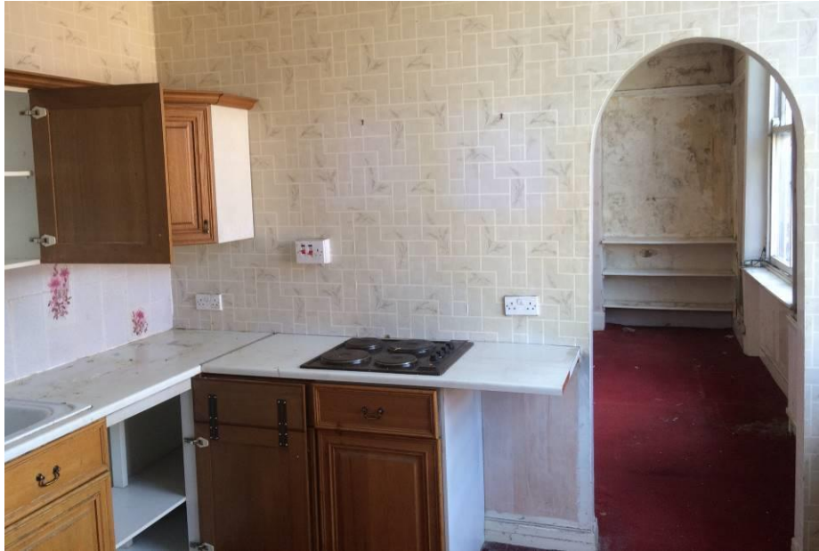
Figure 64a – Looking south from 1F10 into 1F11 which was originally one large room probably used as a commercial room or sitting room for guests. Beneath the two sash windows to the right is similar timber panelling as found in the neighbouring rooms 1F01 and 1F02.
