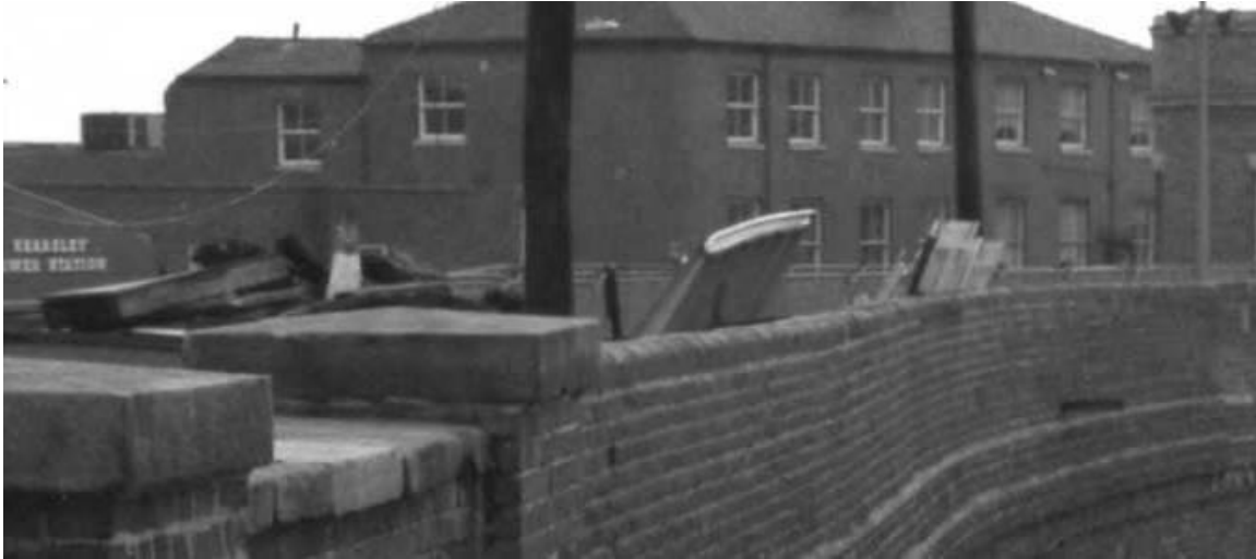
Figure 21 – A view looking in a southerly direction towards the front (north) elevation of the Site from the Liverpool Road Station site in 1992. This image shows that by 1992 No. 123 has had its render removed and brickwork restored, including replacement casements in the style of sash windows. (Source Manchester Local Imaged Archive).
