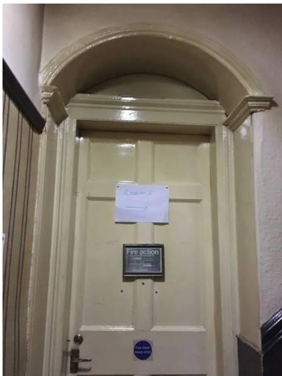
Figure 55 – The mid-landing doorway which originally led up into a link corridor connected to the first floor level of the now demolished rear stables/coach house building. Now a foreshortened cupboard (1F05).
