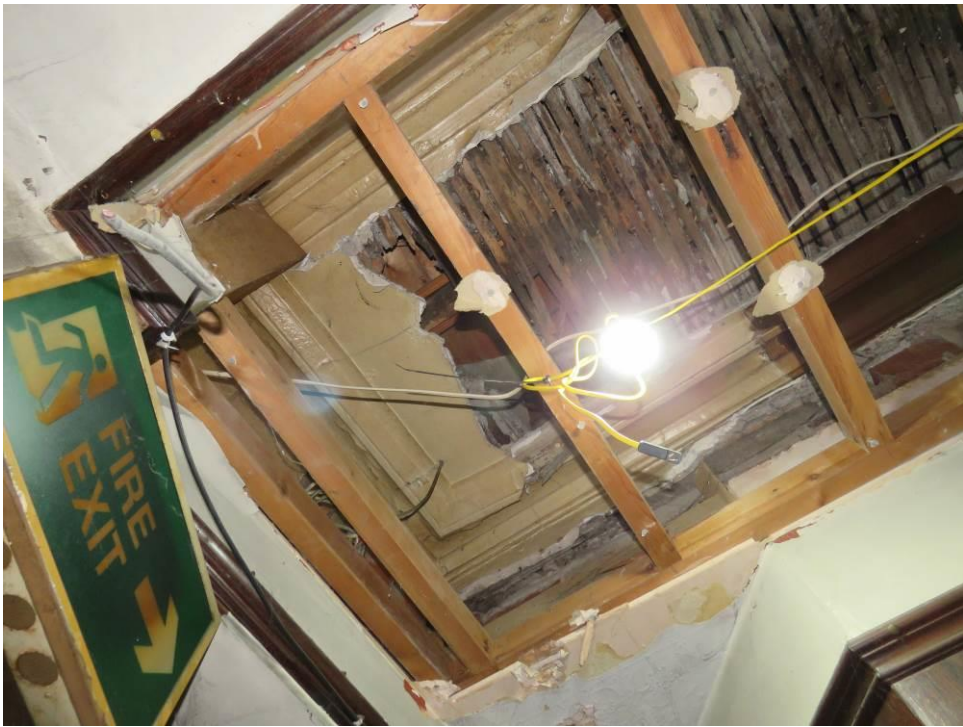
Figure 117 – Looking up at the ceiling of GF5, showing an area of surviving laths, lath and plaster and cornice,
