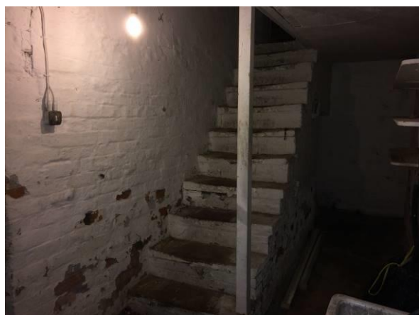
Figure 69 – The original stone and brick basement steps.
