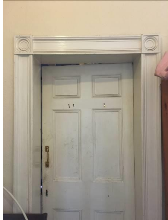
Figure 58 – An original six-panelled door and distinctive architrave with circular corner blocks on the first floor corridor (1F07) leading into 1F08.
