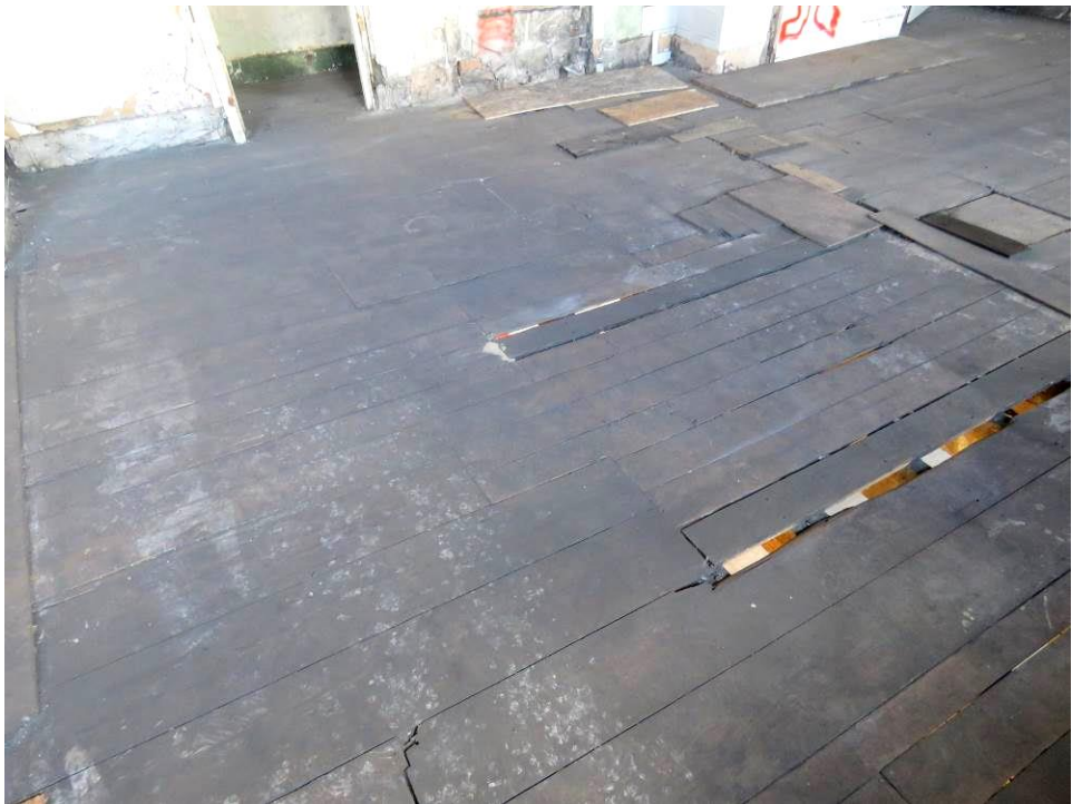
Figure 155 – The now exposed original and early floorboards to 2F02.
