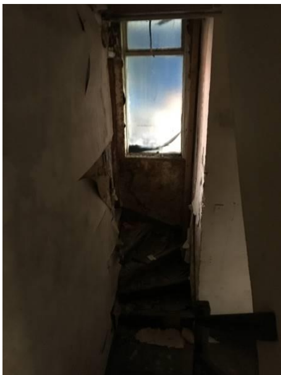
Figure 35 – The first floor landing of No. 123, showing the later inserted steps into the first floor level of the building.
