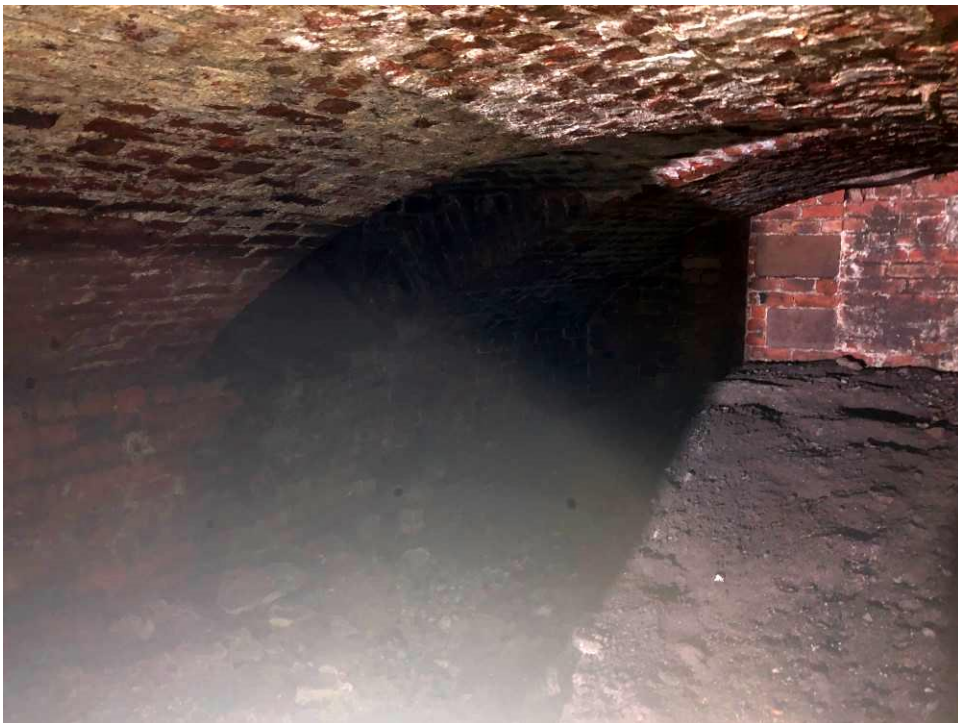
Figure 84 – A view further east into one of the newly discovered subterranean chambers beneath the 1950s/60s building.
