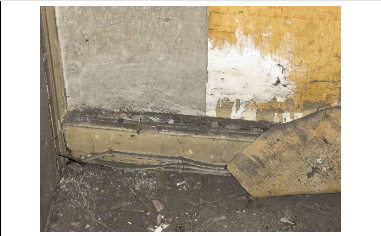
Figure 137 – A surviving area of original skirting to the former link corridor (1F05).
