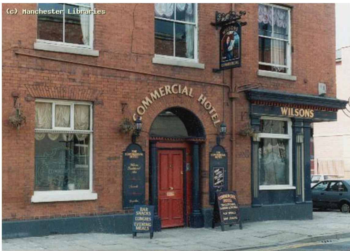
Figure 22 – The same view as seen in 1994, showing the reintroduction of two new timber columns and a more appropriately designed timber panelled door.
