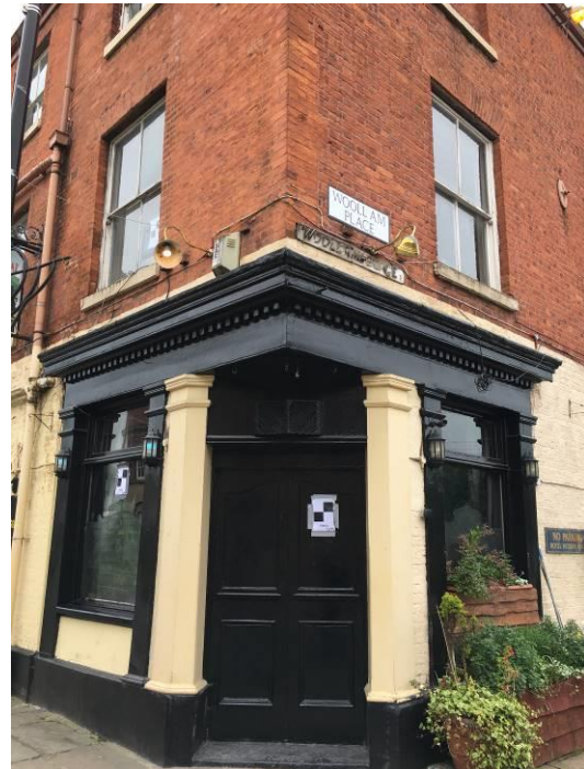
Figure 41 – The c1890s inserted corner entrance and bar shop fronts on the corner of Woollam Place.
