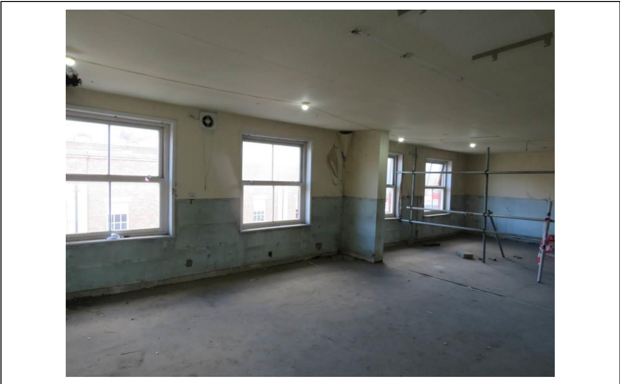
Figure 92 – Looking along the north elevation of the second floor (2F14).
