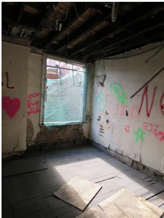
Figure 134 – Looking into 1F06, showing removal of skirtings, a largely destroyed sash window, and consented removal of ceiling.
