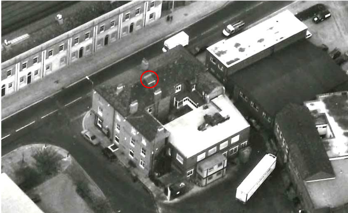
Figure 17 – Aerial view looking north over the Site in the early 1980s, showing the large c1950s/60s block on the site of the original stables/coach house. Note the skylight over the main staircase of the Commercial Inn (circled). (Source Manchester Local Image Archive).
