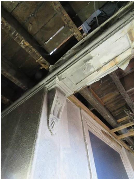
Figure 144 – The original surviving plaster corbel to corridor 1F07.
