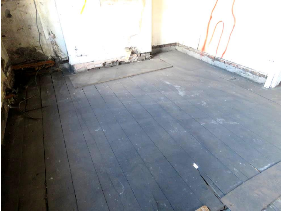
Figure 148 – The now exposed original wide floorboards in 2F03.
