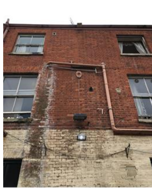
Figure 44 – The vertical joint between the c1829 hotel to the left, and the c1836 extension to the right. (see Figures 8 & 9, which show the c1830 view of the hotel).
