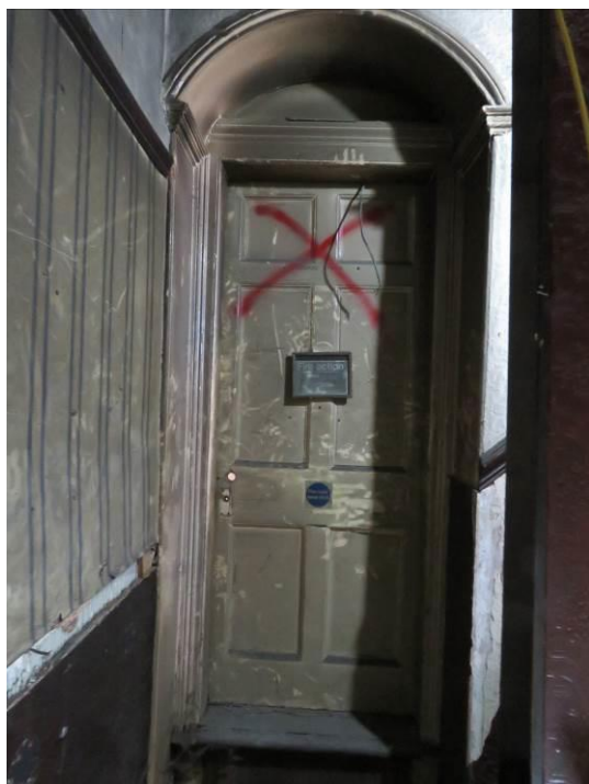
Figure 119 – The mid-landing (1F04) looking towards an original surviving panelled door to 1F05, which formed the original link corridor to the coach house/stables.
