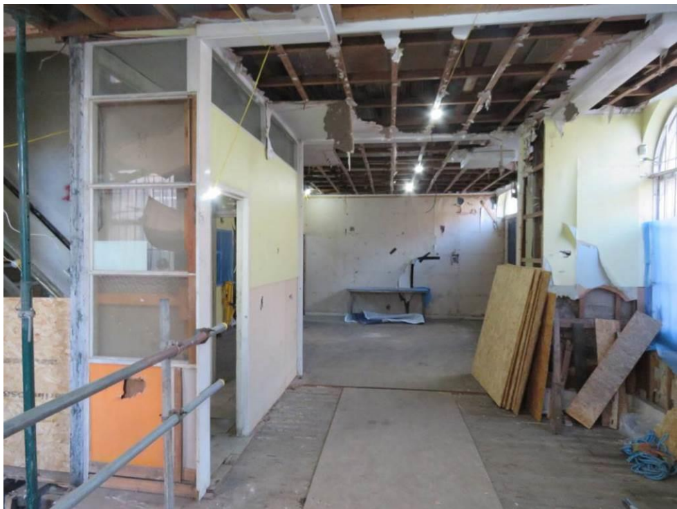
Figure 75 – Looking west across GF13.
