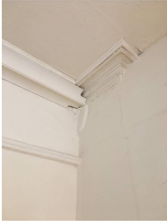
Figure 61 – A section of original plaster cornice around the chimney breast of the former commercial room, which is now largely concealed by a modern partition dividing the room into two, as viewed from the eastern side of the partition (1F02).
