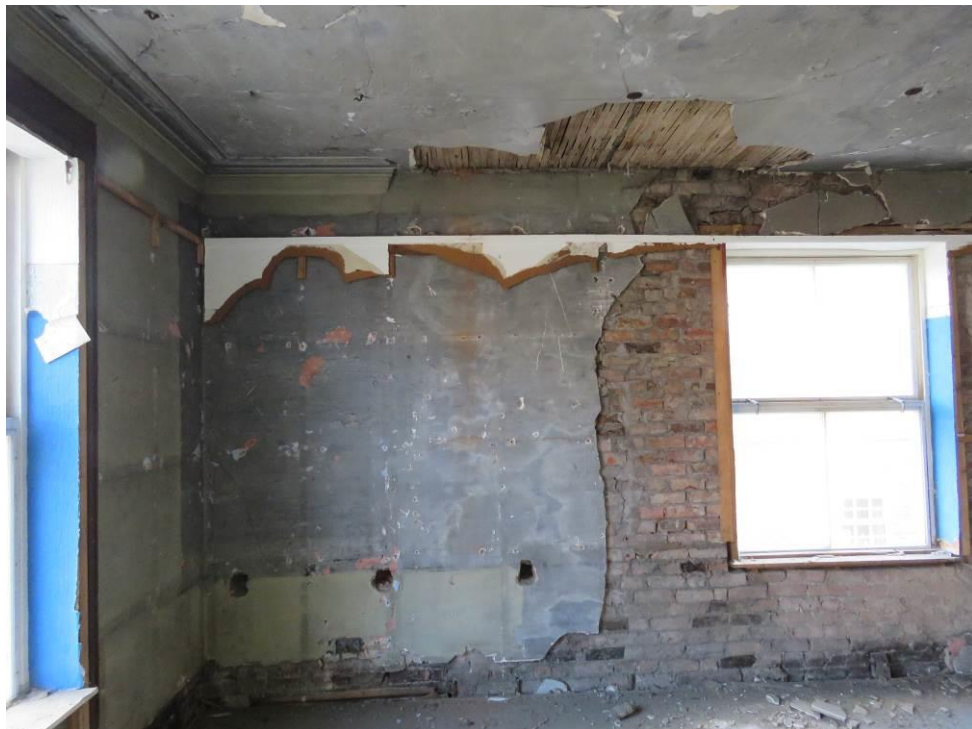
Figure 91 – Looking along the east elevation of 1F14, showing the area of cornice.
