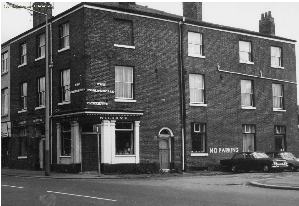
Figure 18 - The west elevation on Woollam Place in 1972. (Source Manchester Local Image Archive).
