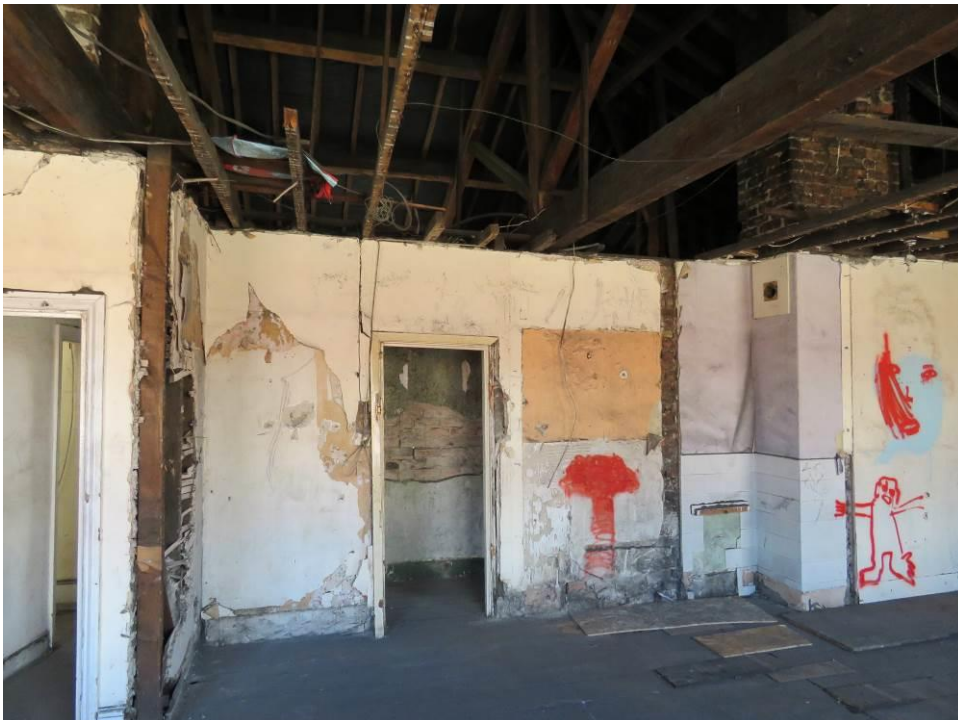
Figure 149 – Looking south through 2F02 showing the removal of lath and plaster ceilings and area of ceiling structure.
