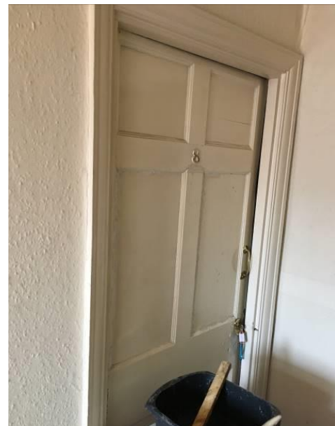
Figure 68 – An early six-panelled door located in the c1836 extension (2F10), which has been relocated
