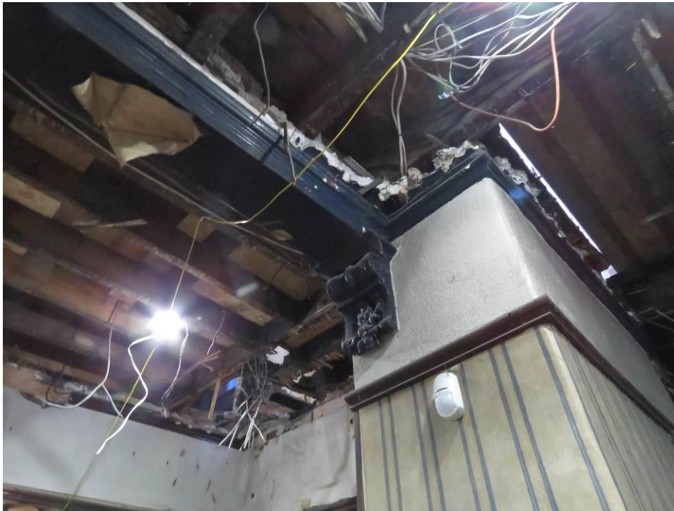
Figure 113 – The surviving decorative plaster corbel between GF1 (right) and GF5 (left).
