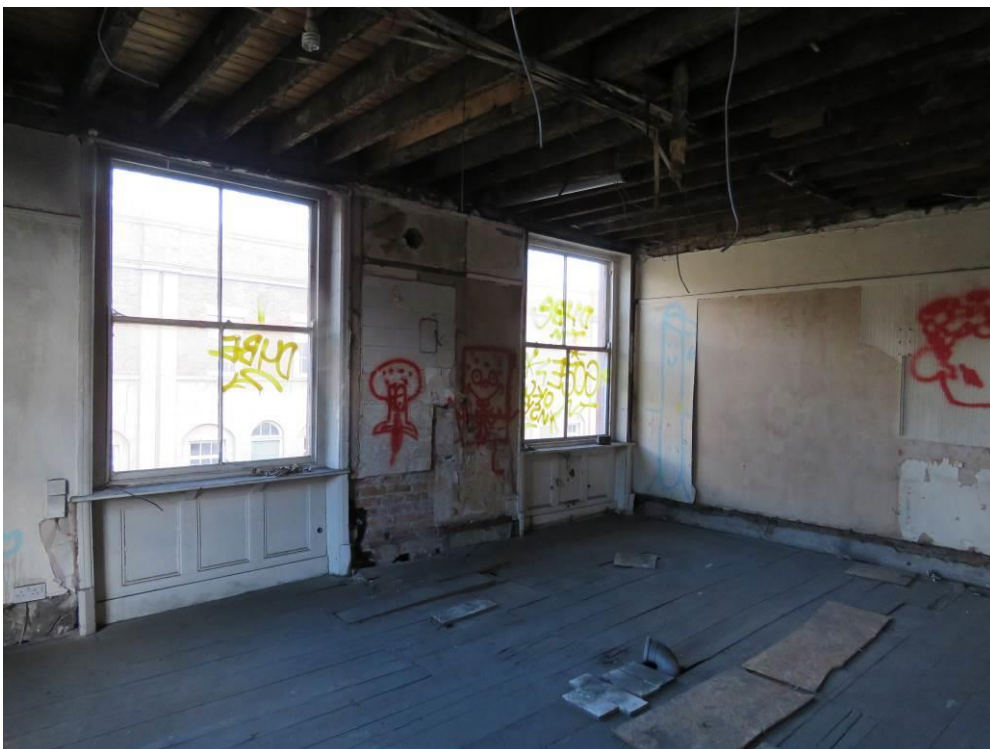
Figure 124 – Looking north-east across the two former rooms of 1F01 (left) and 1F02 (right) which can now be seen in its original proportions, showing the consented removal of modern partitions and bathrooms. Note the removal of original skirting boards.
