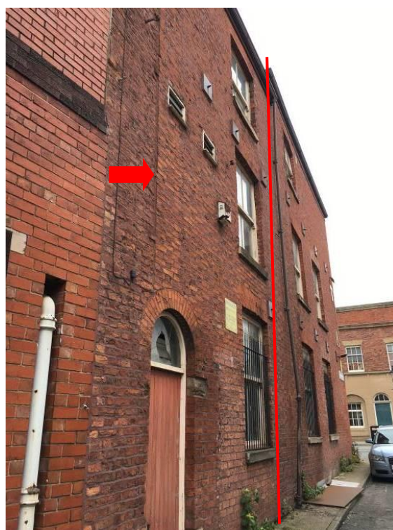
Figure 25 – Looking north along Old Medlock Street showing the neighbouring former dwelling to the left, with original entrance into side alley.
