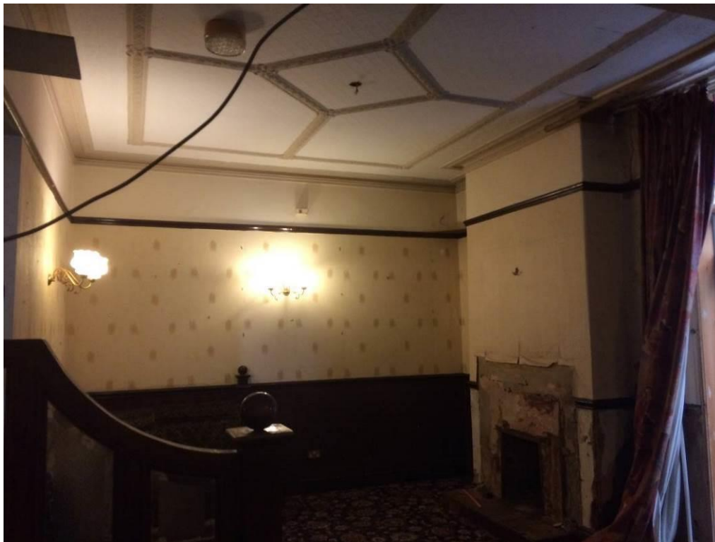
Figure 54 – The rear (south) reception room (GF4), showing the original plaster cornice and 19 th century
