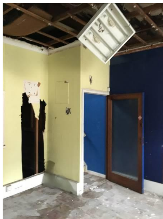
Figure 28 – The location of the original staircase to No. 123 (GF12).
