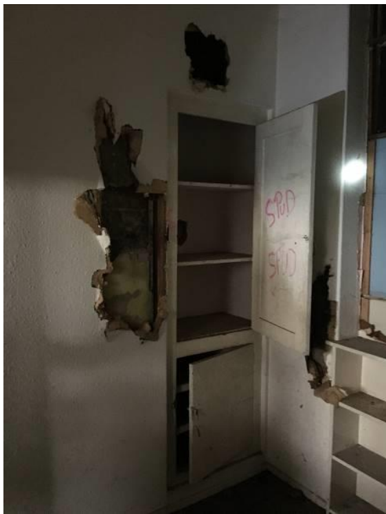
Figure 31 – The surviving original, hand made,
