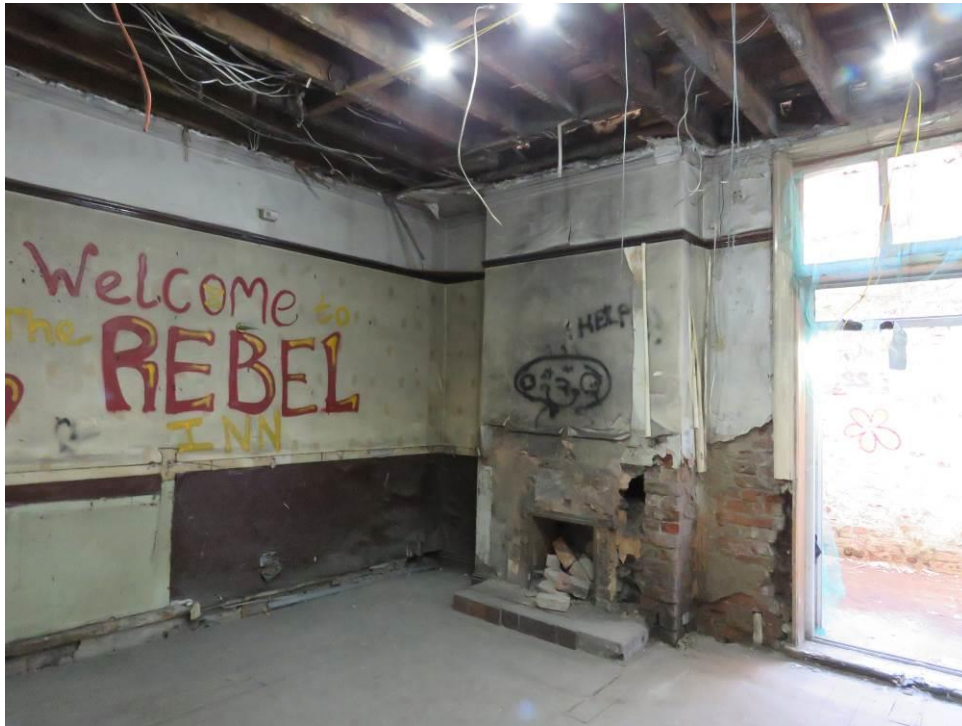
Figure 114 – Looking into the rear bar room (GF4), showing the removal of lath and plaster ceiling, cornice, and decorative plaster ceiling decoration.
