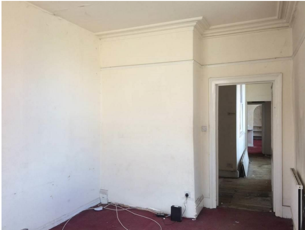
Figure 64 – Looking south across the former commercial room (1F01), showing the original chimney breast and doorway. The wall on the left is a modern partition which divides the original room into two halves with 1F02.
