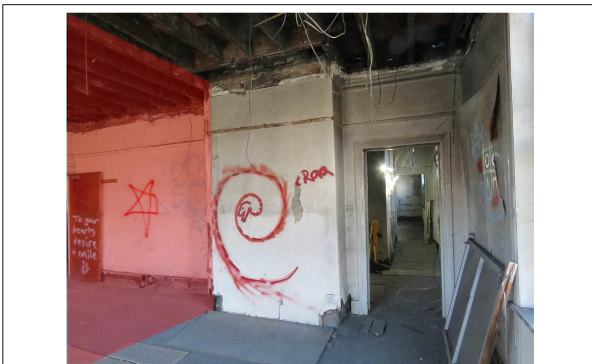
Figure 127 – Looking south through 1F01, showing the now removed modern partition (shaded red) that divided this room from 1F02. Note the removed original lath and plaster ceiling, cornice, original panelled door to the opening (right) and skirtings.
