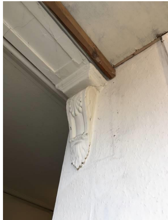
Figure 60 – The c1836 plaster corbel inserted into the new link corridor to the rear extension 1F07.
