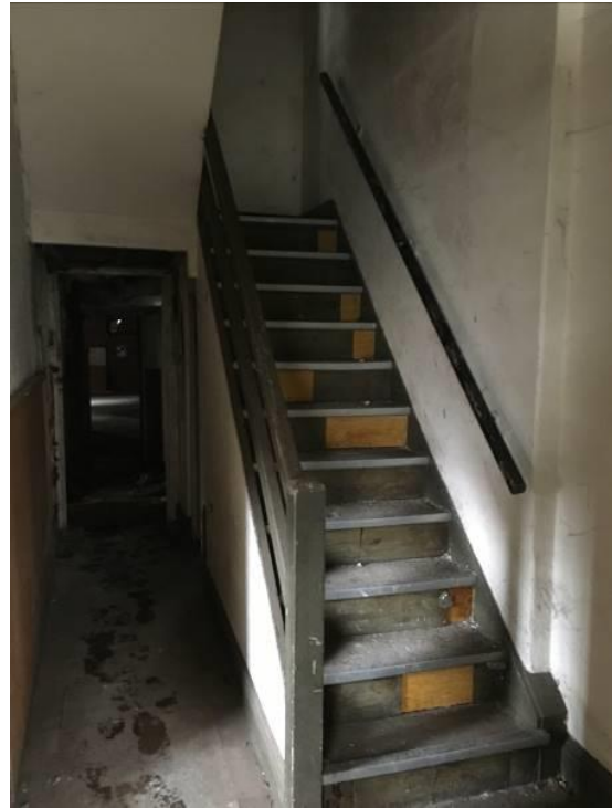
Figure 30 – The modern staircase inserted in the location of the original example at what was No. 121 (GF14).
