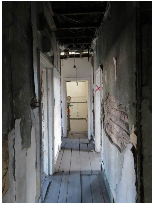
Figure 160 – 2F05 looking east, showing removal of skirtings and ceiling.
