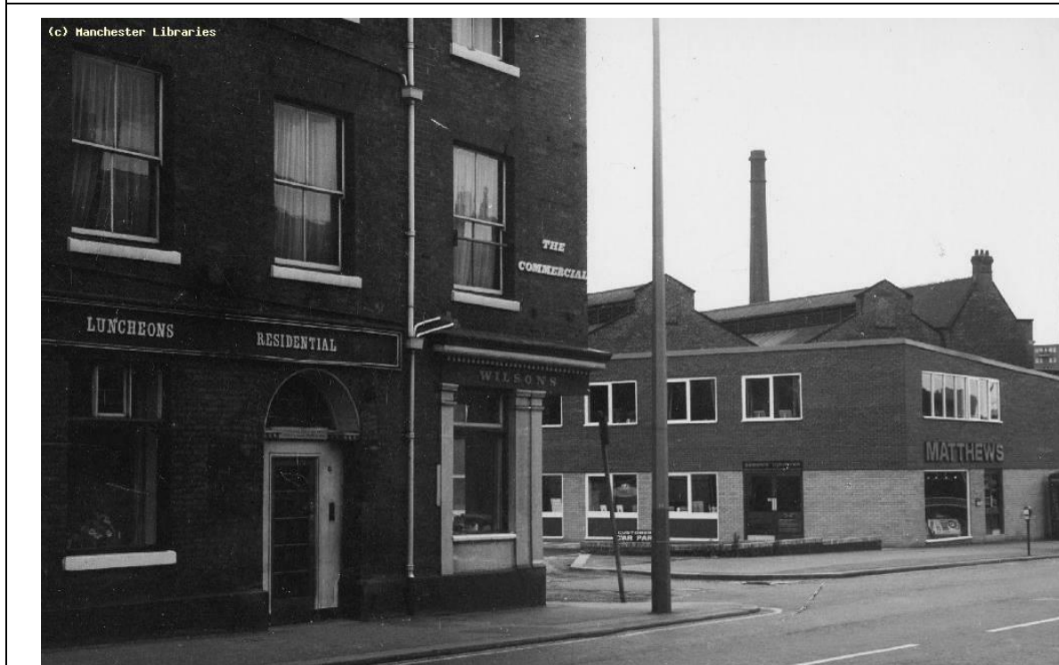
Figure 20 – The corner of the Commercial Hotel in 1972, showing the insertion of a new glazed door and the removal of the original timber columns either side. (Source Manchester Local Imaged Archive).
