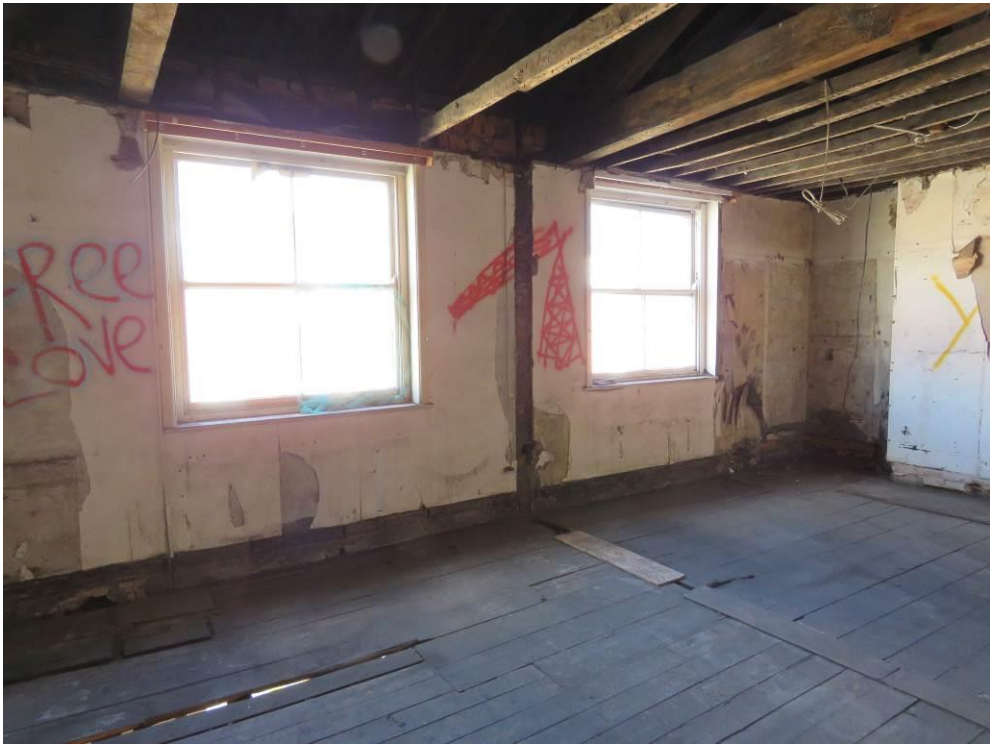
Figure 154 – Looking north-east from 2F02 into 2F03.
