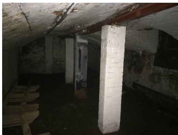
Figure 70 – Looking south into the barrel-vaulted basement room.
