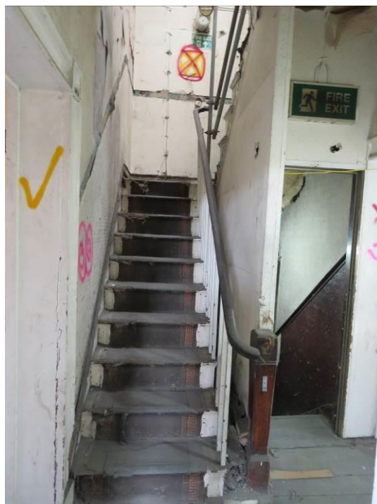
Figure 120 – The first floor landing (1F04).
