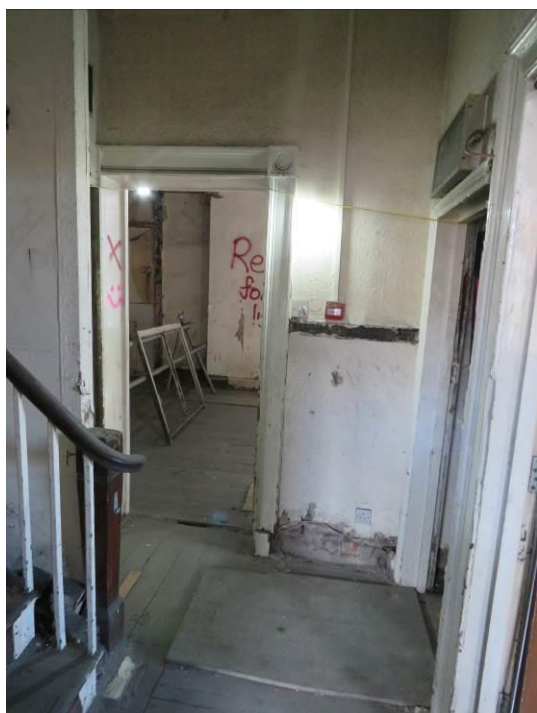
Figure 121 – Looking south across the landing, showing the removal of original skirting boards.
