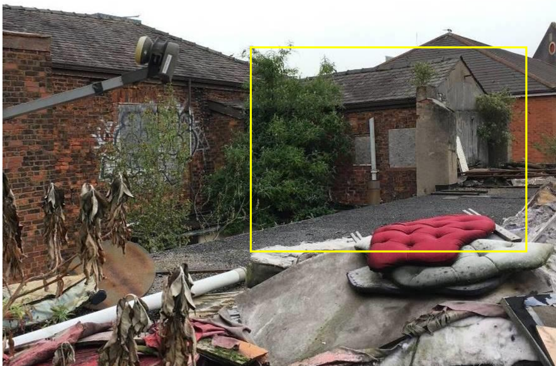
Figure 26 – The rear (south) elevation of the building, showing the rear of the east return along Old Medlock Street to the right (outlined yellow). The areas of grey render mark the remains of the original c1829 coach house and stables.
