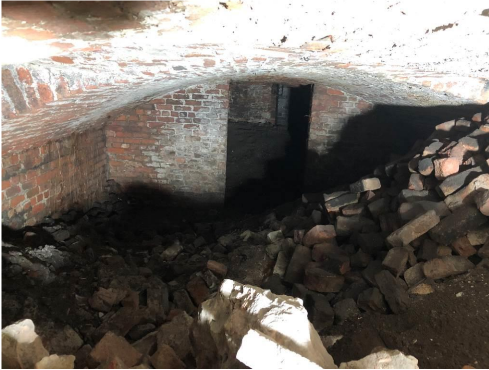
Figure 83 – A view looking east into one of the newly discovered subterranean chambers beneath the 1950s/60s building, which originally formed part of the basement of the original coach house and stables.
