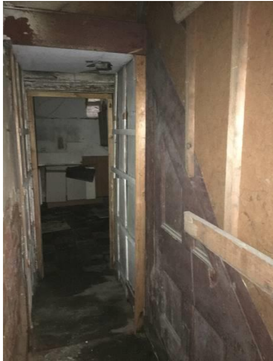
Figure 29 – The surviving original timber panelling to the side of the staircase in No. 123 (GF12). Note the original access to the basement beside the panelling is blocked.
