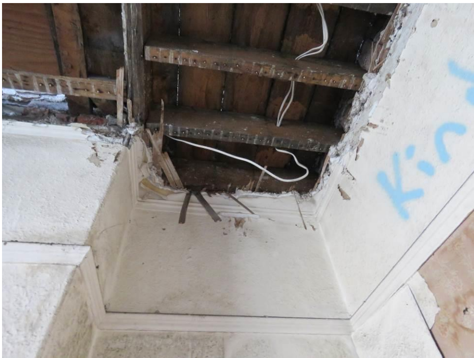
Figure 132 – A small surviving area of damaged cornice to the alcove of 1F03.
