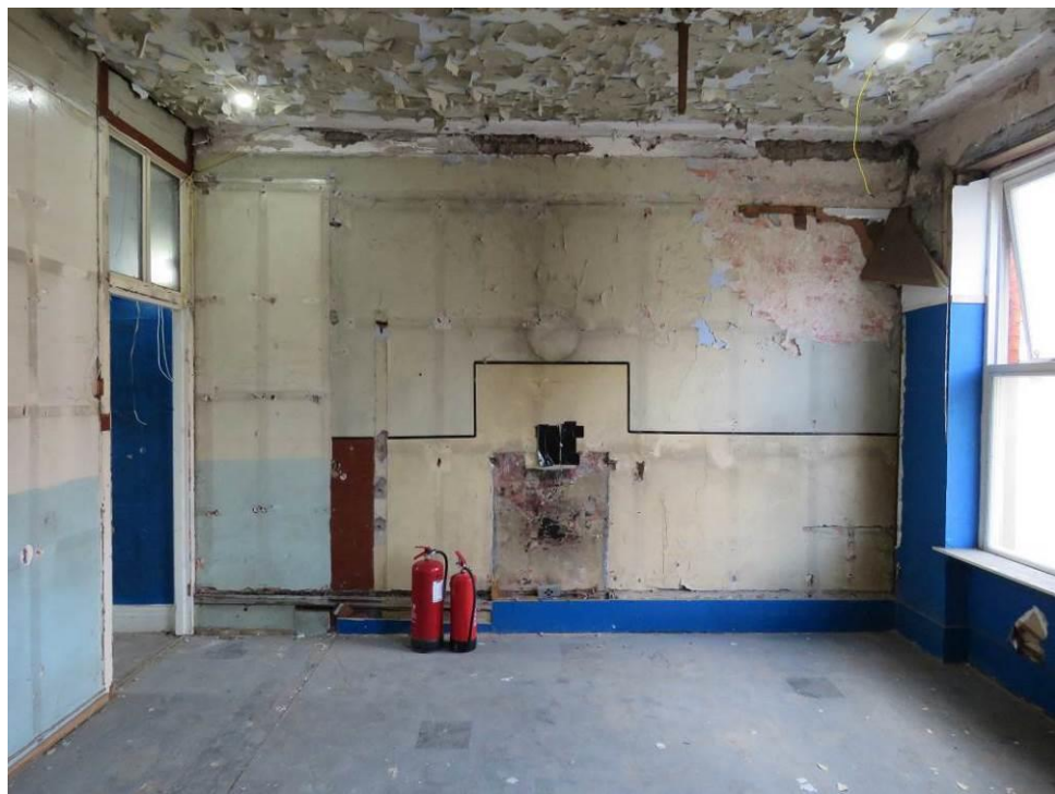
Figure 87 – Looking west into 1F12. The doorway leads into the staircase (1F18).
