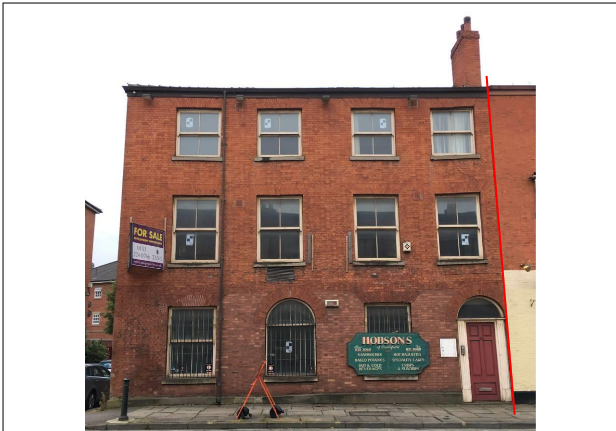
Figure 23 – The north (front) elevation of No. 123 Liverpool Road. Note the original entrance to No. 121 now forming a window to the left, and entrance to No. 123 to the right.
