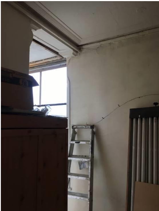
Figure 59 – Looking from the corridor into the inserted link corridor (1F07).
