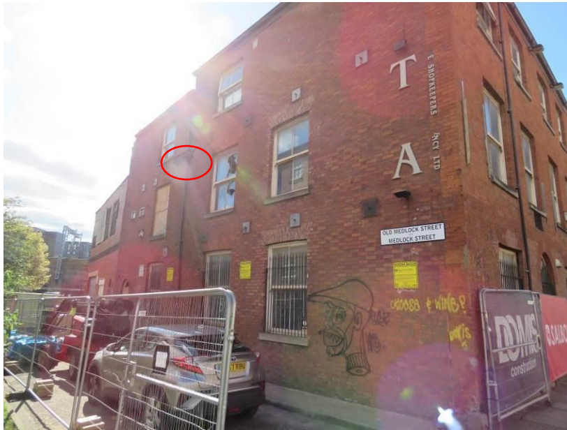
Figure 73 – Looking south along the east elevation, showing the recently completed emergency stabilisation works (circled).
