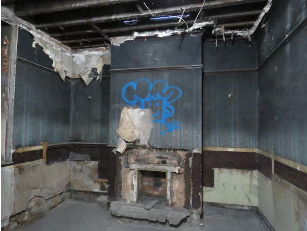
Figure 104 – Looking into the front bar room showing removed ceiling, cornice and timber fire surround (GF2).
