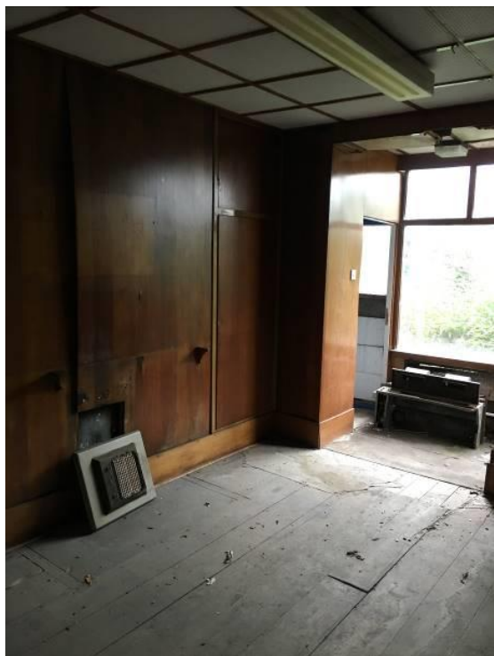
Figure 33 – The rear room on the first floor, showing the 1950s panelled interior and glazed extension (1F17).
