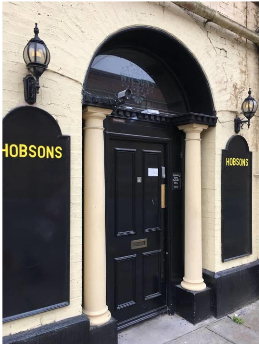
Figure 40 – The original entrance into the hotel, showing the partial survival of classical door case.
