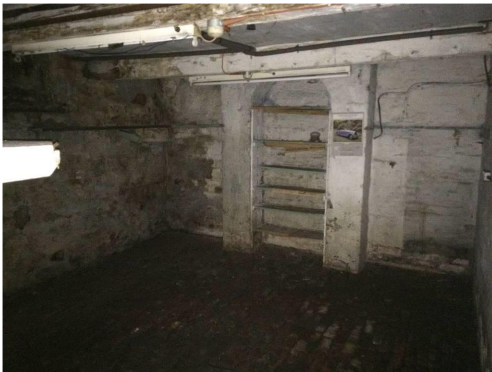
Figure 71 – The cellar room below the eastern bar room (GF2).
