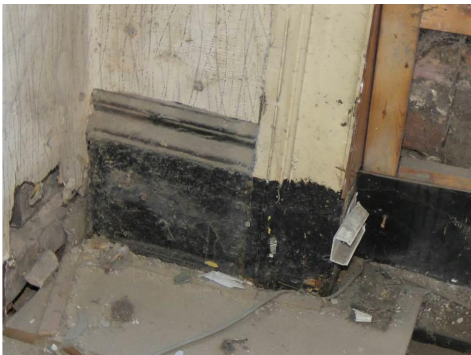
Figure 90 – A small example of surviving original timber skirting discovered adjacent to a window in 1F13.
