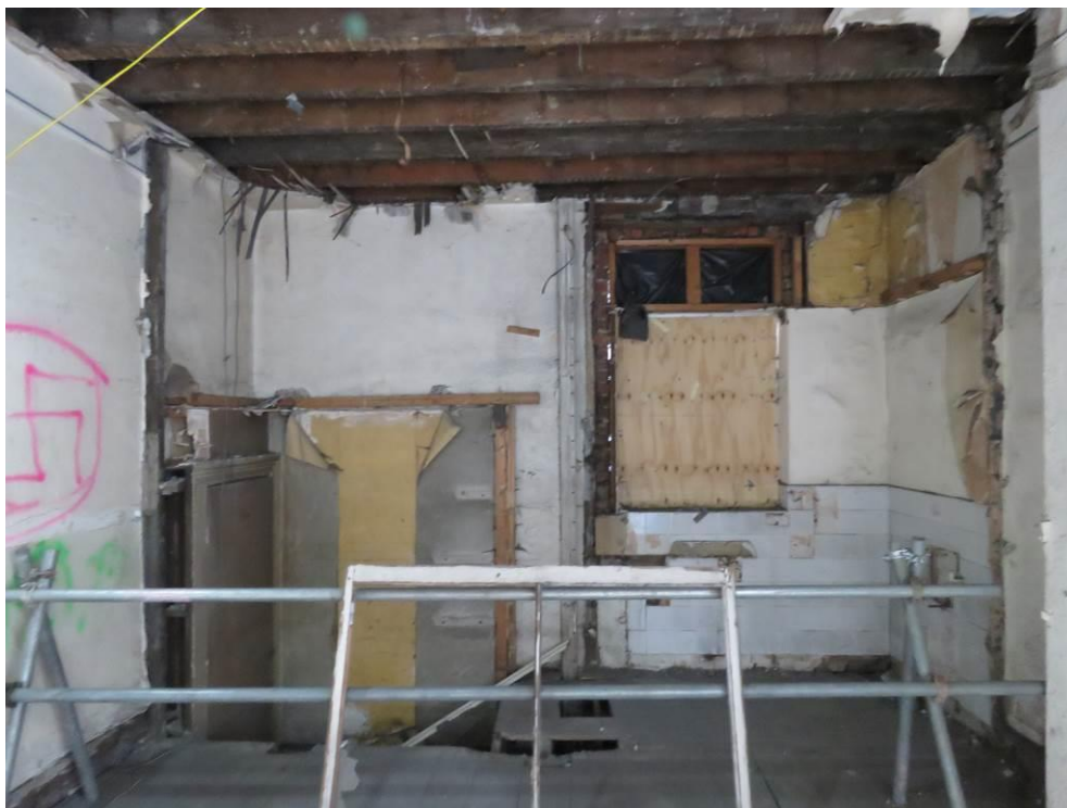
Figure 136 – Looking east across 1F06 towards the now removed partition enclosing the original link corridor. The extent of the former walk-in cupboard of 1F05 can now be seen to the left.
