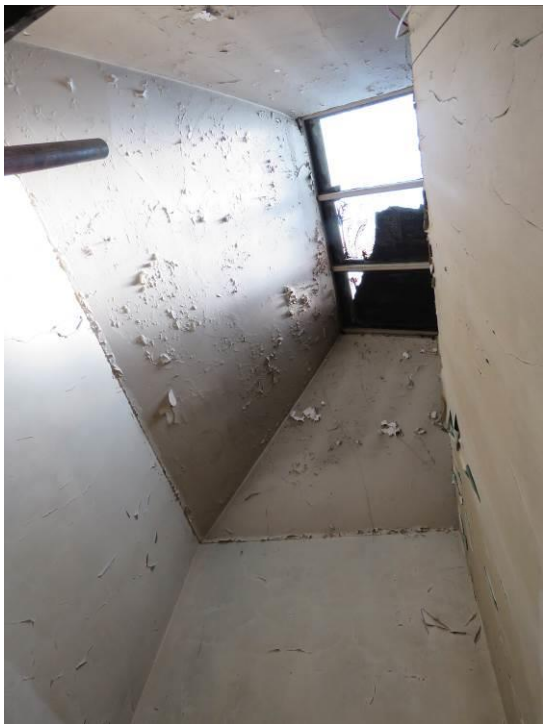
Figure 163 – The original rooflight to the head of the staircase (2F04).
