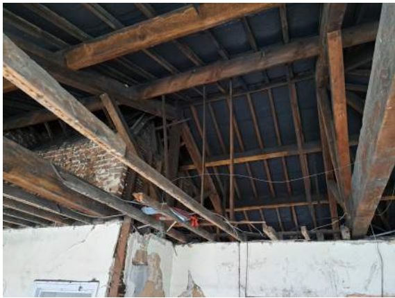
201: GENERAL VIEW OF ROOF TRUSSES OVER ORIGINAL PART OF 125 LIVERPOOL ROAD. THESE APPEAR TO BE IN GOOD CONDITION.
