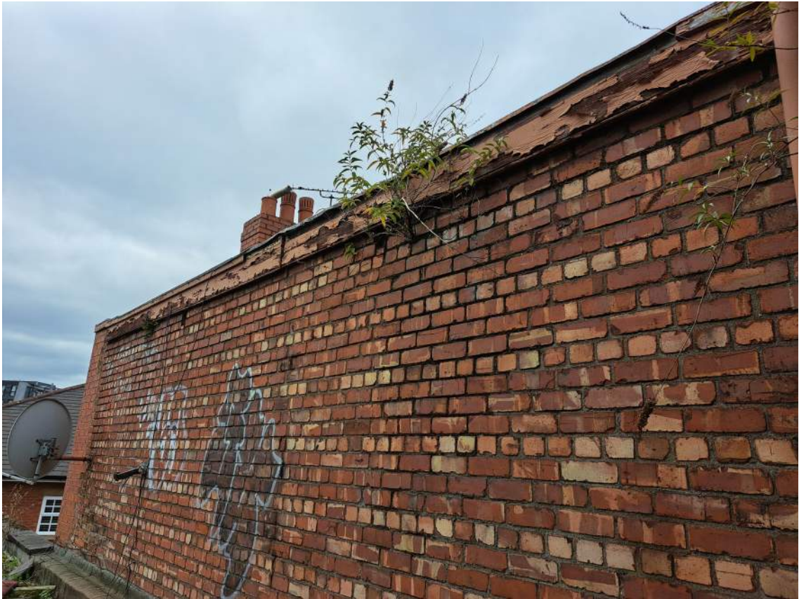
E04: MASONRY ON EAST ELEVATION TO 19TH CENTURY WOOLLAM PLACE EXTENSION SHOWS NO OBVIOUS DEFECTS. TIMBER FASCIA IN NEED OF REPLACEMENT. VEGETATION PRESENT AT EAVES LEVEL.
