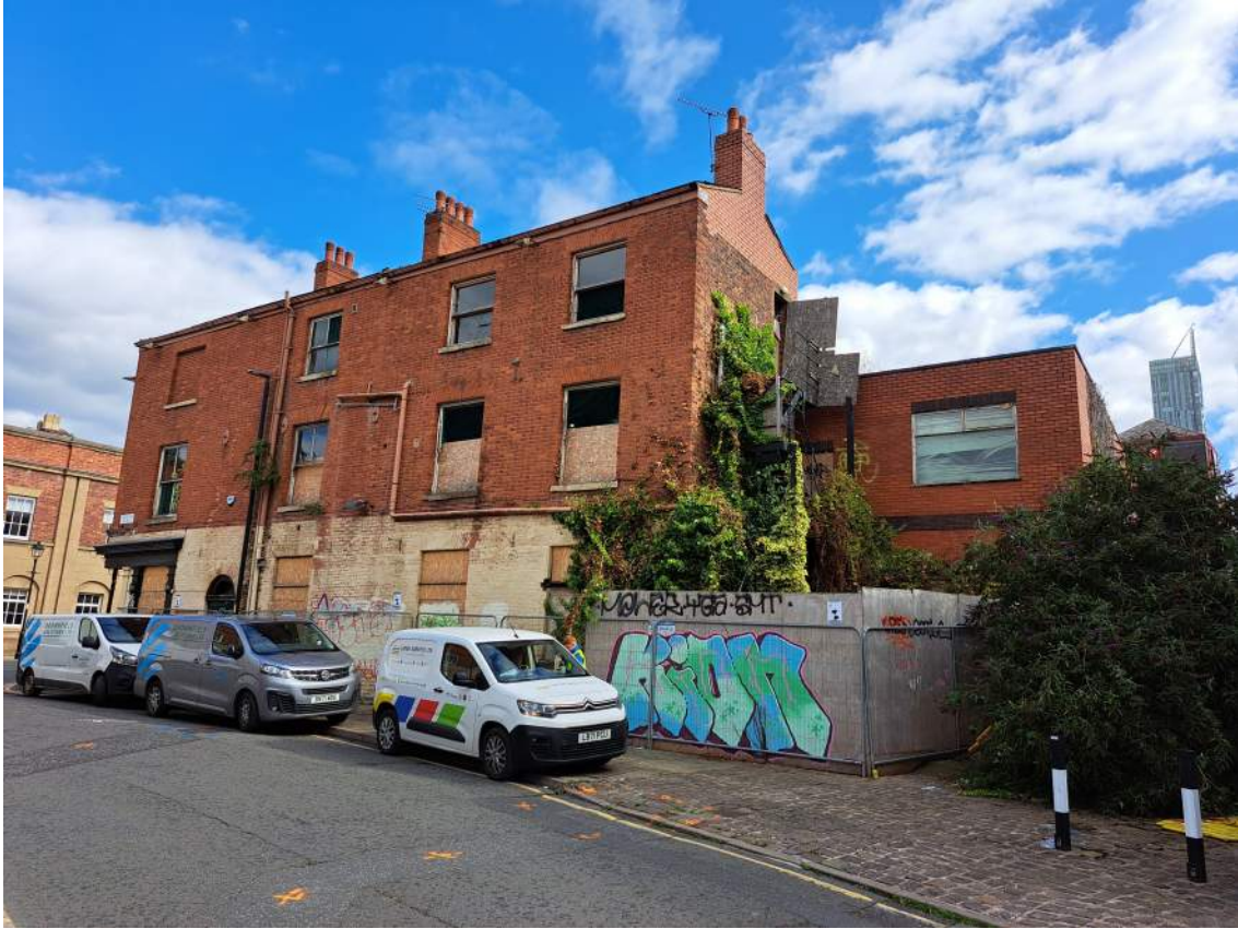
E16: GENERAL VIEW OF 125 LIVERPOOL ROAD FROM WOOLLAM PLACE.
