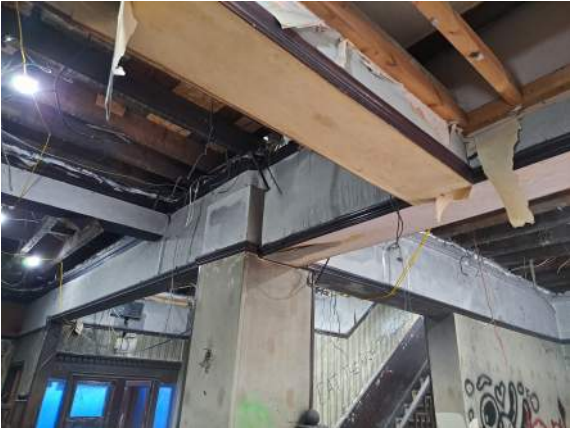
G04: DOWNSTAND BEAMS OVER ROOM G02. THESE HAVE LIKELY BEEN INTRODUCED TO ALLOW LOAD-BEARING WALLS TO BE REMOVED.
