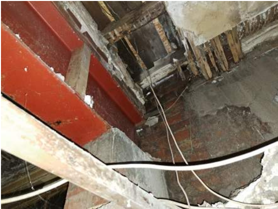
G03: STEEL BEAM BEARING ONTO MASONRY PIER BEHIND BAR IN ROOM G02.
