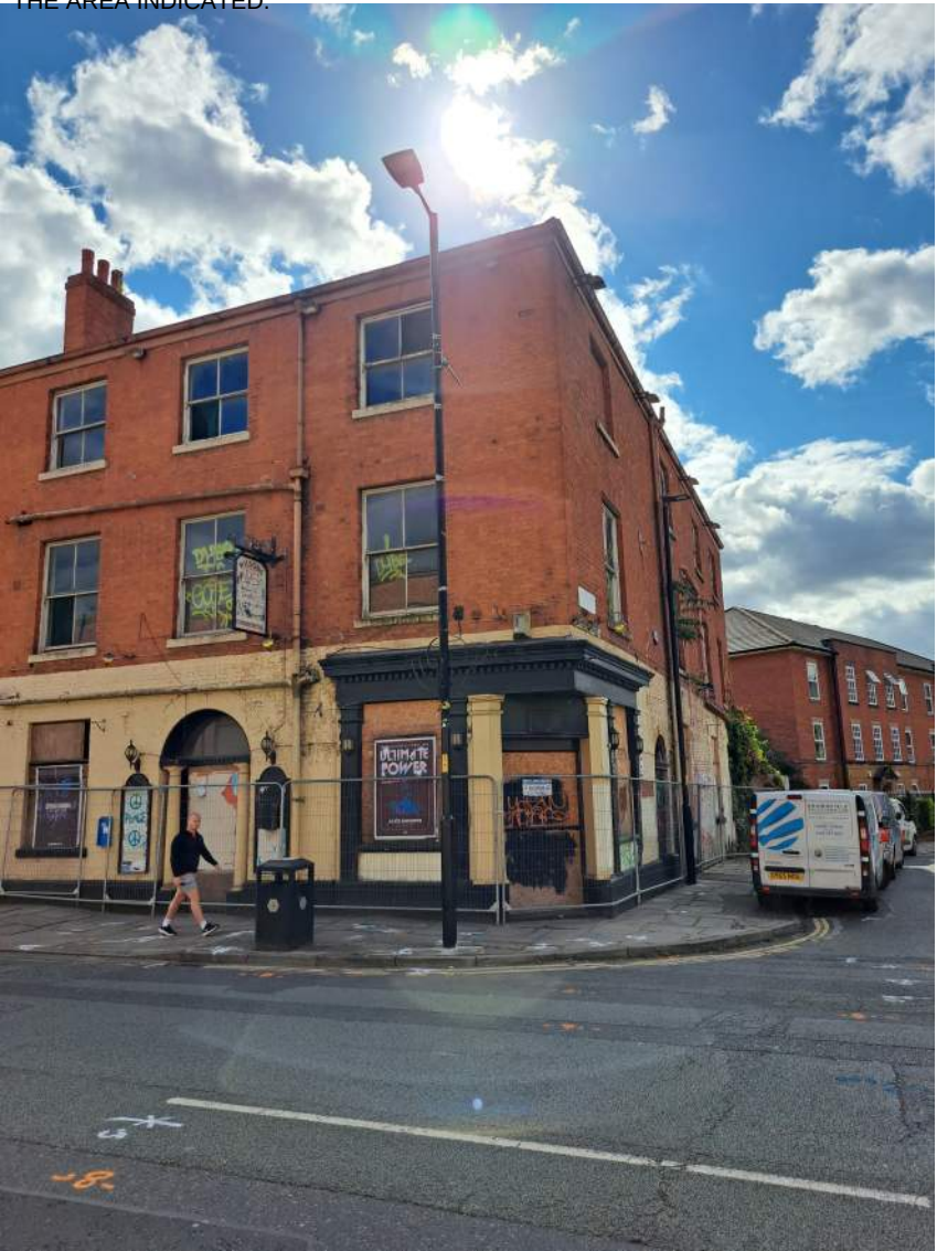
E12: GENERAL VIEW SHOWING THE RECESSED NORTH WEST CORNER AT GROUND FLOOR LEVEL OF 125 LIVERPOOL ROAD.
