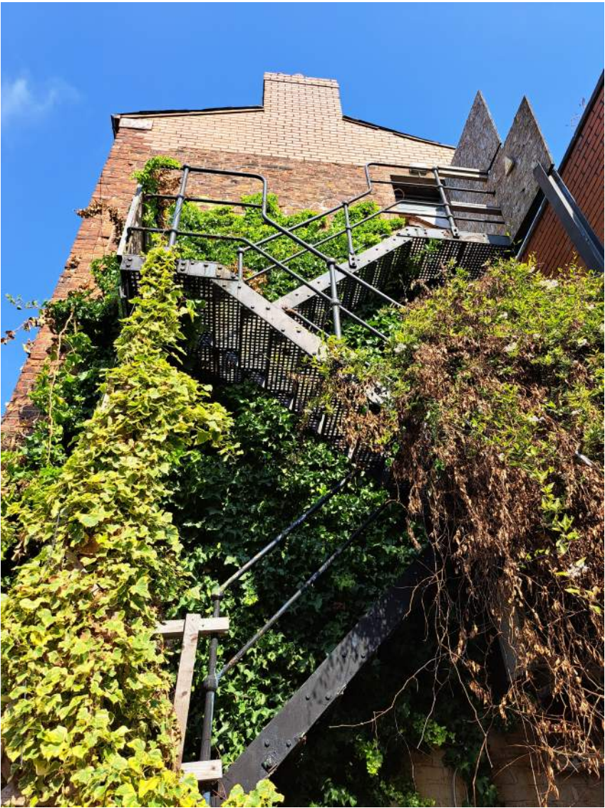
E15: VIEW OF SOUTH ELEVATION TO 19TH CENTURY WOOLLAM PLACE EXTENSION IS MAINLY OBSCURED DUE TO VEGETATION GROWTH. EVIDENCE OF RE-BUILDING ABOVE EAVES LEVEL. EXTERNAL FIRE ESCAPE APPEARS TO BE IN SERVICEABLE CONDITION.
