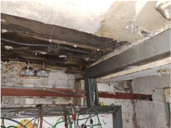
B08: REMEDIAL MASONRY PIER AT END OF TIMBER BEAM IN ROOM B08.
