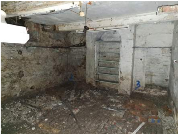
B03: GENERAL VIEW OF ROOM B02. THE BASEMENT FLOOR GENERALLY CONSISTS OF BRICK PAVING.
