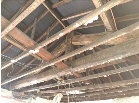
209: ROOF TRUSS OVER ROOM 206.
