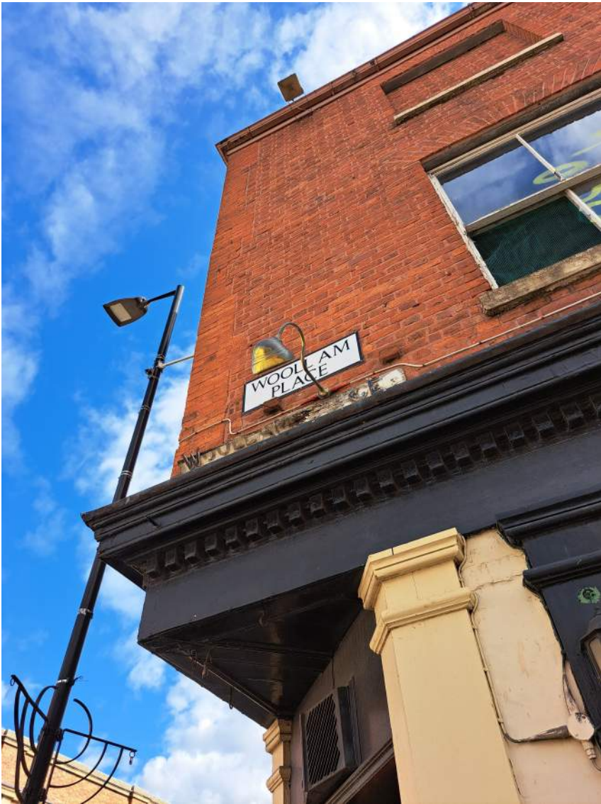
E13: PROJECTING CORNER ABOVE 1ST FLOOR ON THE NORTH WEST CORNER OF 125 LIVERPOOL ROAD. THERE ARE NO OBVIOUS SIGNS OF STRUCTURAL DISTRESS ABOVE.
