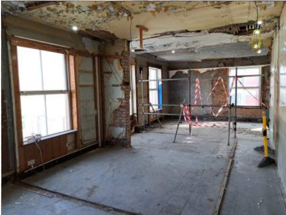
119: GENERAL VIEW OF ROOM 107.
