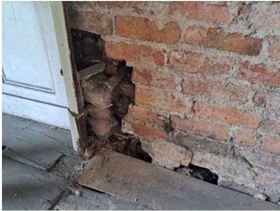
101: SECTION OF EXTERNAL WALL ON LIVERPOOL ROAD WITHIN ROOM 103 HAS BEEN OPENED UP TO ALLOW FOR SERVICE PENETRATIONS.
