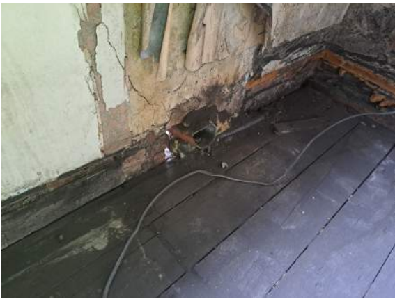
203: OPENING FORMED THROUGH EXTERNAL WALL ON LIVERPOOL ROAD IN ROOM 203 TO ALLOW FOR FOUL WATER PIPE.
