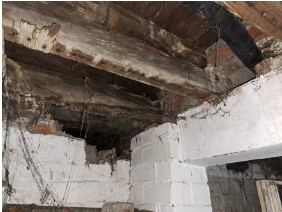
B06: MASONRY PIER PRESUMABLY ADDED AS REMEDIAL DETAIL TO ADDRESS LOSS OF TIMBER BEAM BEARING OVER ROOM B06. THIS WAS NOTED IN SEVERAL AREAS OF THE BASEMENT TO 125 LIVERPOOL ROAD.
