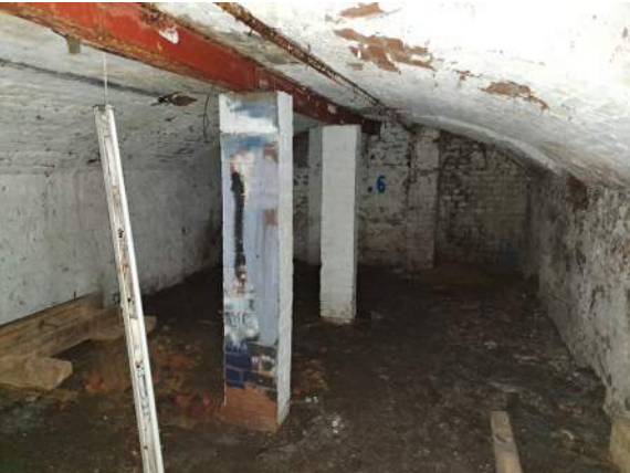
B09: REMEDIAL MASONRY PIERS AND STEEL BEAMS ADDED TO SUPPORT THE CROWN OF THE VAULTED CEILING IN ROOM B07.
