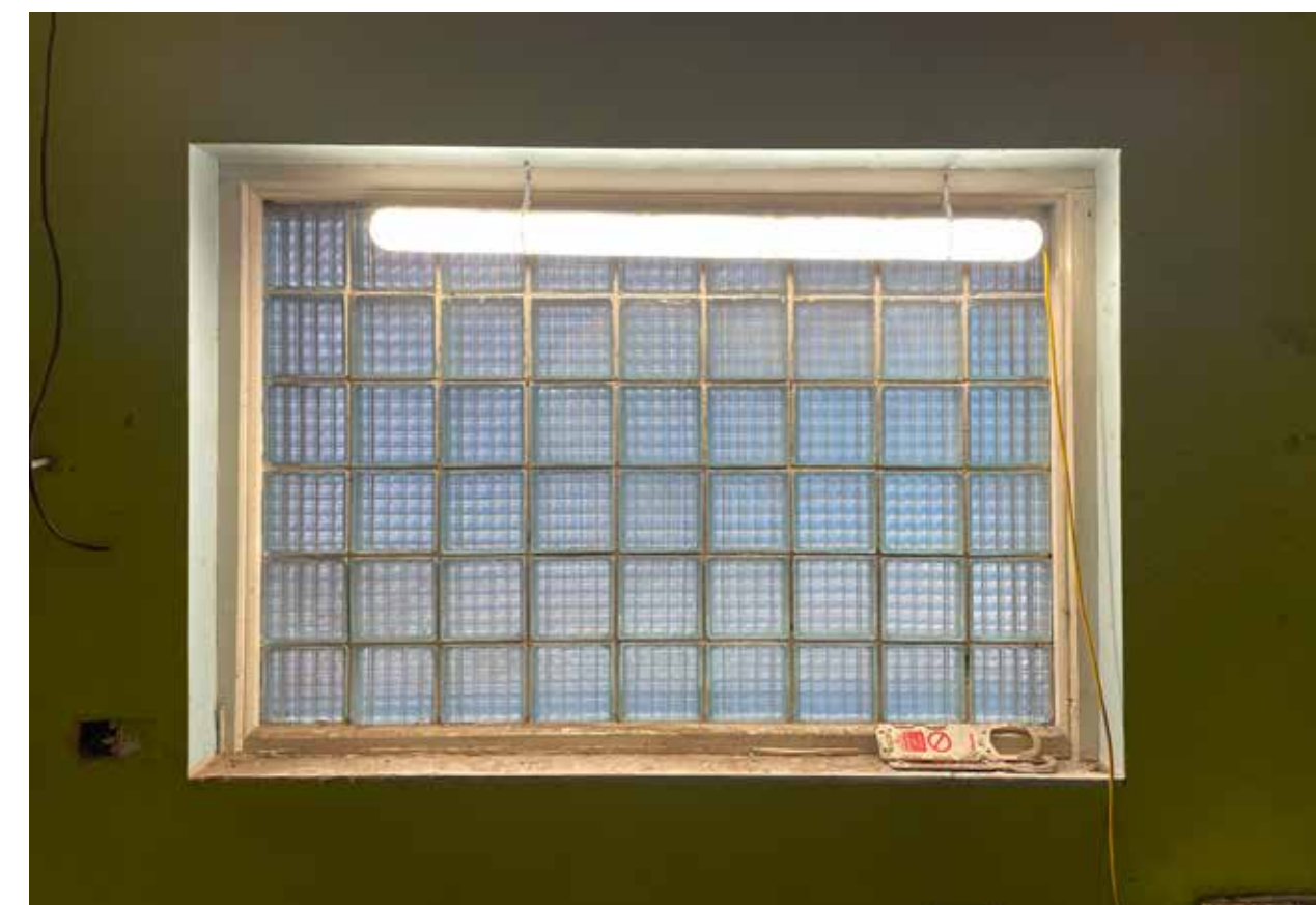
Image of later-inserted glass block window to Mangle Street facing end of building.
