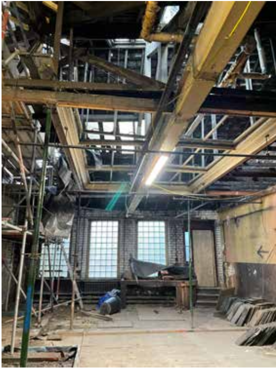
Image: Internal ceiling 10/12 following removal of lath and plaster.
