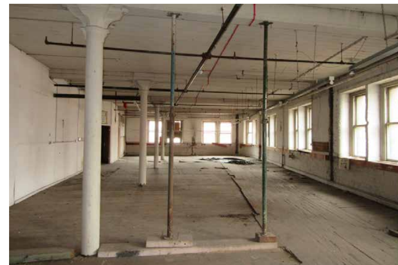
Image: Interior of first floor over Cottonopolis showing floor boards and columns.
