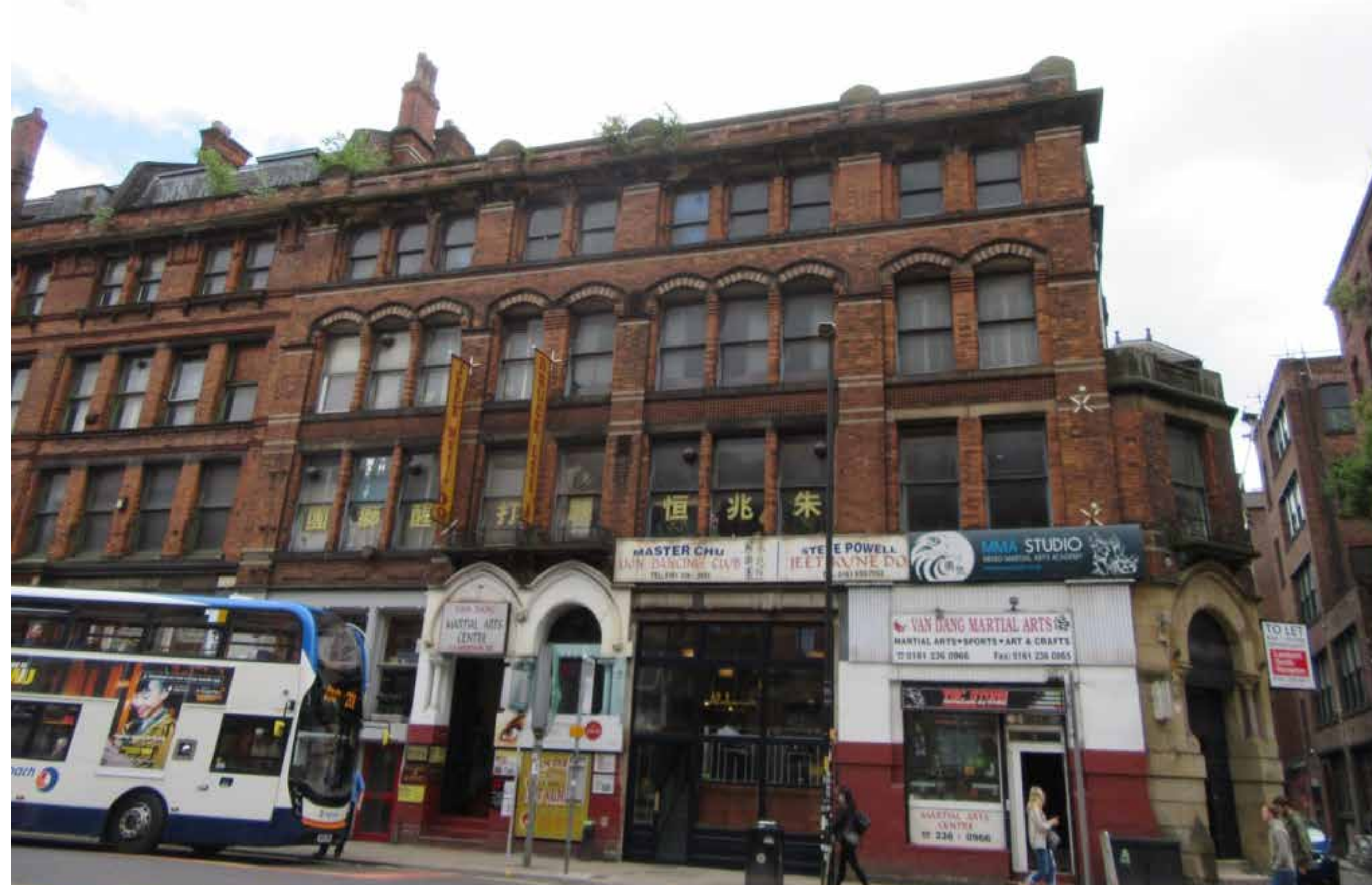
Image: Newton Street elevation, prior to start of works, 2017
