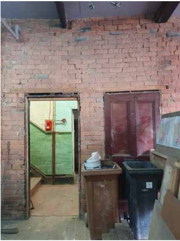
Images: Interior, ground floor at 12 Newton Street, showing small section of wall to be removed (between existing doors).
