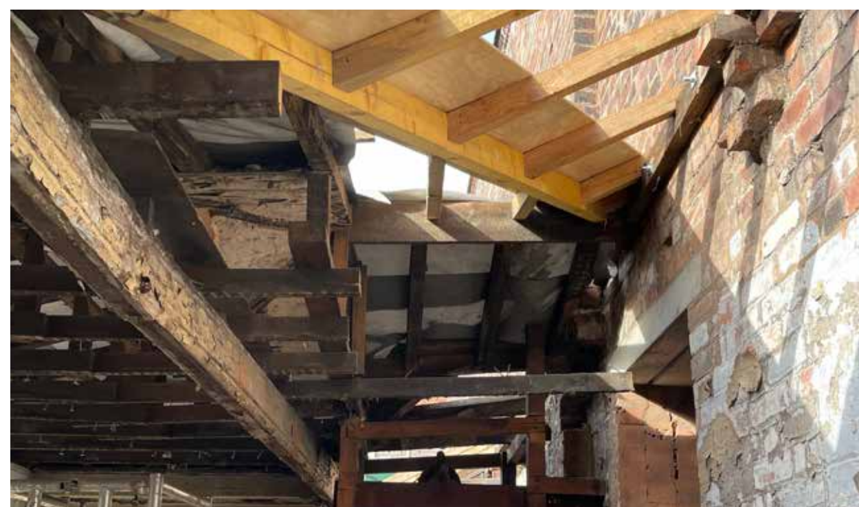
Images: Fourth floor internal space and mansard windows, hatches to roof, replacement dormer timbers.
