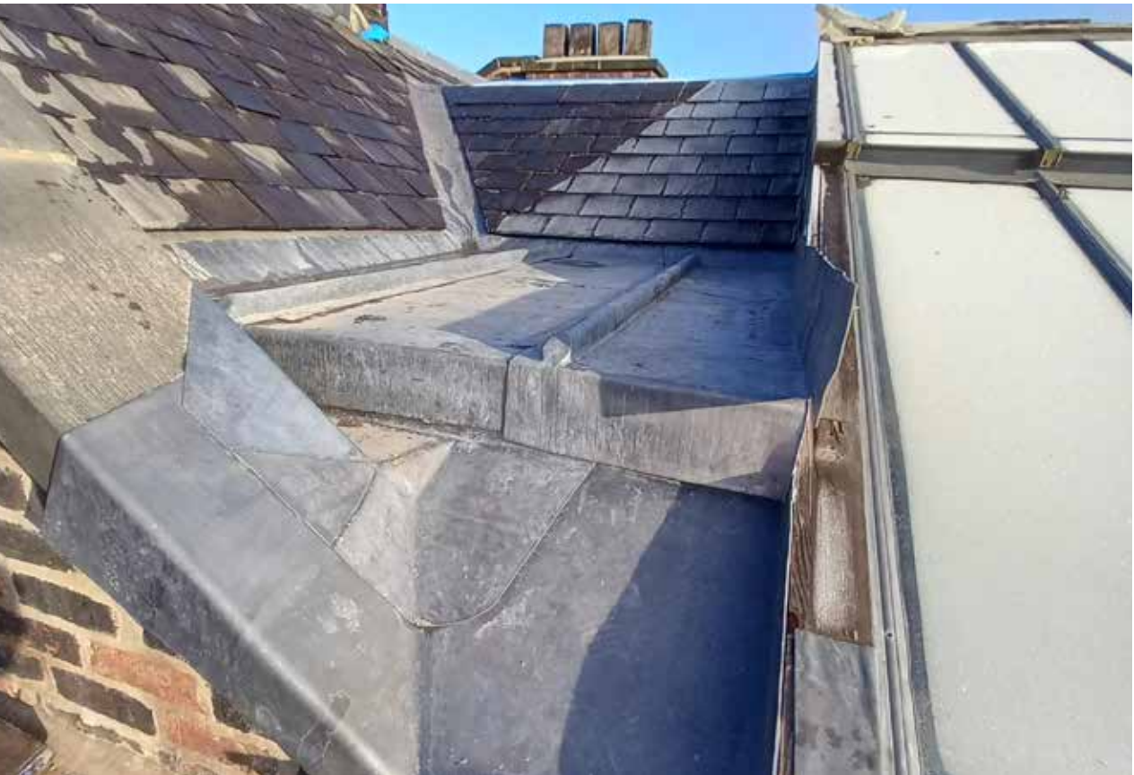
Image: Lift head to roof, with lead covering.
