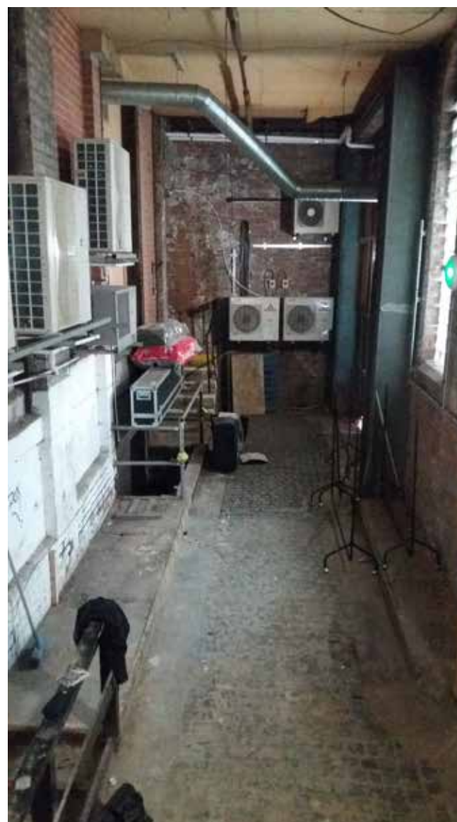
Image: Internal view of loading bay with staircases to left hand side.
