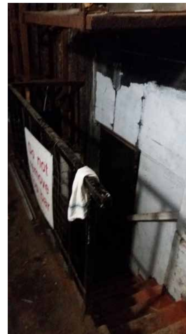
Image: Staircase connecting loading bay and basement
