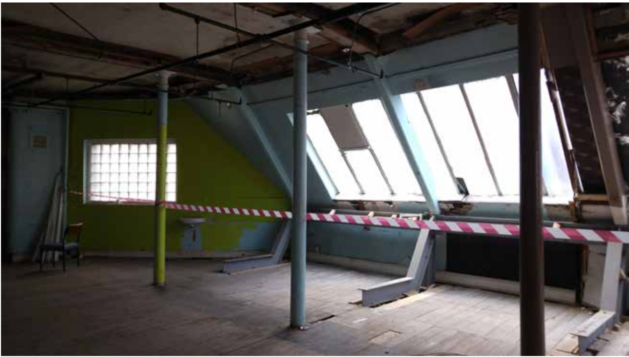
Image: Non-original glass block window, rooflights, columns and internal supports, first floor.
