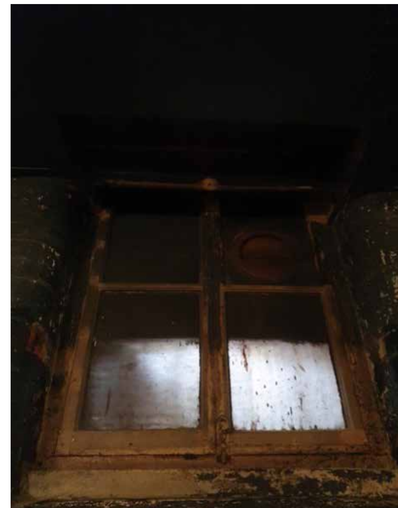
Image: Internal view of basement windows, Back Piccadilly.
