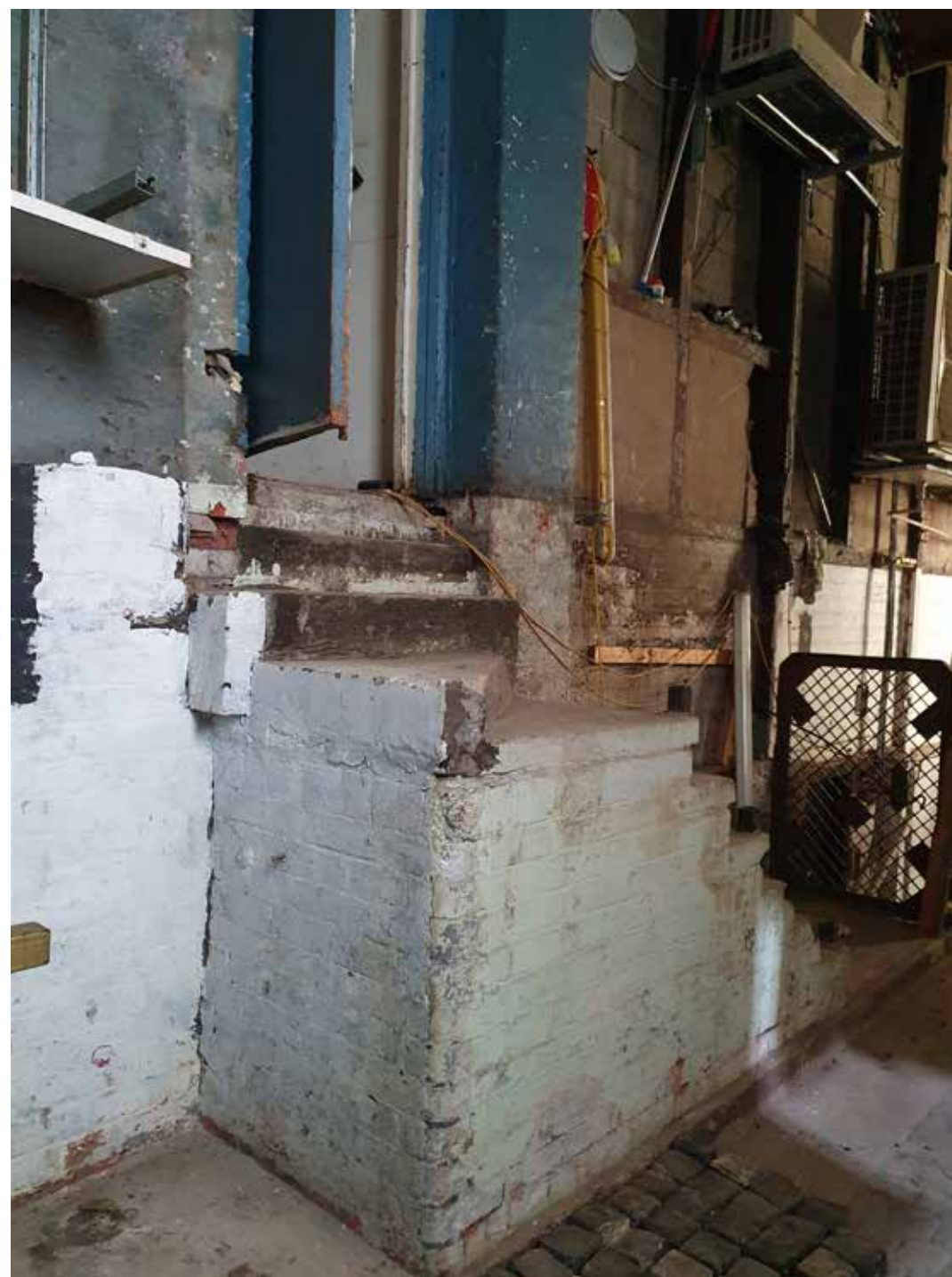
Image: Existing stairs (ST23) to loading bay, to be remodelled.
