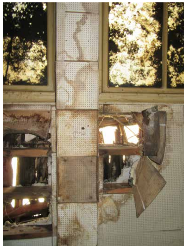
Image: Ceiling, now removed, third floor 10/12 Newton Street.
