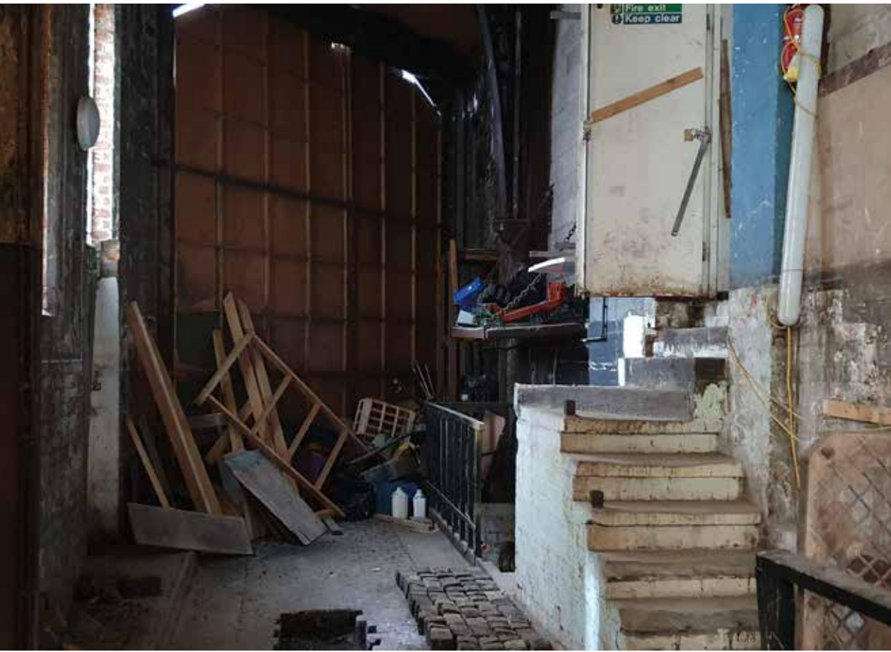
Image: ST23 to foreground and ST08 behind (to be glazed over).
