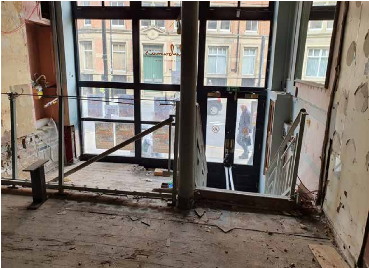
Image: Interior of number 10, showing floor and windows.
