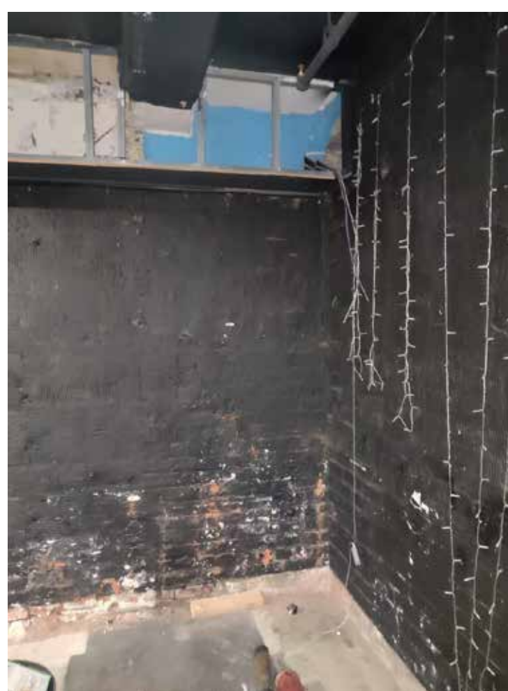
Image: Internal wall in basement, location of new doorway.
