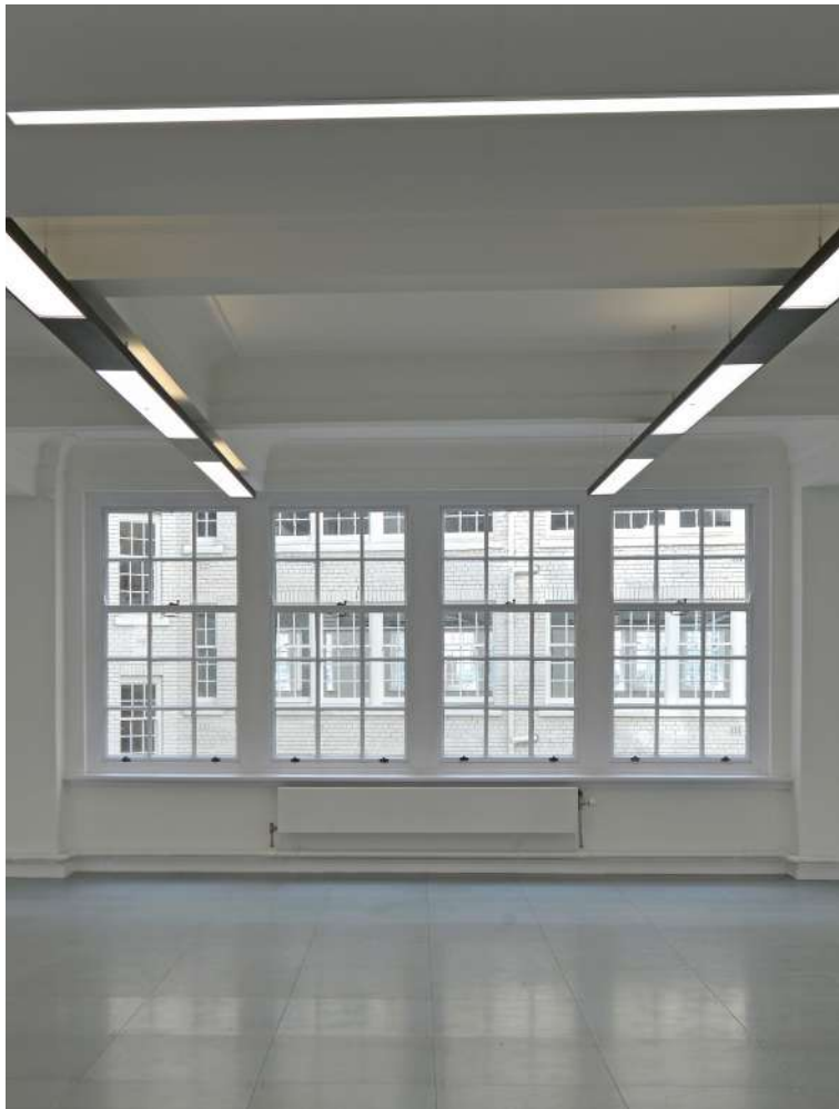
SASH WINDOWS TO LIGHTWELL AND OUTER FACADE
