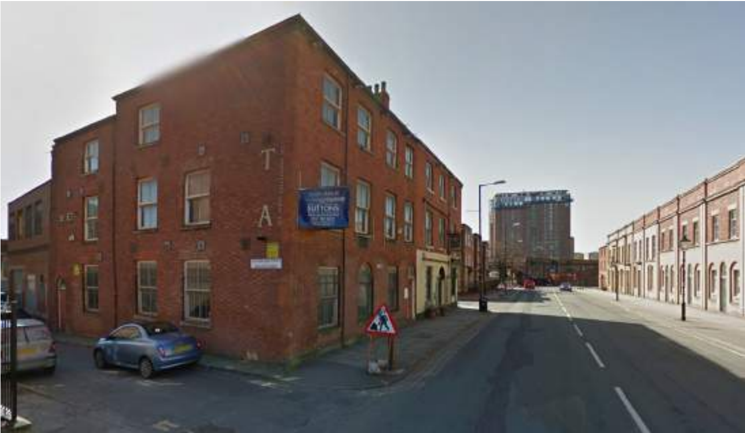
No. 123 from Liverpool Road/ Old Medlock Street.
