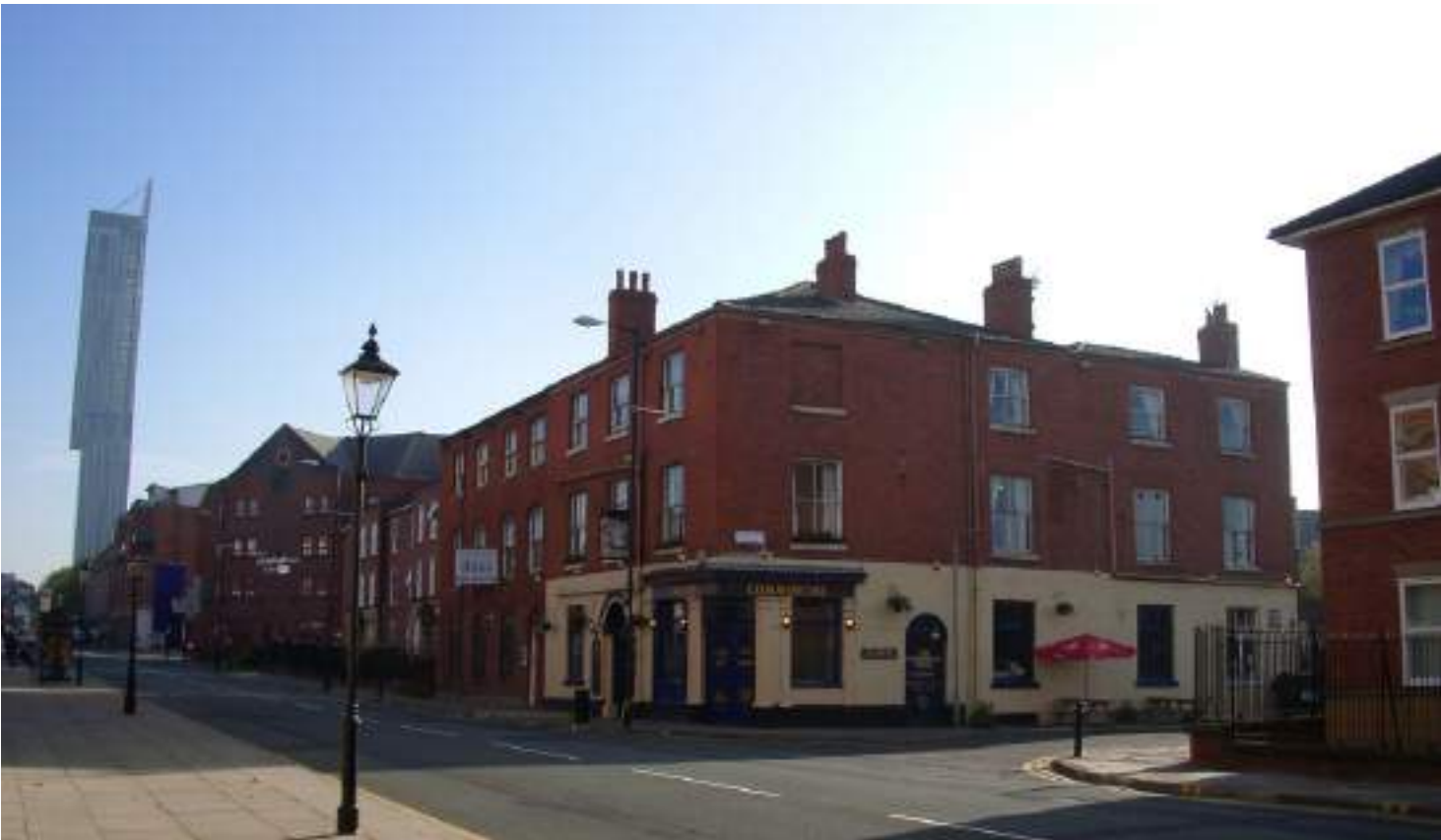
S02. No. 125 and 123. View from Liverpool Road
