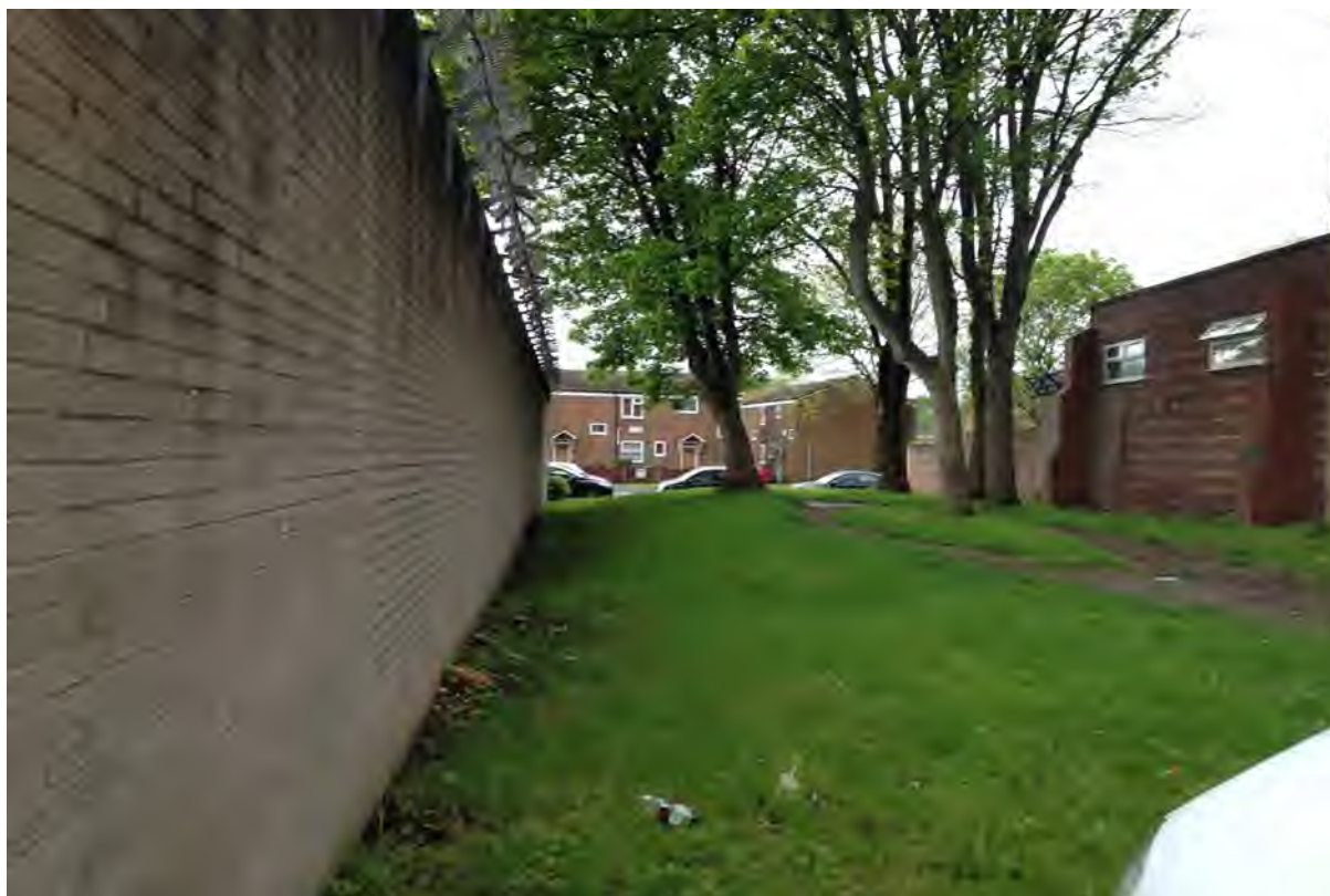
Plate 17 – Western Boundary Looking South
