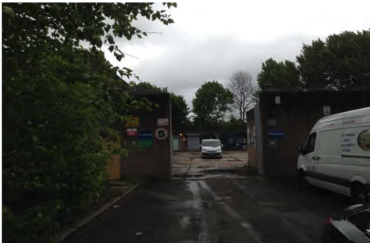
Plate 1 – Ripon Street Entrance Looking East
