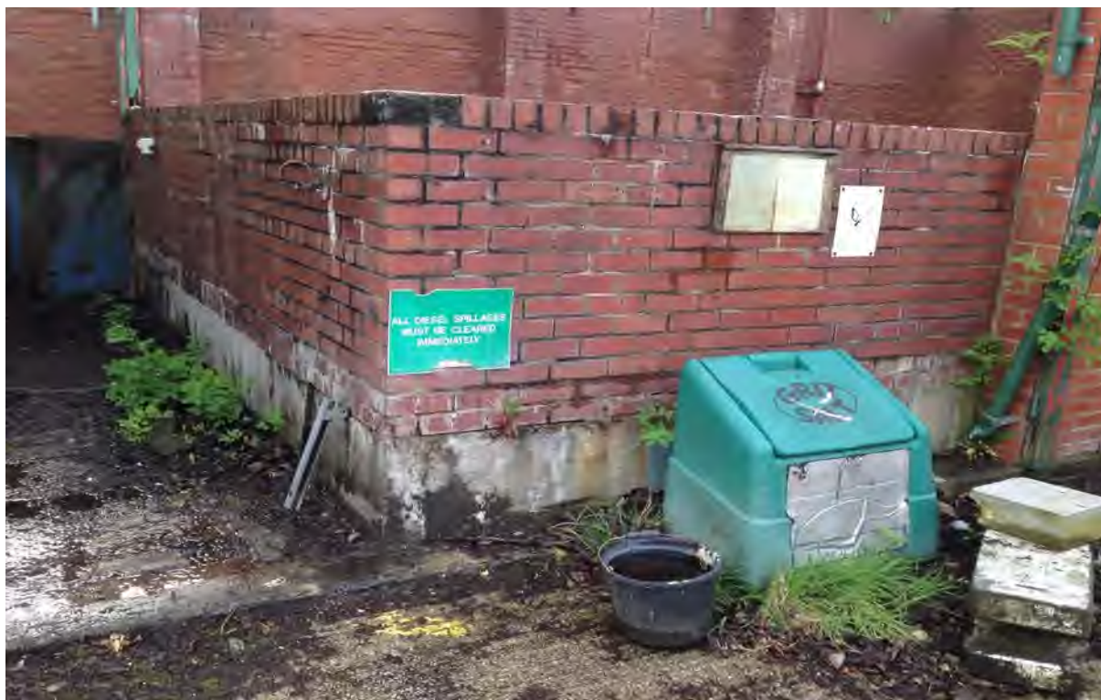
Plate 7 – Diesel Tank Bund in Southeastern Corner of Property
