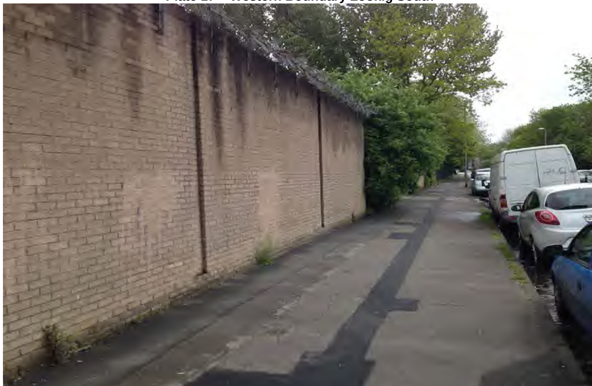
Plate 18 – Southern Boundary Looking East Along Denmark Road
